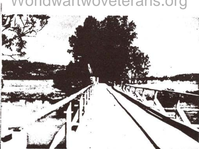
THE 111th ENGINEER BATTALION worked day and night to complete this timber trestle bridge across the Doubs in 22 hours. Then tanks and infantry poured across to continue the chase (below).
