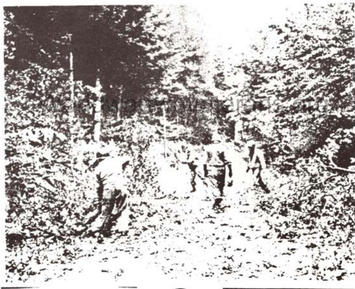
CANT HOOKS are used to roll logs off to the side of the road. (Below) ENGINEERS clear remaining brush.
