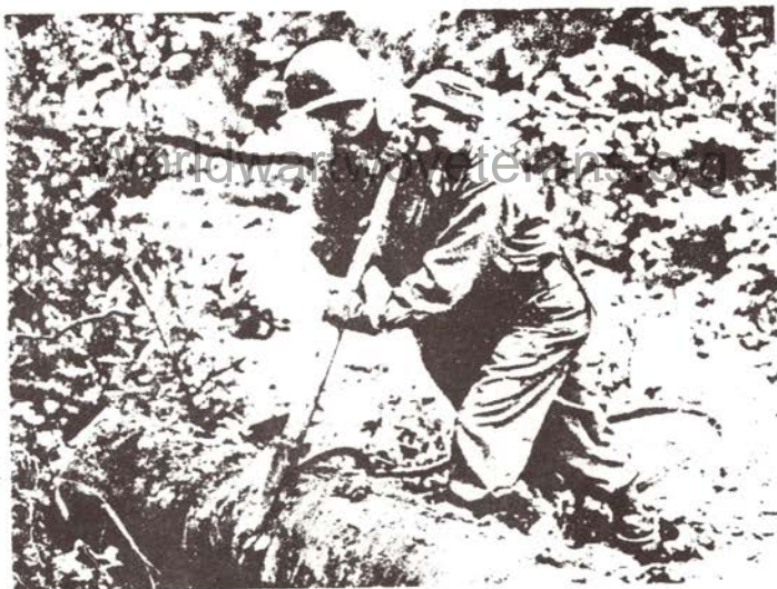
CANT HOOKS are used to roll logs off to the side of the road. (Below) ENGINEERS clear remaining brush.
