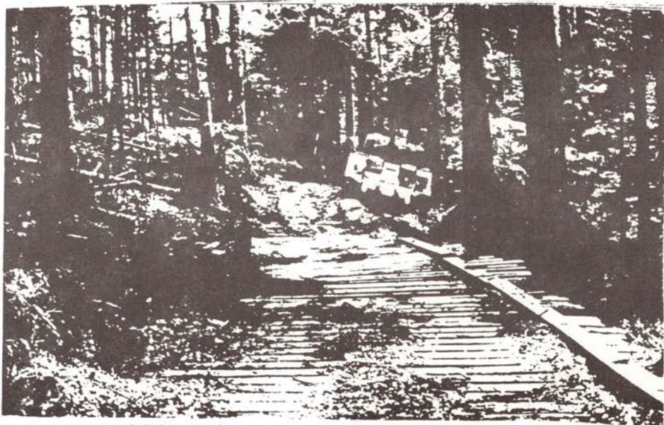
ENGINEERS CONSTRUCTED A PLANK FLOOR OVER SECTIONS OF SEVEN AND ONE-HALF MILE ROAD TO "LOST BATTALION."
