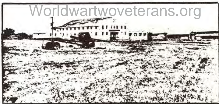
Here's old Headquarters Area, north part of the Camp Bowie area, going east to warehouse area, as it looks today. Lot's of memories.
