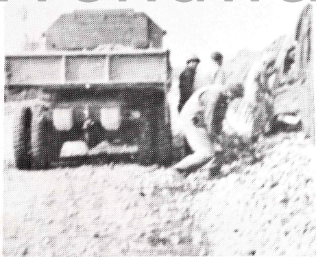
Here's some Co. C, 111th Engineers loading railroad ballast to build a road to the ill-fated Rapido River crossing in Jan. 1944, sent in by Oscar Troehler, Circleville, OH.
