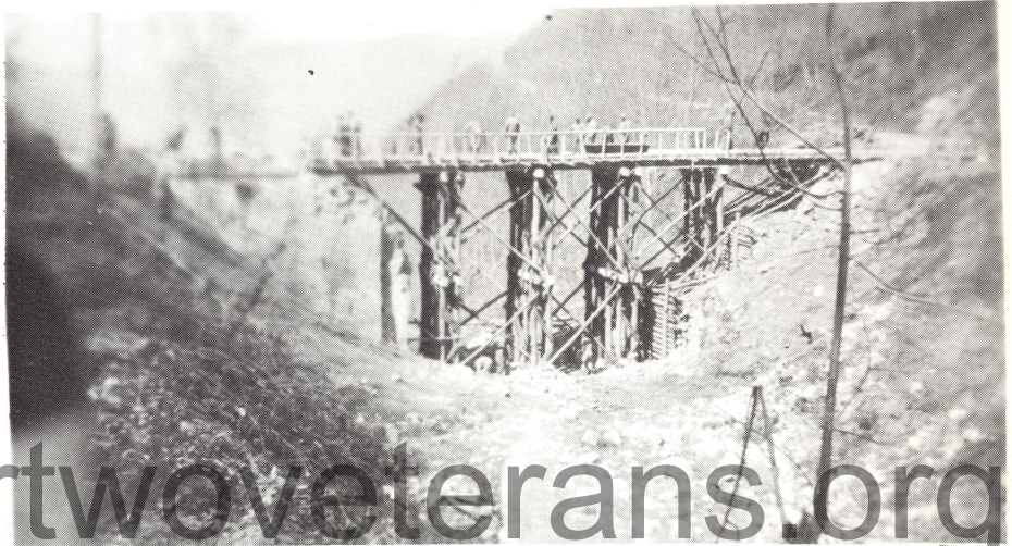
If you haven't got the proper materials, you gotta improvise. Here's a timber trestle bridge in the mountains of Italy constructed entirely of native materials by the ingenious 111th Engineer Battalion. Col. Stoval knew his men 'wood' do it. (Thanks for this pix, Col.)
