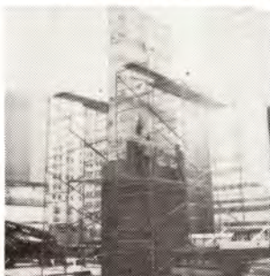
Monument during removal
