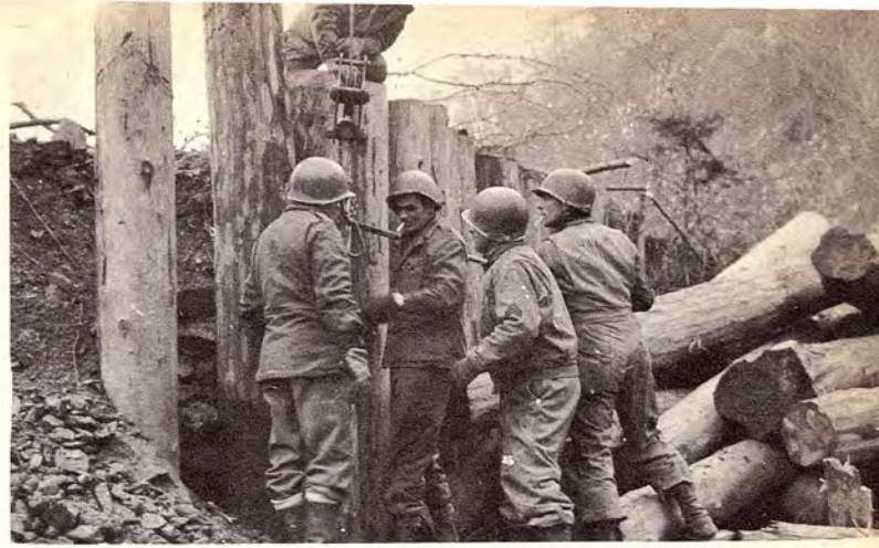
MEN OF THE 111th ENGINEERS removing one of the many roadblocks that slowed the drive into the Rhine Valley.
