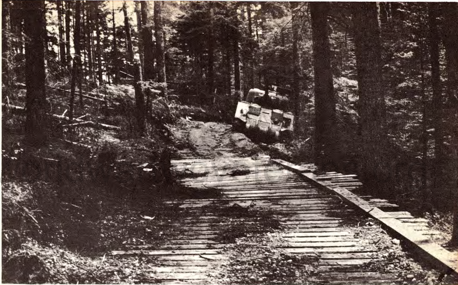
ENGINEERS CONSTRUCTED A PLANK FLOOR OVER SECTIONS OF SEVEN-AND-ONE-HALF MILE ROAD TO "LOST BATTALION."
