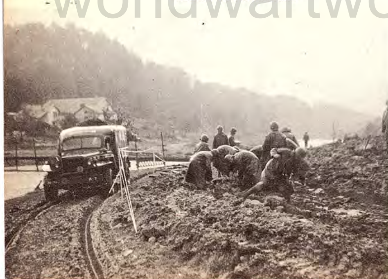
HEAVY RAINS KEPT ENGINEERS BUSY ON THE BRIDGE APPROACHES.
