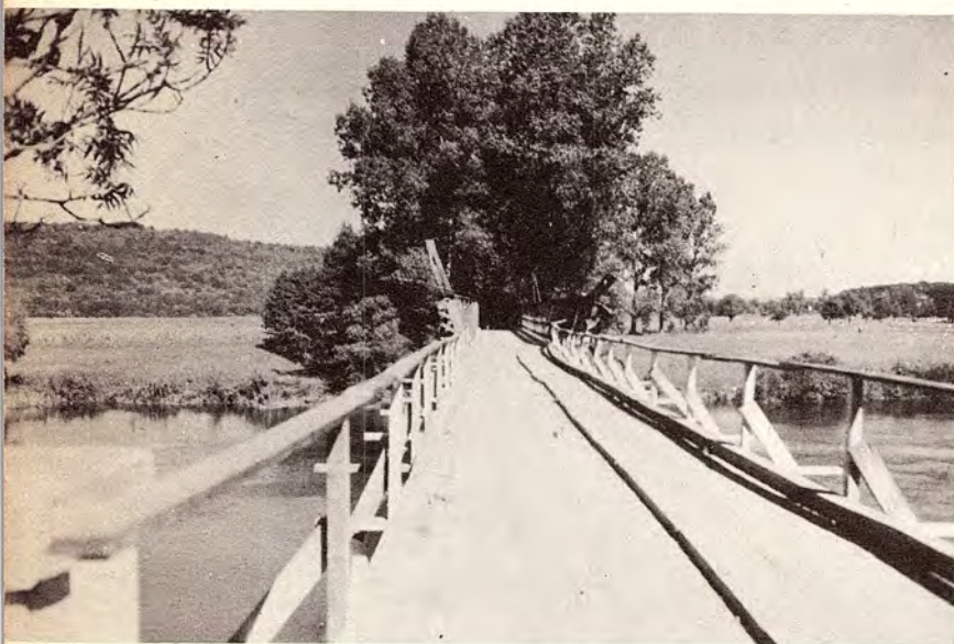
THE 111th ENGINEER BATTALION worked day and night to complete this timber trestle bridge across the Doubs in 22 hours. Then tanks and infantry poured across to continue the chase (below).
