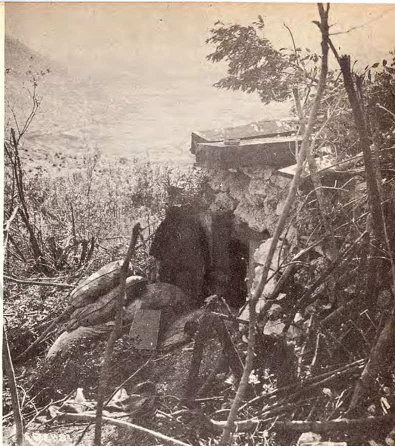
RAILROAD TIES , telephone poles, local stones and sandbags went into the construction of German shelters on Mt. Lungo. These enabled the enemy to withstand heavy artillery bombardments.
