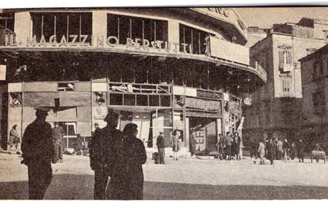
ONE OF THE MOST FREQUENTED spots on the Via Roma is the Galleria Umberto. In the interior are the more exclusive jewelry, painting, and wine shops. Bombing severely damaged the Galleria's glass dome. above. Naples street scene shows some modern shops.
