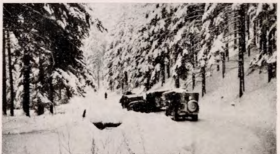
MAINTENANCE CREW AT WORK IN VOSGES
