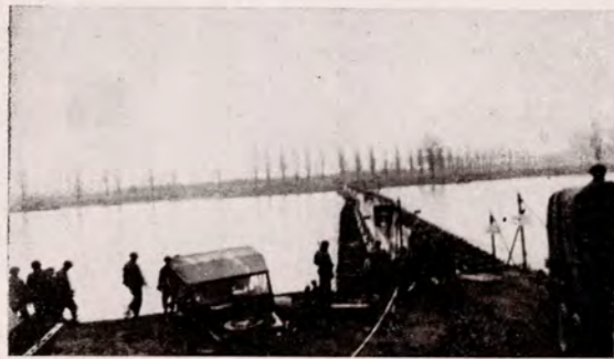
PONTOON BRIDGE ACROSS RHINE
