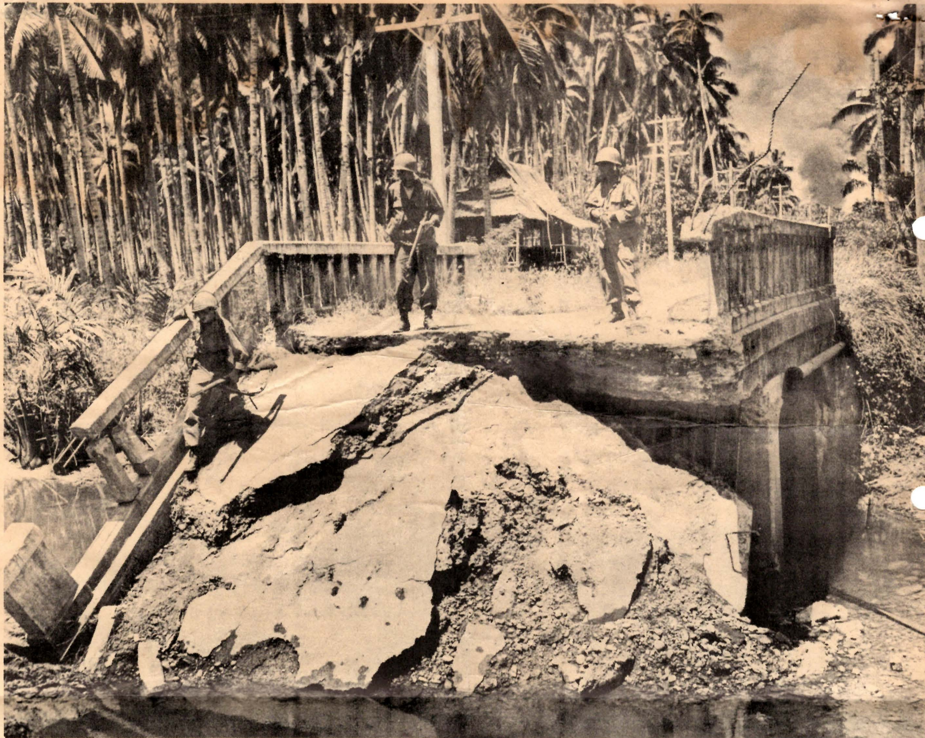
EFFORT WASTED---It takes more than a destroyed bridge to halt the advance of Yanks on Mindanao Island, Philippines. Here, Infantrymen cross a ruined bridge south of the city of San Jose. Smoke in the background pours from oil and gas dumps which were set ablaze by Jap artillery. (U.S. Army Signal Corps Photo, reproduced and distributed by Information Branch, I-E Section, CPBC).
