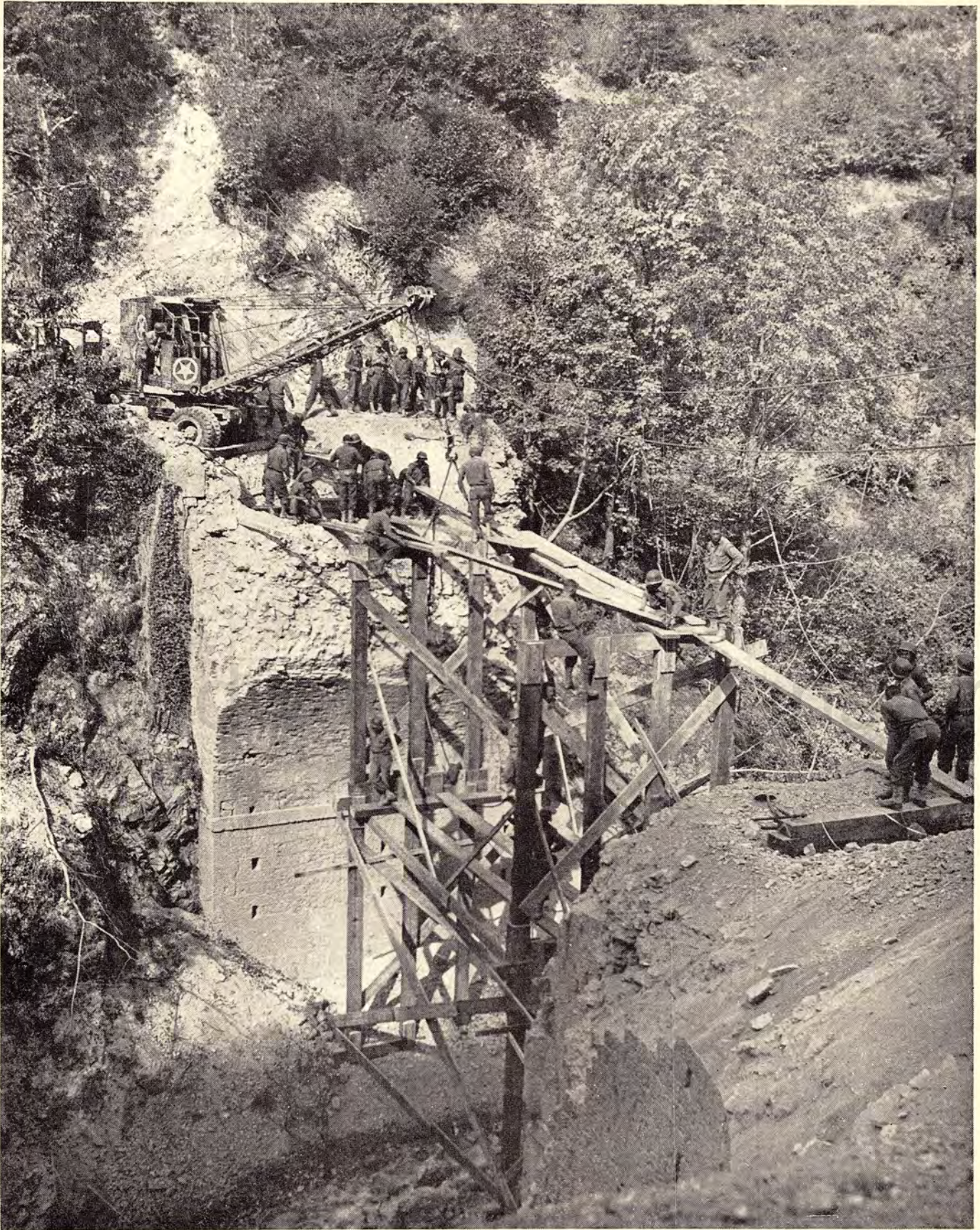
3d Division's 10th Engineers reconstruct a demolished bridge near Salitto, Italy.
