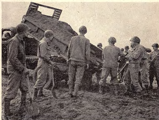
The 10th Engineers construct a road through the Division's bivouac area in the forest.
