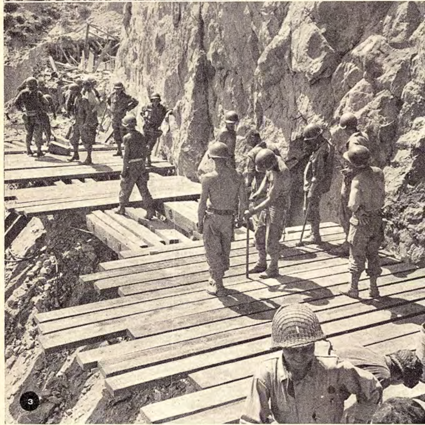
The 3d Division's 10th Engineers "hang a bridge from the sky" at Cape Calava. (1) an engineer drills into the rock with a jackhammer. (2) a heavy timber is wrestled into position. (3) the flooring is laid. (4) General Truscott is the first to cross the span.
