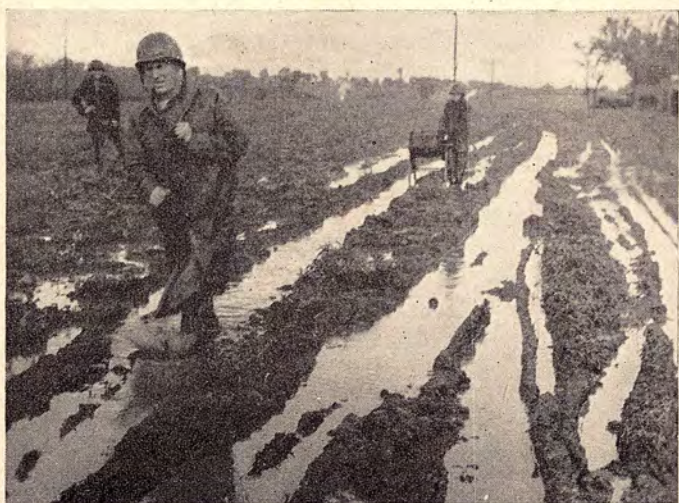
Wiremen of the 3d Signal Company lay wire in the Italian mud.
