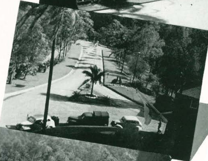
Below: Main Road showing Hairpin Turn.
