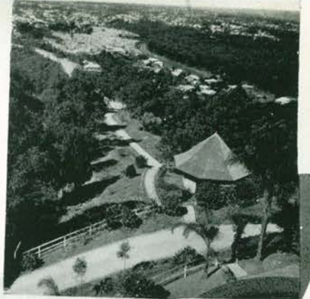
Summer House and footpath leading to Hospital.
