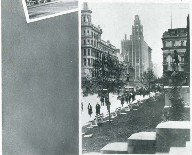
Collins Street, looking West.
