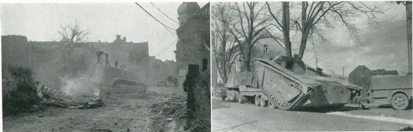
Many routes had to be widened and cleared of debris for the passage of the heavy vehicles transporting equipment to the west bank of the Rhine River for the crossing operation. At left, a bulldozer clears a route through Alpen, Germany. At right, Alligators are being unloaded in the vicinity of Rheinberg, Germany.
