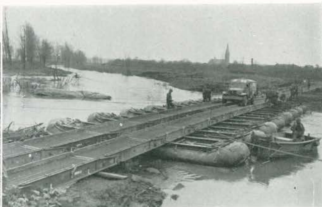
By 27 February, troops and equipment were moving across the Roer River in a steady stream. At left, elements of the 35th Infantry Division approach crossing sites near Hilfarth to cross the completed treadway bridge shown at right.
