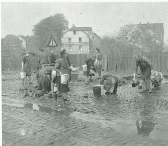
An acute water shortage existed in many of the cities of the Ruhr industrial area. Here, citizens of Witten, Germany, scoop water out of the street adjacent to a broken water main. Appropriate notices were posted to warn these people of the dangers arising from such practices, and action was taken to restore water service as soon as possible.
