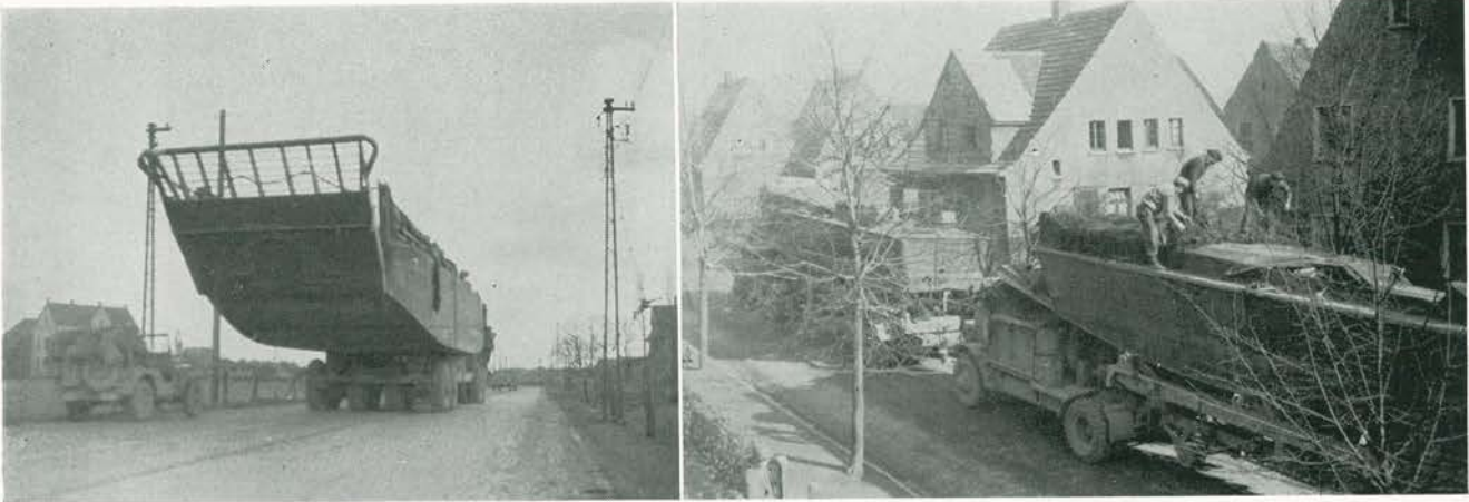
Giant trucking operations were under way in the XVI Corps sector just prior to the river-crossing operation, as heavy Ordnance vehicles moved up road- and bridge-building materials, storm and assault boats, and landing craft. At left, landing craft that had been set ashore at LeHavre, France, are trucked forward to the vicinity of Lintfort, Germany.
