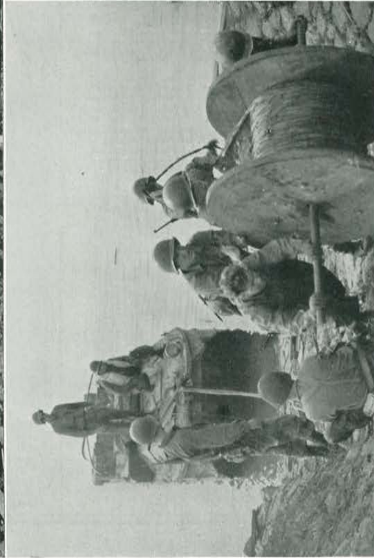
At upper left, a 97th Signal Battalion sign painter gets an OK from his first sergeant marking the location of communications cable across the Rhine River from Borth, Germany. At upper right, a Signal Battalion cableman identifies pairs on a German underground cable used to carry telephone conversations on the XVI Corps front near Borth, Germany. At lower left, linemen roll a reel of submarine cable ashore on the east bank of the Rhine River after the cable had been laid across the river by means of the amphibious vehicle in the background. At lower right, spiral-four cable, commonly used throughout all XVI Corps operations for wire communications, is buried with a cable plow as wire communications men of a signal battalion run lines up to forward positions near Rheimberg. Cable was buried to provide greatest possible protection from interruptions during combat. The continuous painstaking efforts of the Corps signal battalion in providing efficient and uninterrupted communications service throughout the Corps contributed immeasurably to its success.
