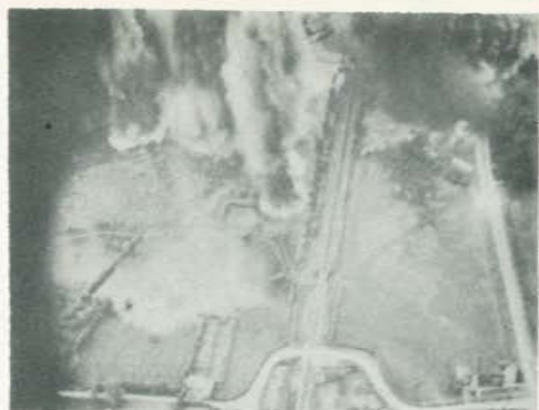
LESSAY RAIL & HWAY FACILITIES
