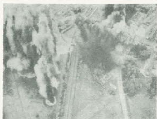
LESSAY RAIL & HWAY FACILITIES
