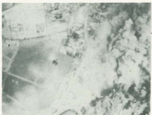
CARENTAN RAIL FACILITIES
