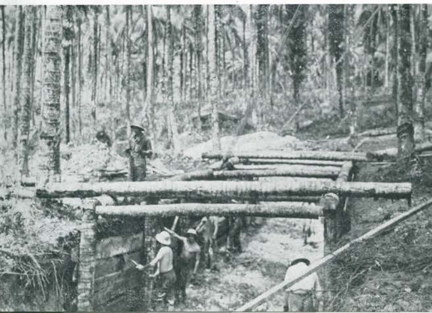
Framing underground surgery
