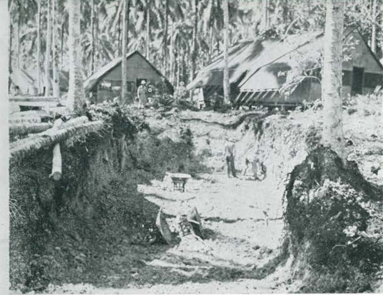
Excavation for underground surgery
