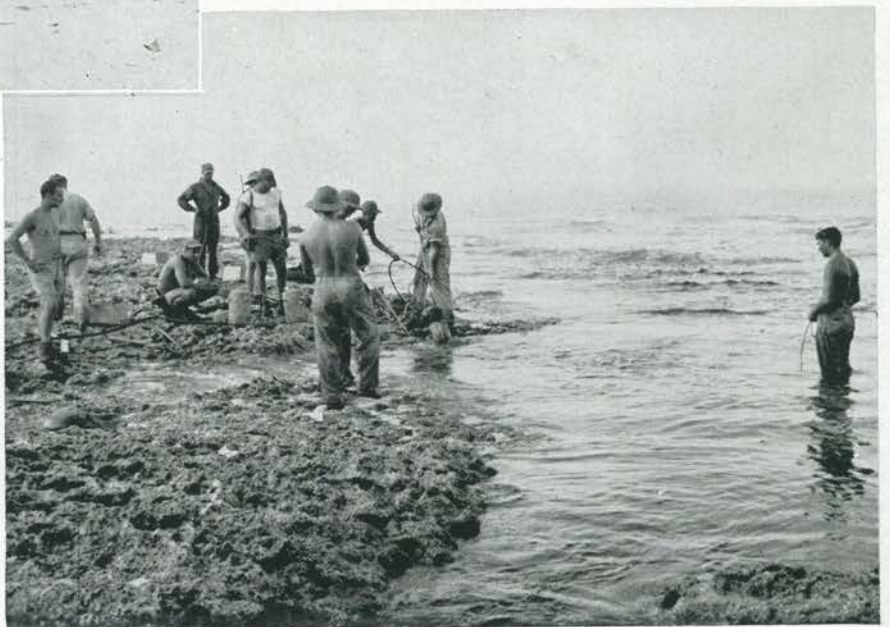
Setting Dynamite Under Water-Pilots' Pool
