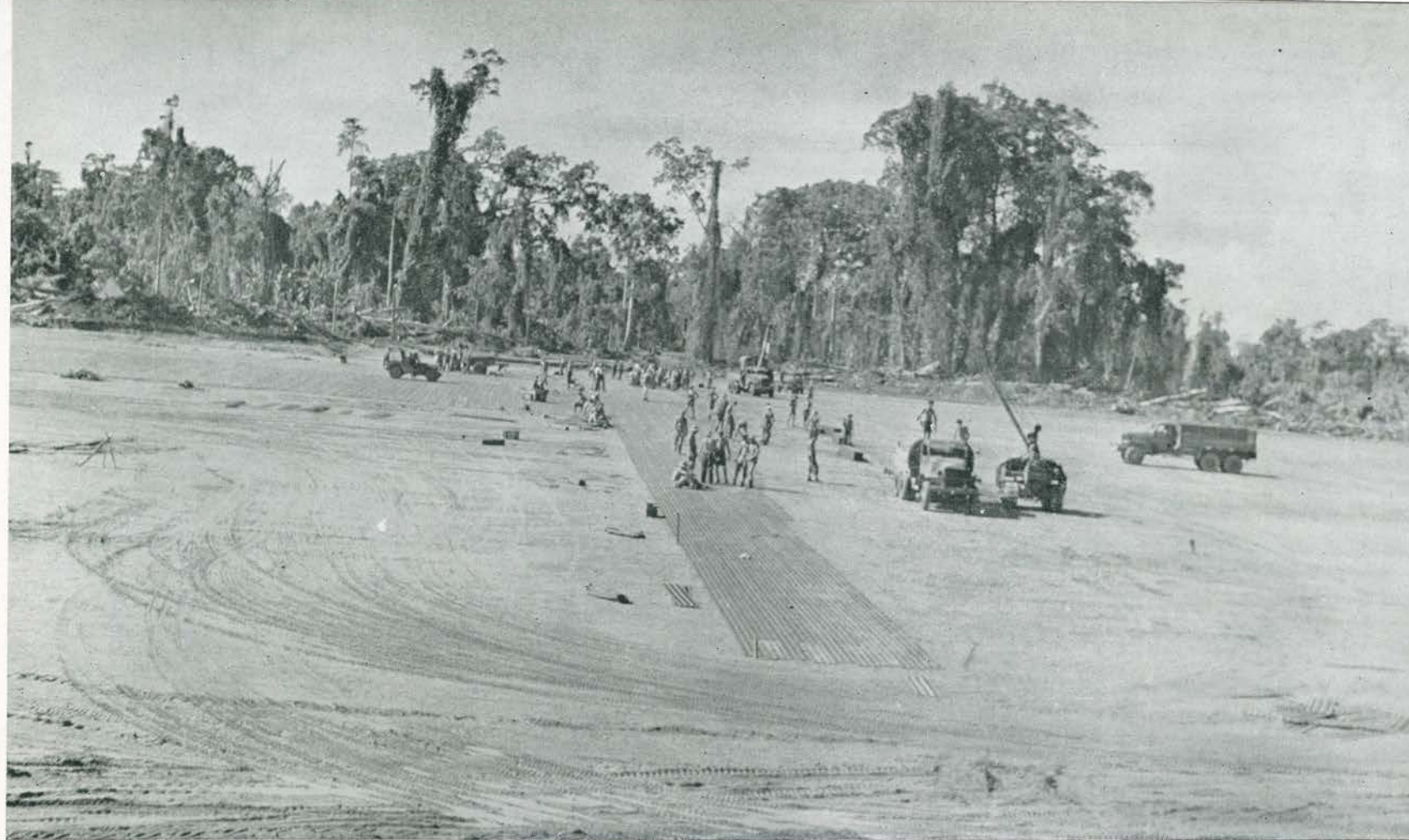
Apron Under Construction
