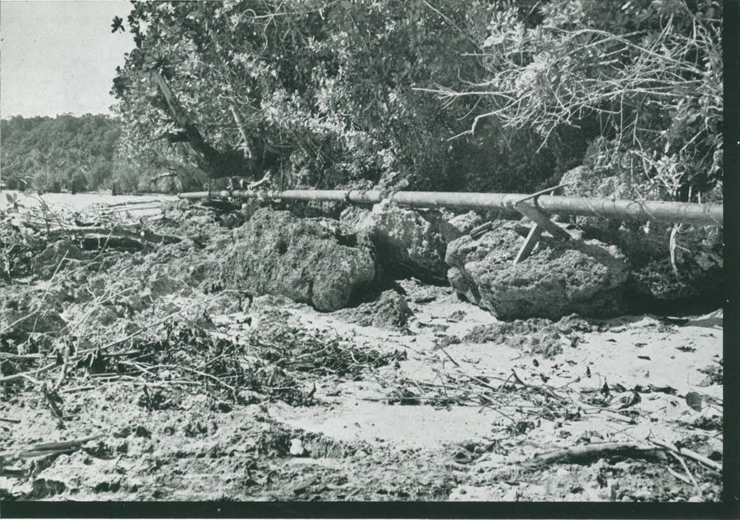
Pipeline Along Shore
