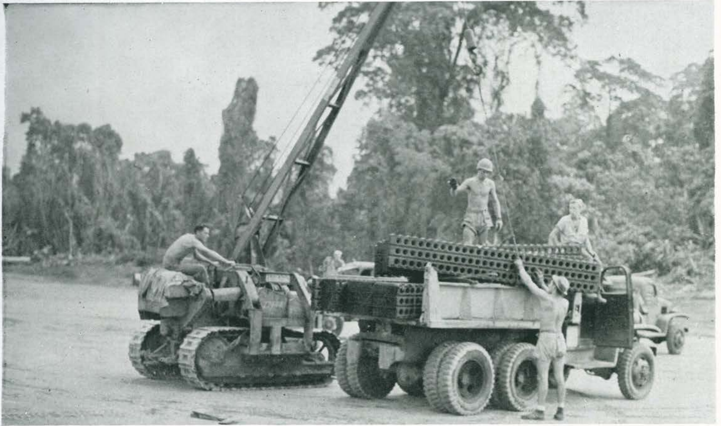
Unloading Pierced Planking
