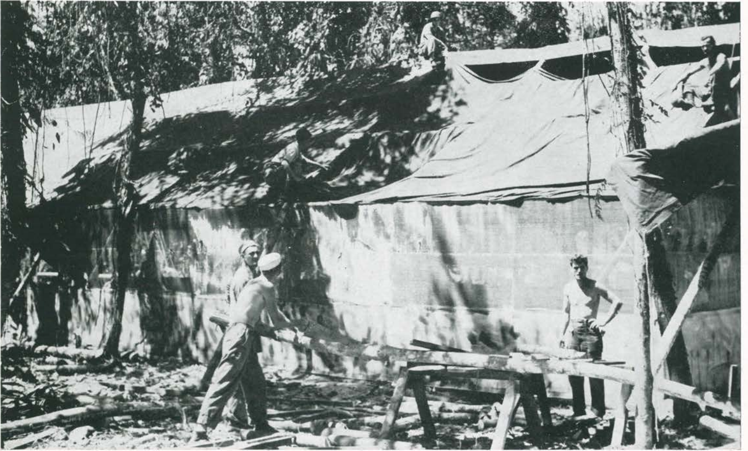
77th Mess Hall Going Up
