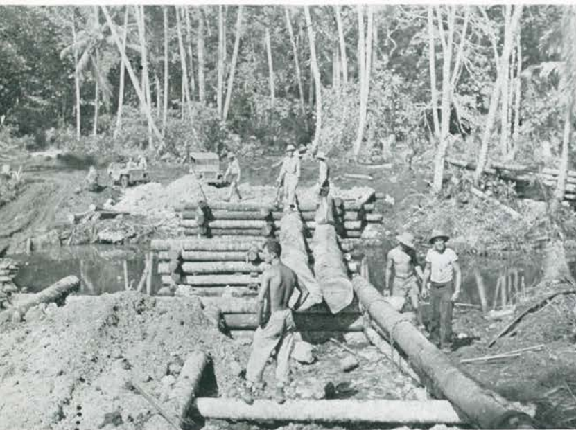
At left, reading from top to bottom: Temporary bridge—Biporo River. Beginning second bridge. Below, left: Open to traffic; right: Sawmill on Juno River.
