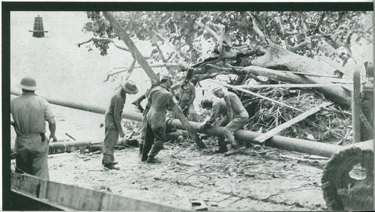
Welding Sea Line
