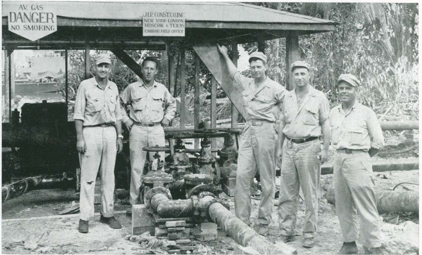
Hamburg Bay Pump Station
