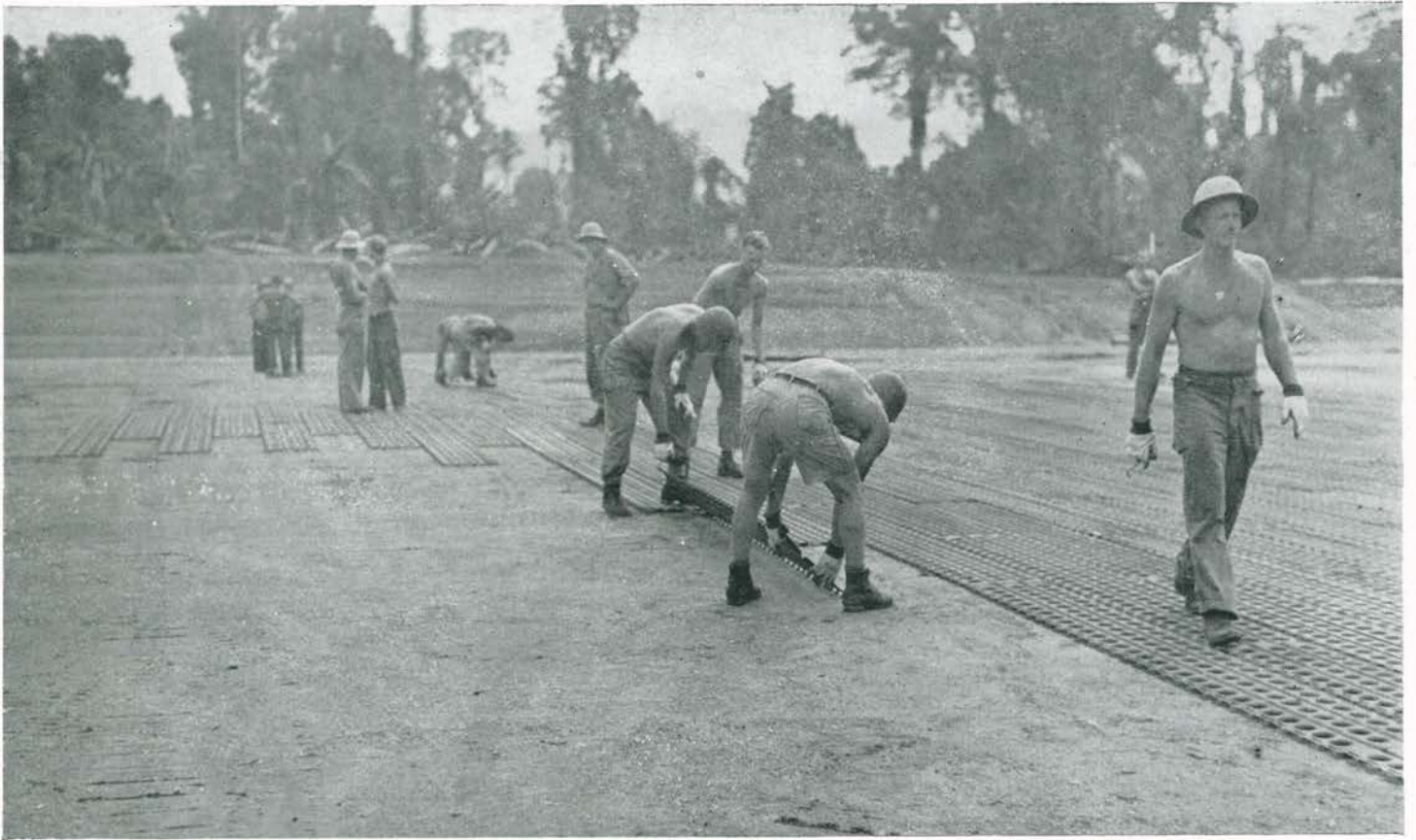
Laying Pierced Planking
