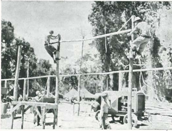
Framing 77th Machine Shop
