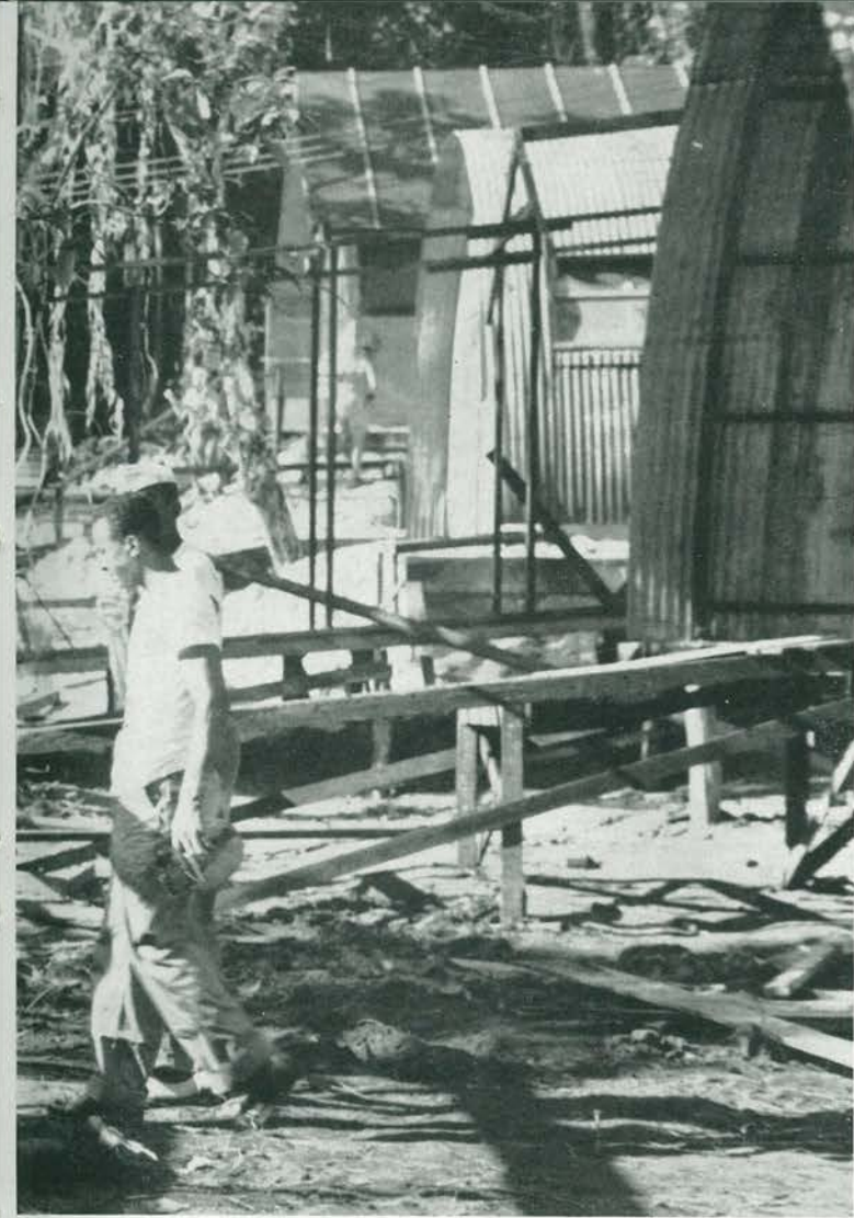
Ramp For Hospital
