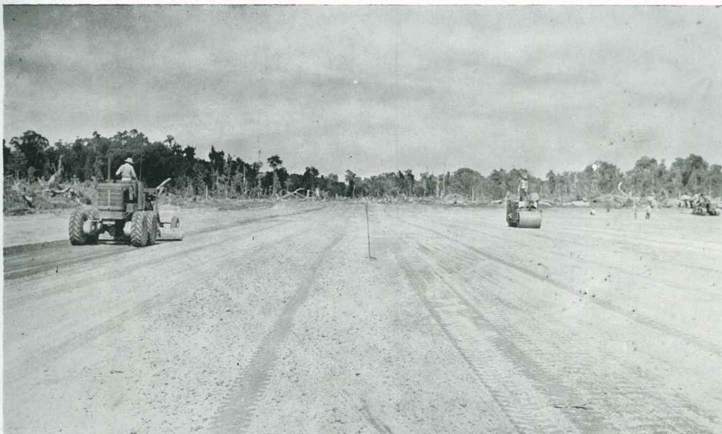
Rolling and Grading Extension
