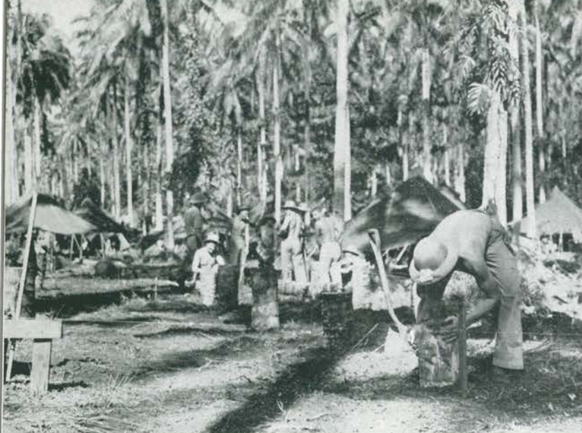
Setting foundation blocks for hospital
