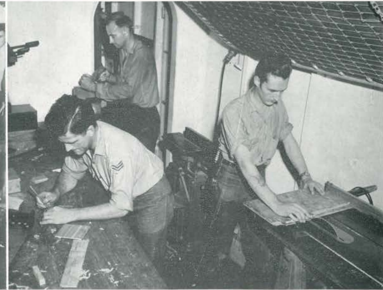
Carpenter's Mates at work in carpenter shop.
