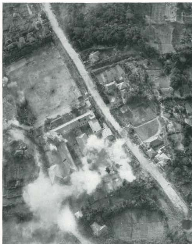
Destruction of large building 7 miles N/E of Naha, Okinawa.
