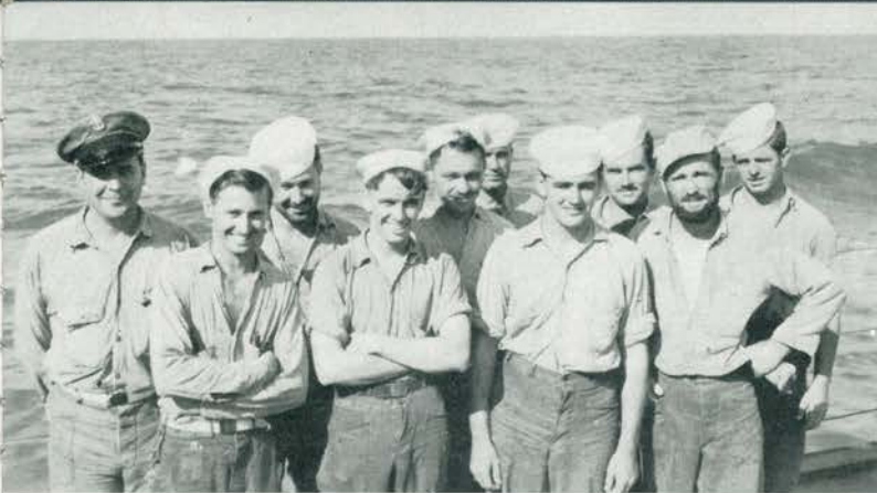
FORWARD FIRE ROOM
