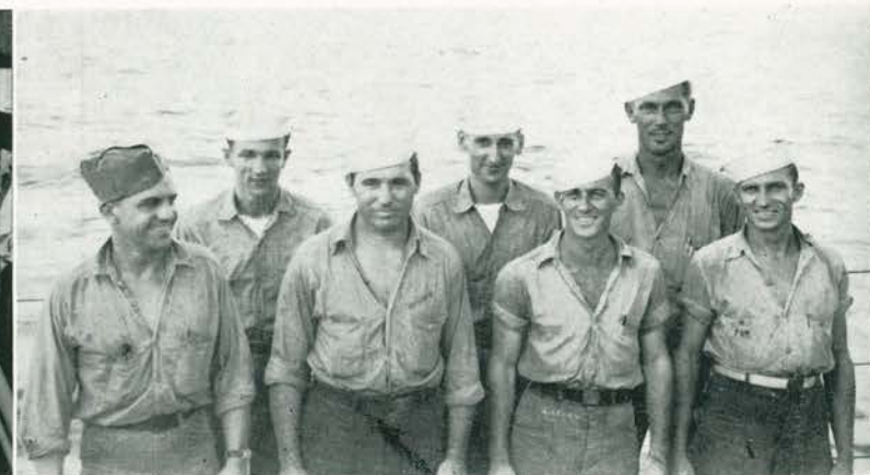
AFTER ENGINE ROOM
