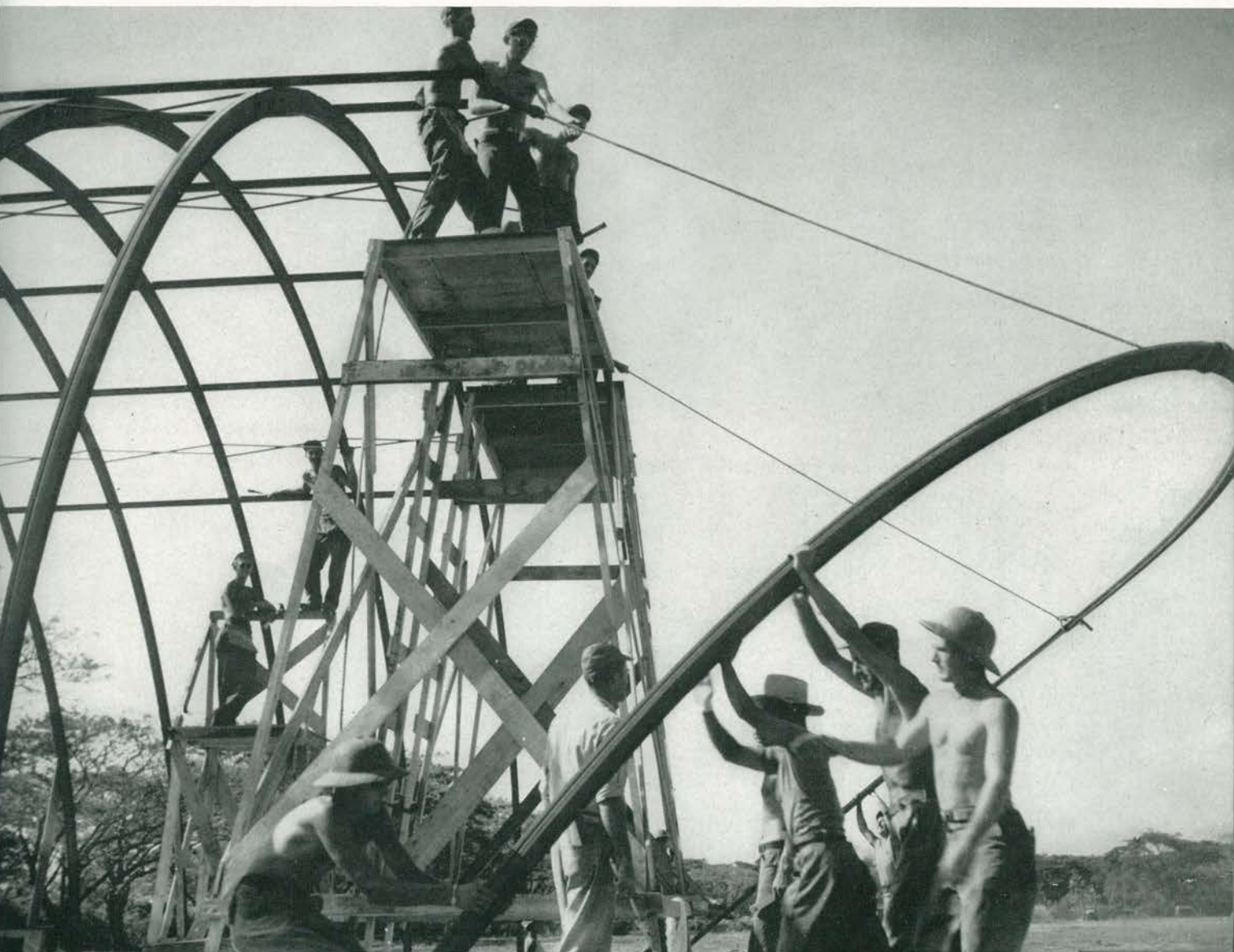
Raising an Arch Rib on a 40' x 100' Quonset Hut.
