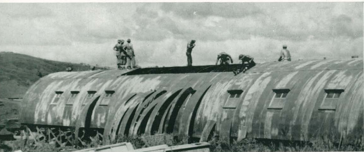
Another hut will soon be completed.
