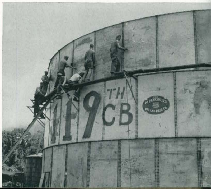
A final check on the bolts.
