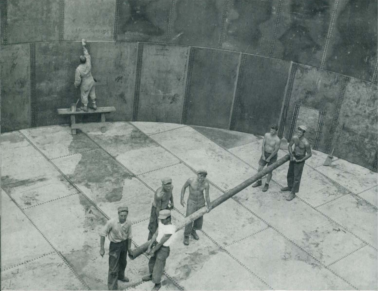
Erecting a steel storage tank.
