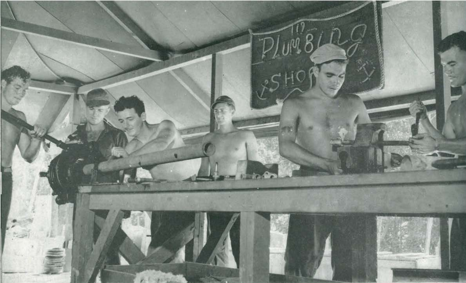
Threading pipe and making fittings before going out to major project.
