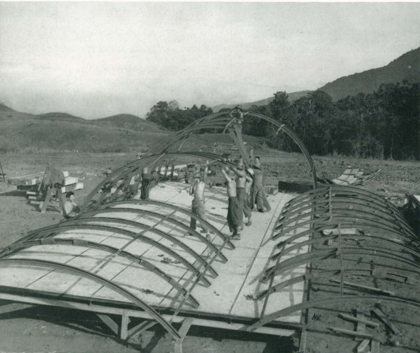
Raising the steel ribs for another Quonset Hut.
