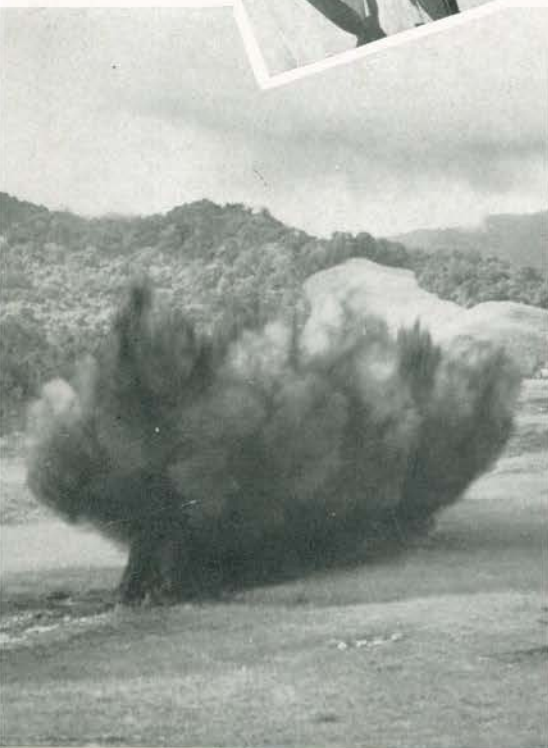
Blasting a ditch for malaria control
