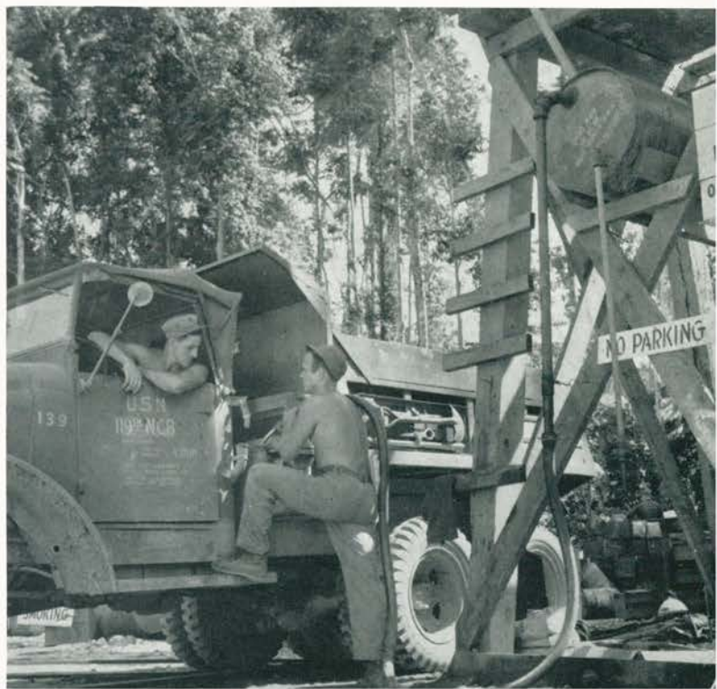
Herb Frazier "fills 'er up". This station consists of two pontoons placed 12 feet high to fuel equipment.
