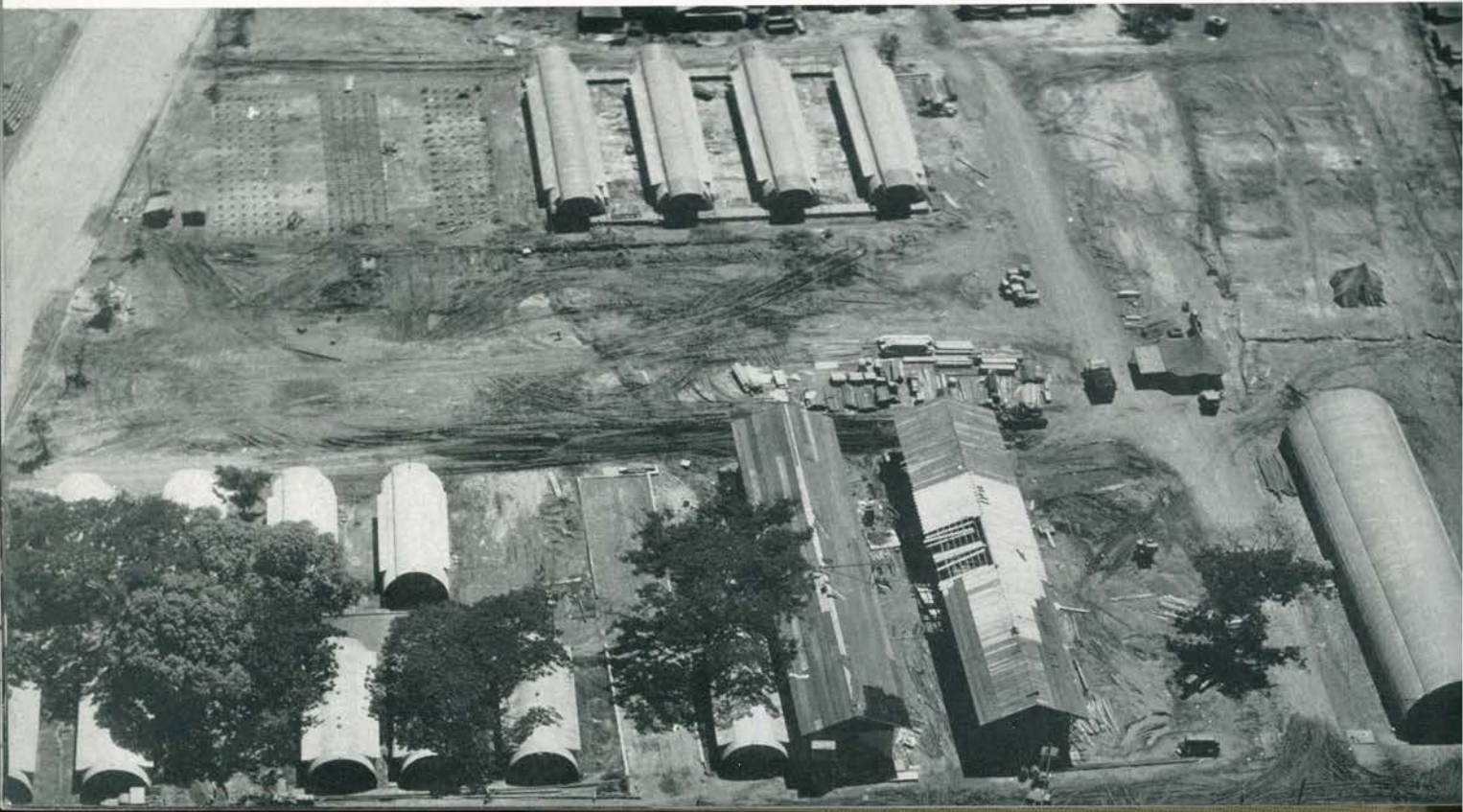
Facilities for Commander Naval Operating Base, Manila-Subic, under construction.
