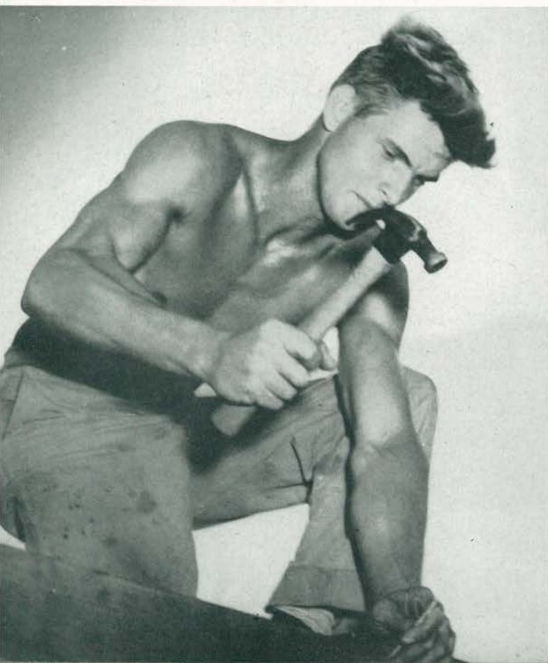
Woodrow Schelvan on construction work.
