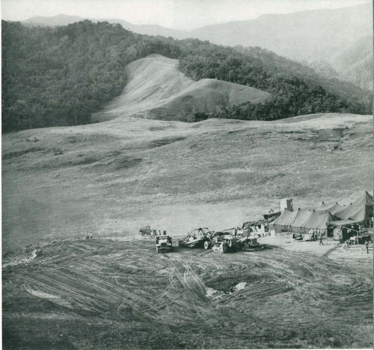
Breaking ground for the Lake Sentani camp.
