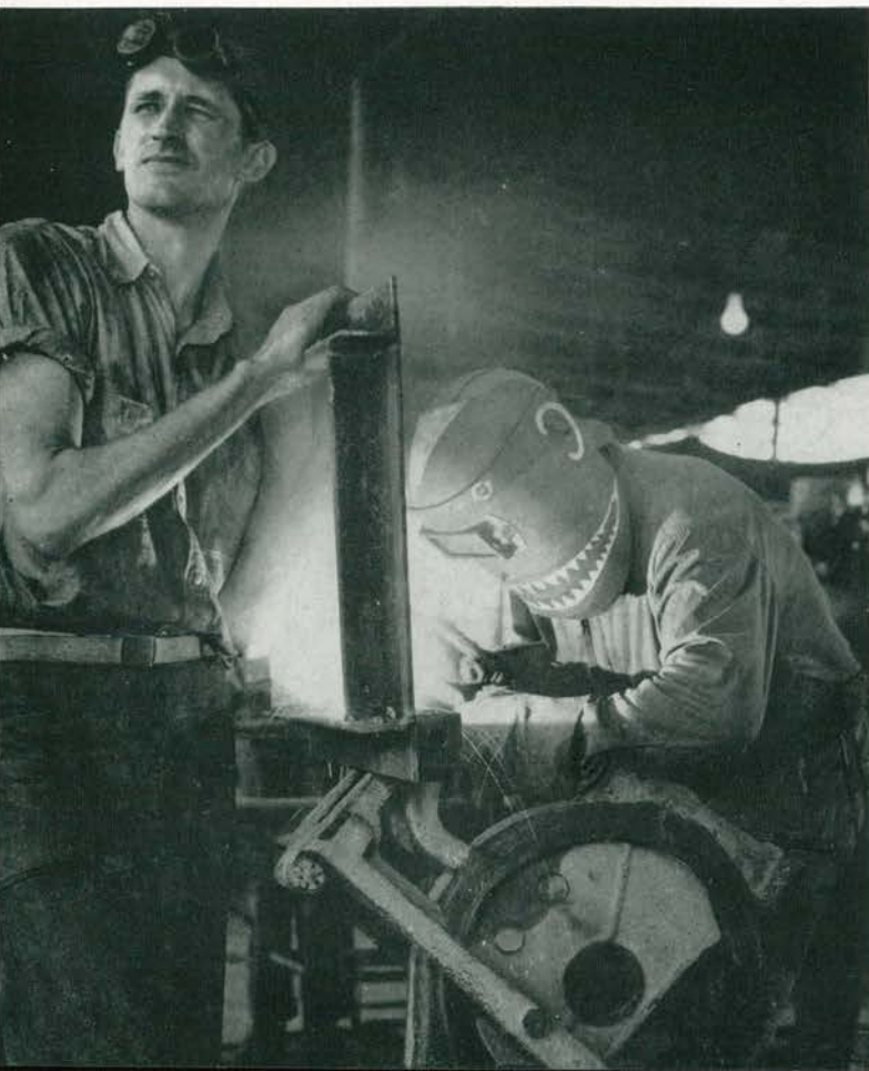
Lane and Sommers repair a Japanese anti-aircraft gun mount for use as a malaria control sprayer.
