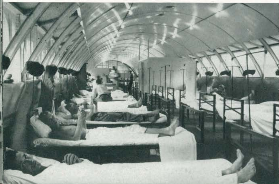
A wardroom in the new hospital addition.
