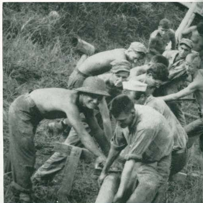
Laying the pipe lines for water.
