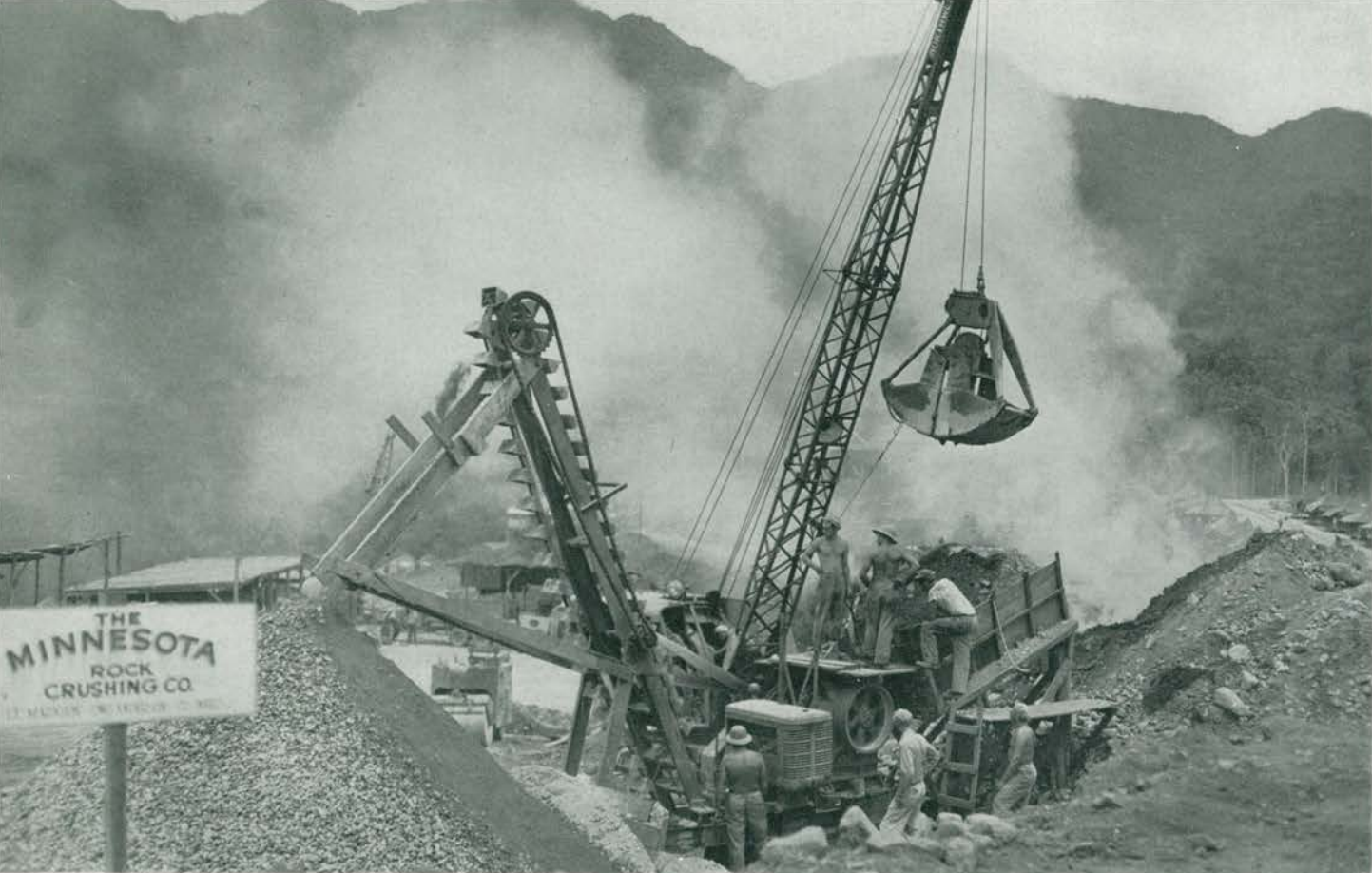
Crushing aggregate to be used in construction.
