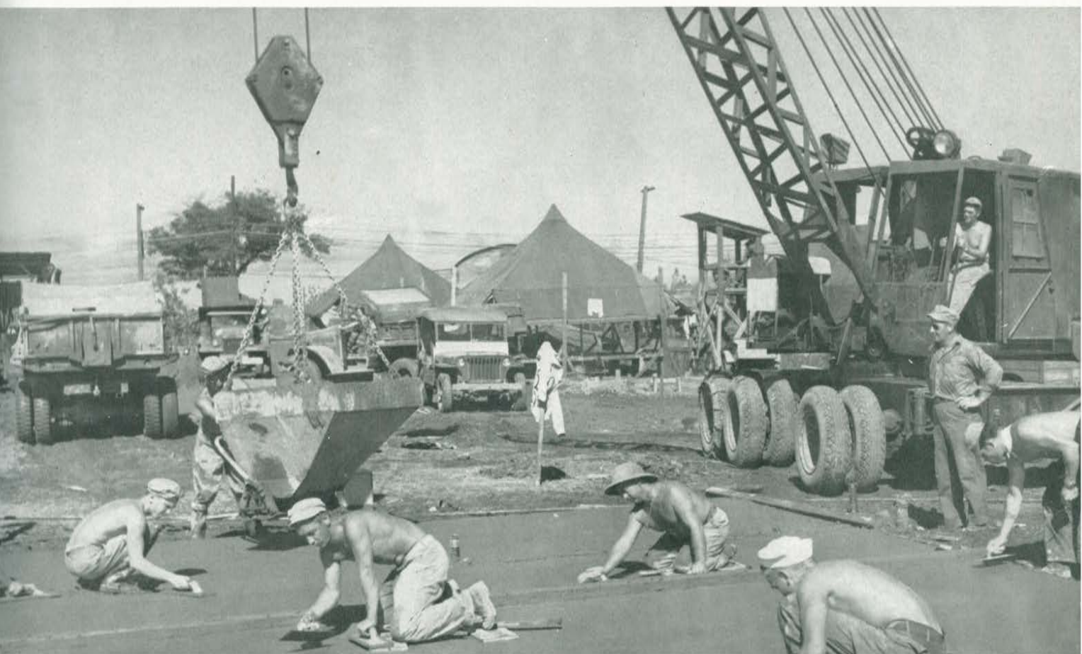
Chief Gier and crew finishing concrete.
