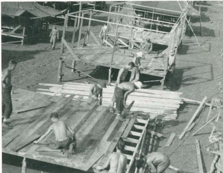
Building the enlisted men's quarters.
