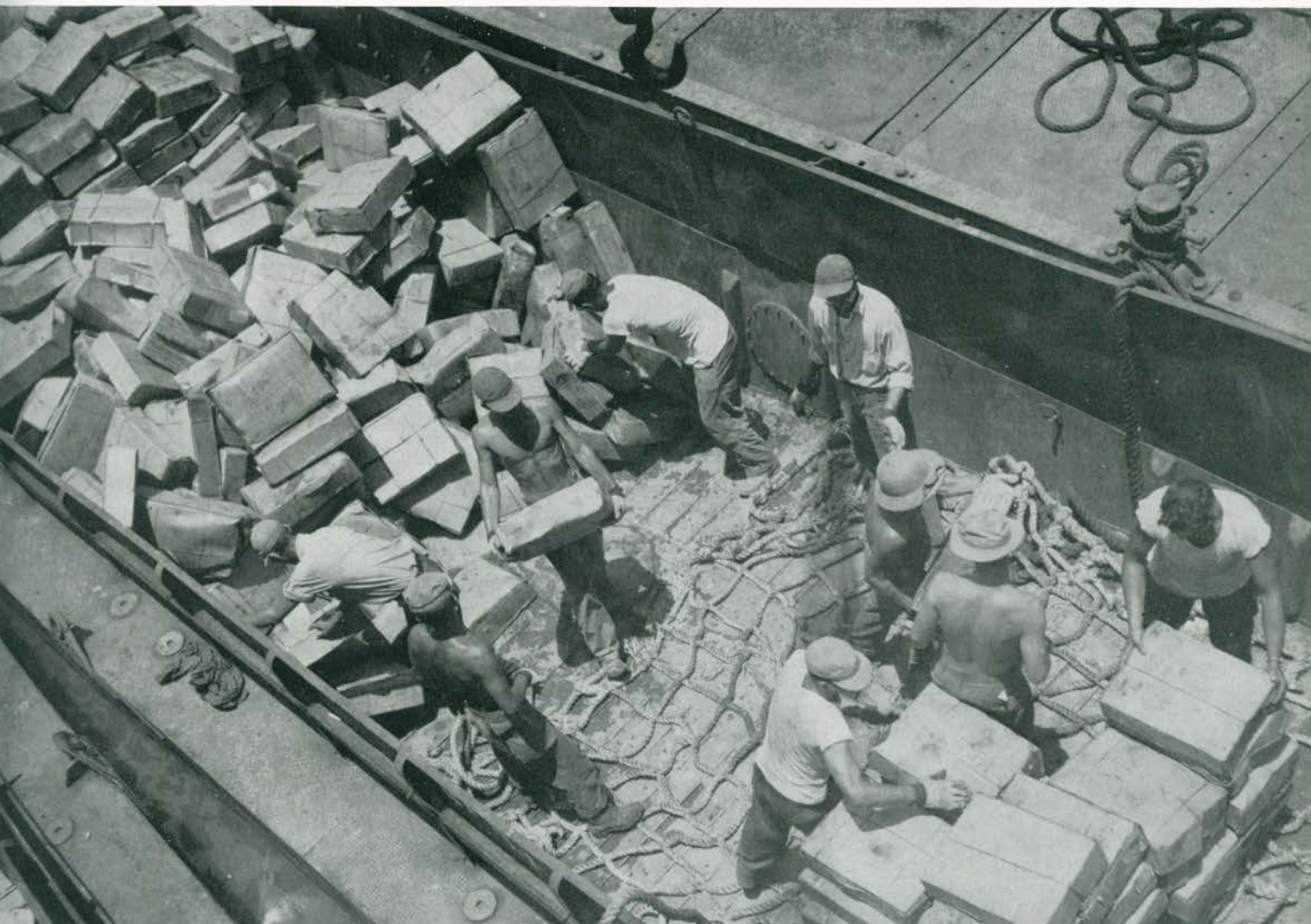
Unloading an LCM at a Pontoon Dock.
