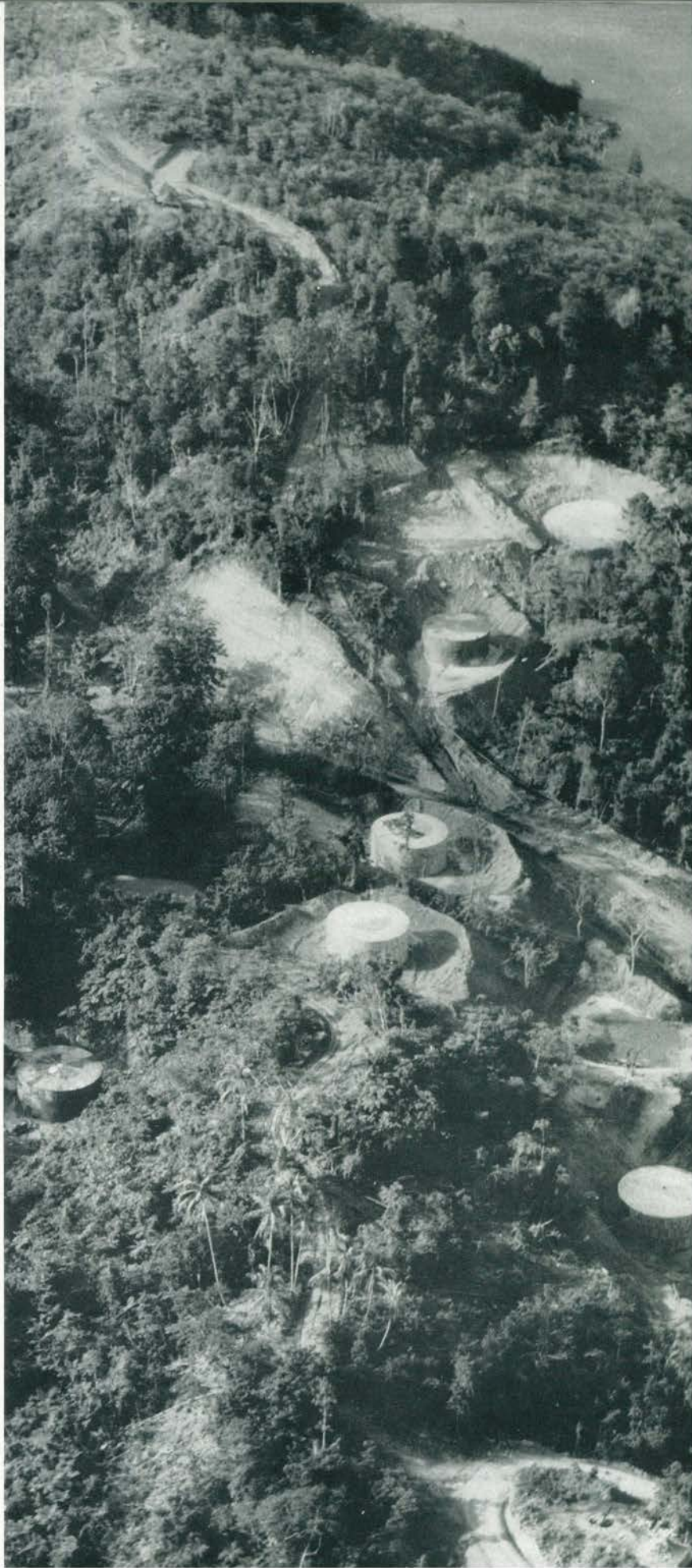
The Tank Farm — at Tanah Merah Bay.
