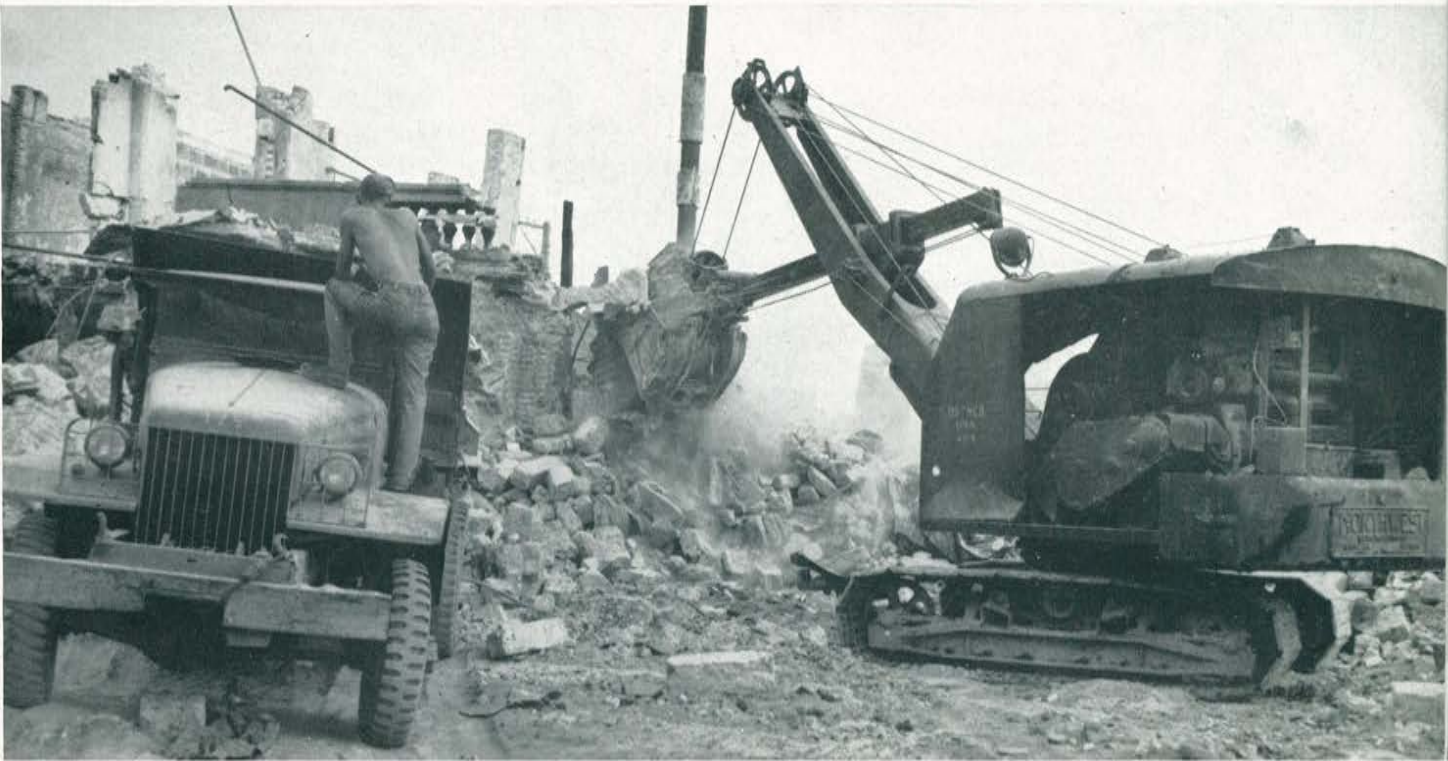
Clearing away the rubble for a construction site.
