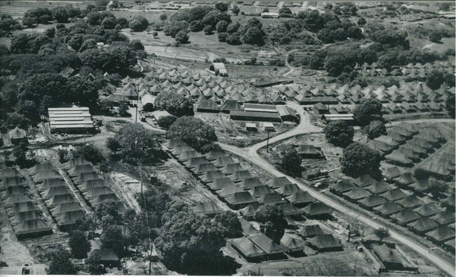
The camp built by the 119th USNCB for repatriated Prisoners of War at the 29th Replacement Depot.
