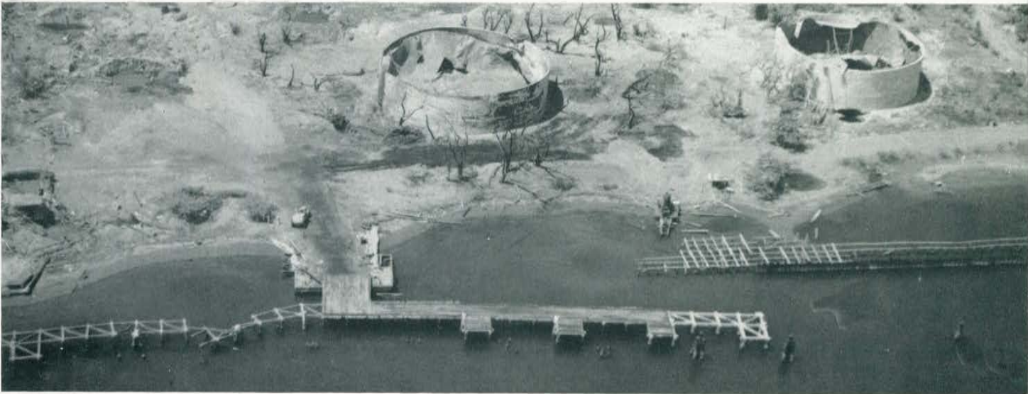
Wrecked docks and fuel tanks at Cavite.
