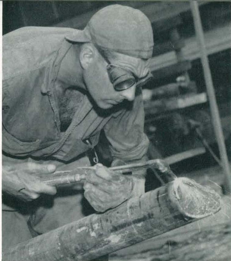
A welder makes another plumbing fixture. Plumbers installing soil pipe.
