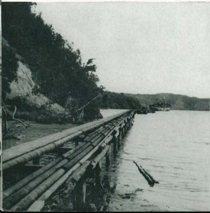
Oil and fuel lines on a jetty.
