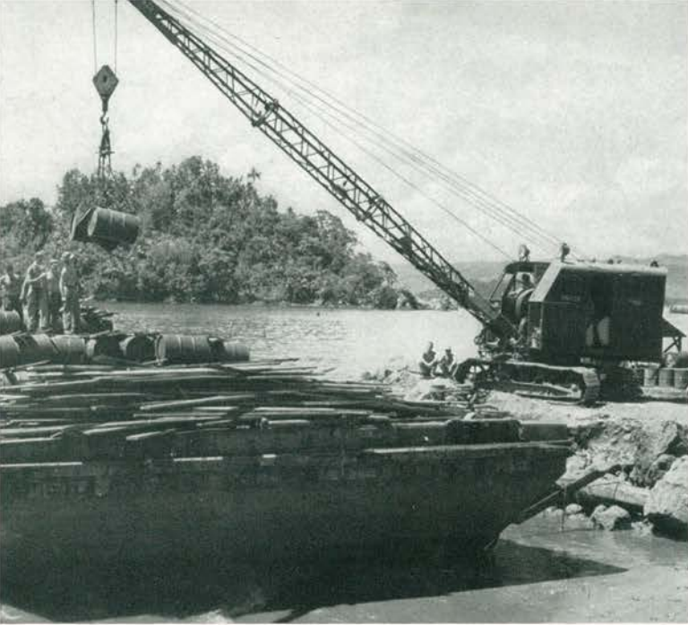
Fuel to run the equipment.
