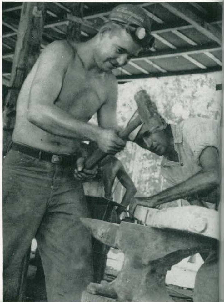
Seabee blacksmiths straighten bent tongue of carryall.
