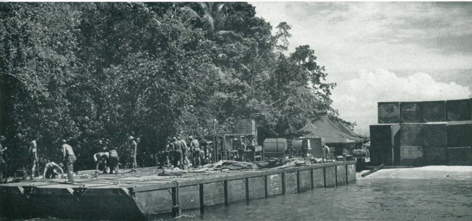
A completed pontoon barge ready to launch at Maderan in Hollandia Bay.
