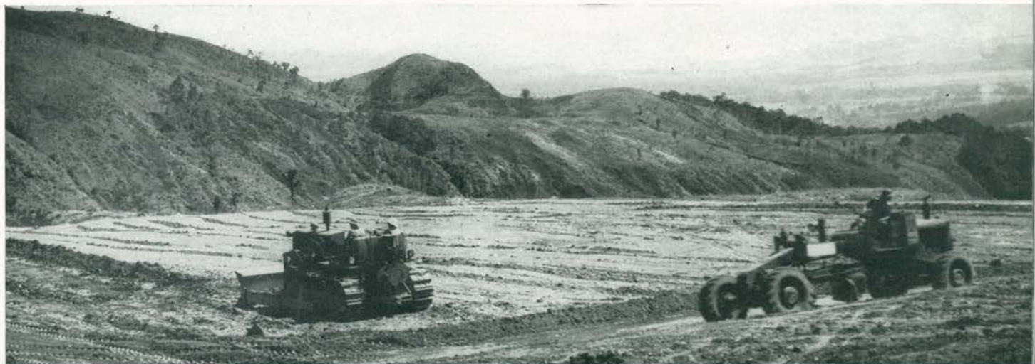
Grading on the Seventh Fleet Headquarters project.
