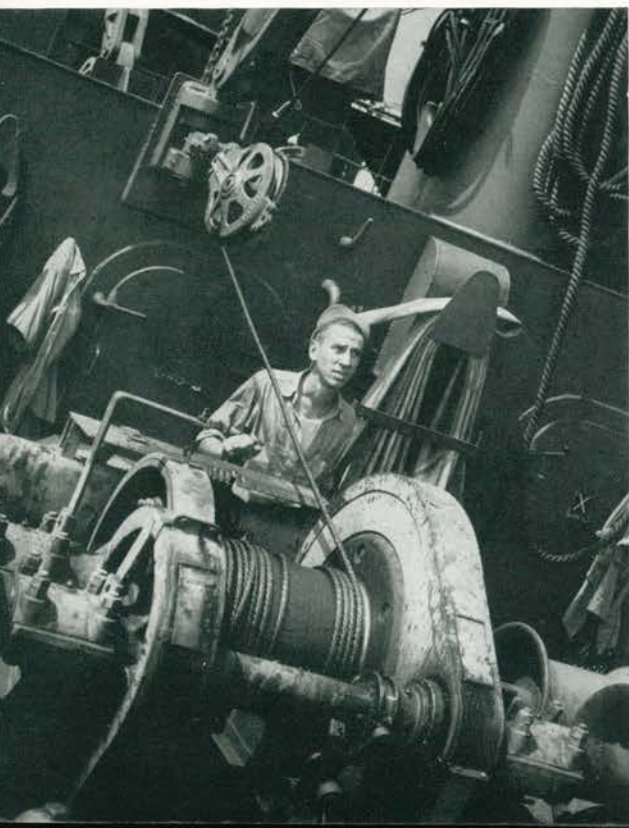
Winch operator making a lift out of hold of ship.
