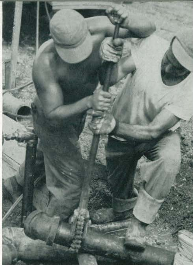
A welder makes another plumbing fixture. Plumbers installing soil pipe.
