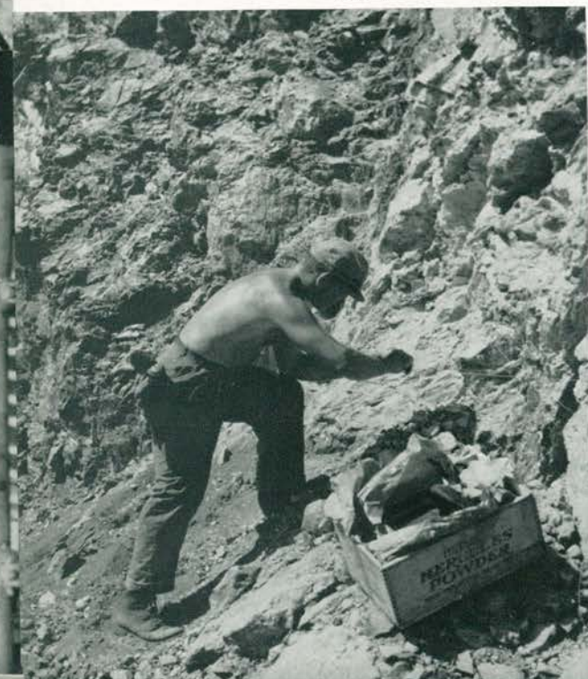
Placing charge for blast. Eugene "Boom Boom" Comtess attaching wires in series to blast loose gravel.
