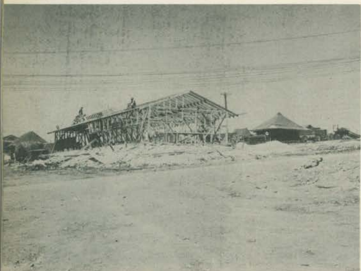
Mess hall construction—October 1944
