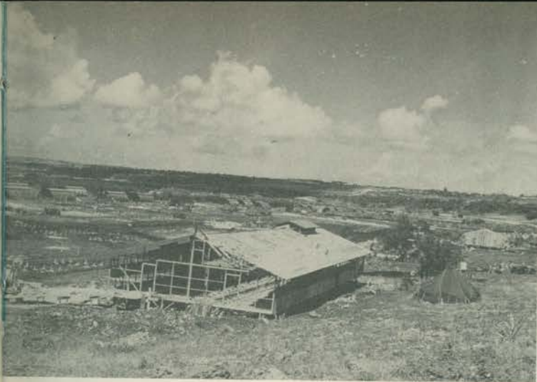
Mess hall (869th) construction—October 1944
