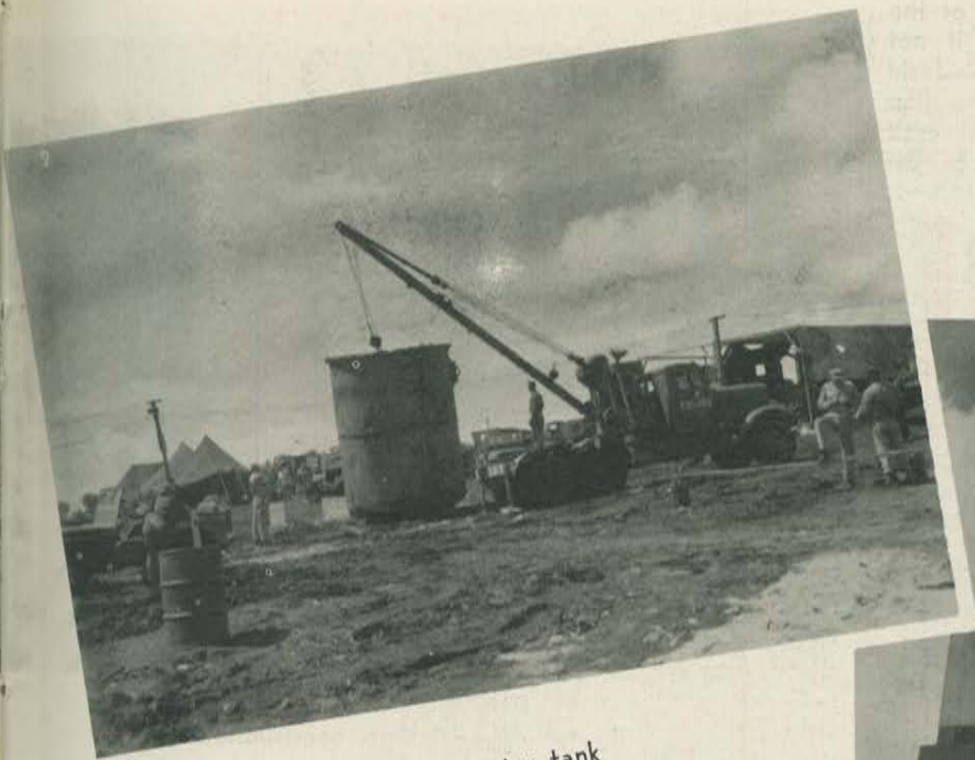
Erection of early water tank
