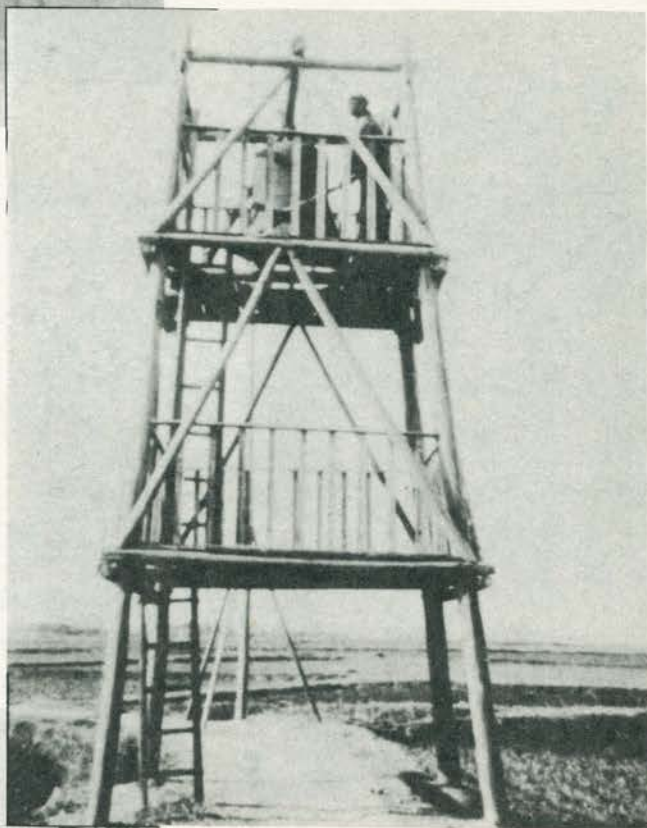
Fire alarm and lookout
