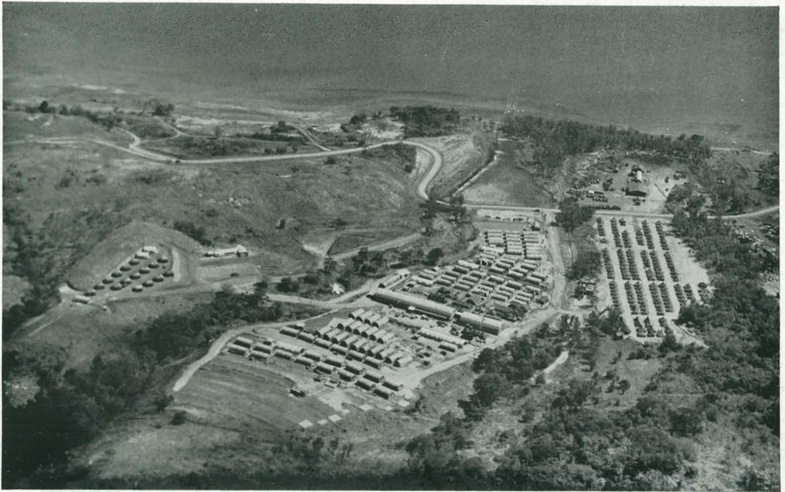
SMALL WORLD. Here is 87th camp lay-out as seen from approximately half-way up Monte D'Or. (For contrasting view taken from summit, see frontispiece, page 149.) In both classic shots, EARTHMOVER photographer, Edmund ("Jas") Jaskulski, has used camera to great advantage in show-
