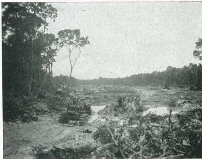
HITCH-HIKERS. A "snatch-cat" tows a huge stump and carries a couple of passengers. The small tractors had been used previously to drag logs out of the rough and up to the loading pits. It has been raining again!
