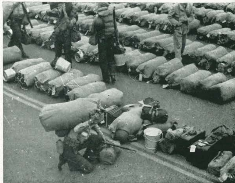
NO BAG INSPECTION. California's celebrated sun wilted even the sturdiest, barrel-chested Seabee as the long, tedious morning of waiting slowly spent itself. Mates have grounded bulging duffelbags containing bedding and are awaiting loading orders in nearby shade.
