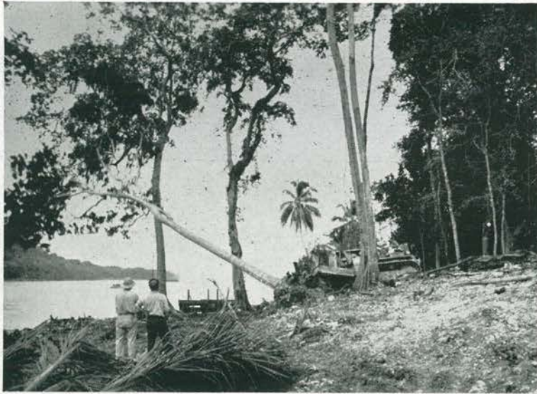
POWER. Initial clearing for Stirling Dock area begins. Jack Kenning (on D-8) pushes over sizeable tree—roots and all, thereby providing more fodder for the battalion sawmill. A stubby LCM plys its route between Stirling and Mono.
