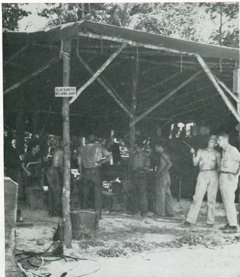
BLACKSMITHS AND WELDERS. By continuously making new machine parts and welding others that couldn't be immediately replaced, the blacksmith and welding shop operated day and night to keep strip equipment in tip-top operating condition right around the clock.
