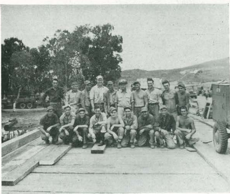
BRIDGE BUILDERS. Most of the credit for construction of seven fine bridges on tough Bourail job must go to Chief Inness and the 18 stalwarts of his hustling carpenter crew. Here, the entire gang knocks off for a group portrait.
