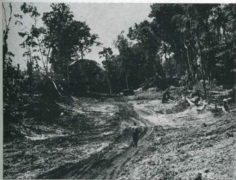
WIDE CLEARING, made for a main highway on Stirling Island, has been brushed out below airfield. Odd-shaped New Zealand truck was used by a Kiwi field bakery in delivering bread to various outlying units. Early roads weren't too good.
