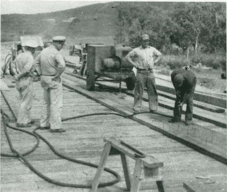
GOLDEN SPIKE? Four lanes of heavy top tread were eventually added to save wear and tear on the main decking of bridge. Chief Bill Inness, Lieut. Ray Pape and F. K. Jones observe as J. C. Jones drives a final row of spikes.
