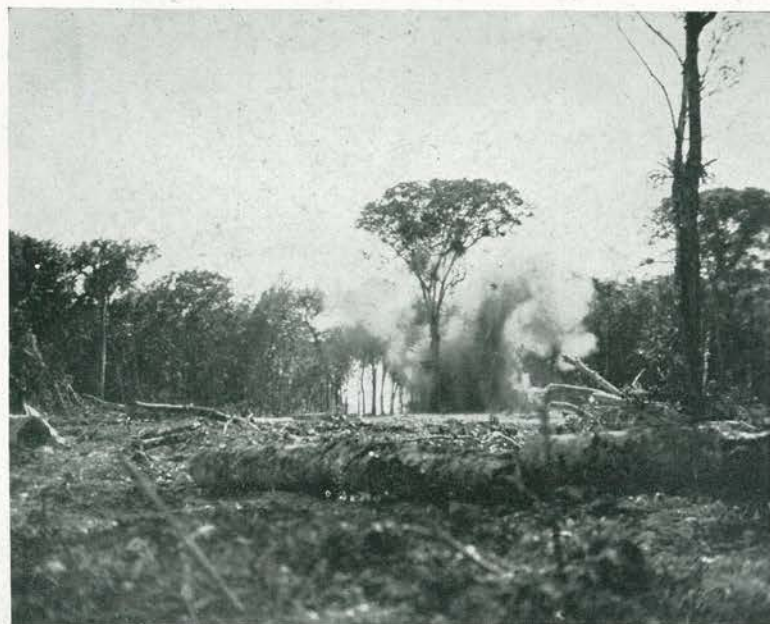
BLOWING IT OUT. Stalwarts like this required a little extra persuasion. This 48-incher, which is held up by large buttressing roots, proved too difficult for the 'dozers. A little "Can Do" and a shot of dynamite finally did the trick.
