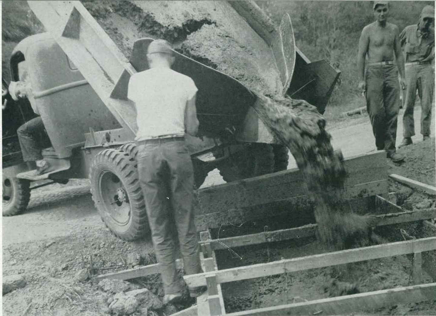
POURING THE MUD. Once the oil-drums were fashioned together and the supporting forms built, mixed concrete was driven up in trucks whose beds had been somewhat redesigned and poured through a rear chute. Mike Kocian and Raymond LaRue (right) stand back from wildly splashing
