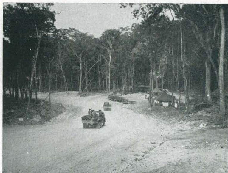
A MAIN DRAG on Stirling Island—a section of beach highway approaching the entrance road to ACORN 12 and the Pilots Camp area. This super-speedway, originally a trail 'dozed out' by invasion forces, was 40 feet in overall width.
