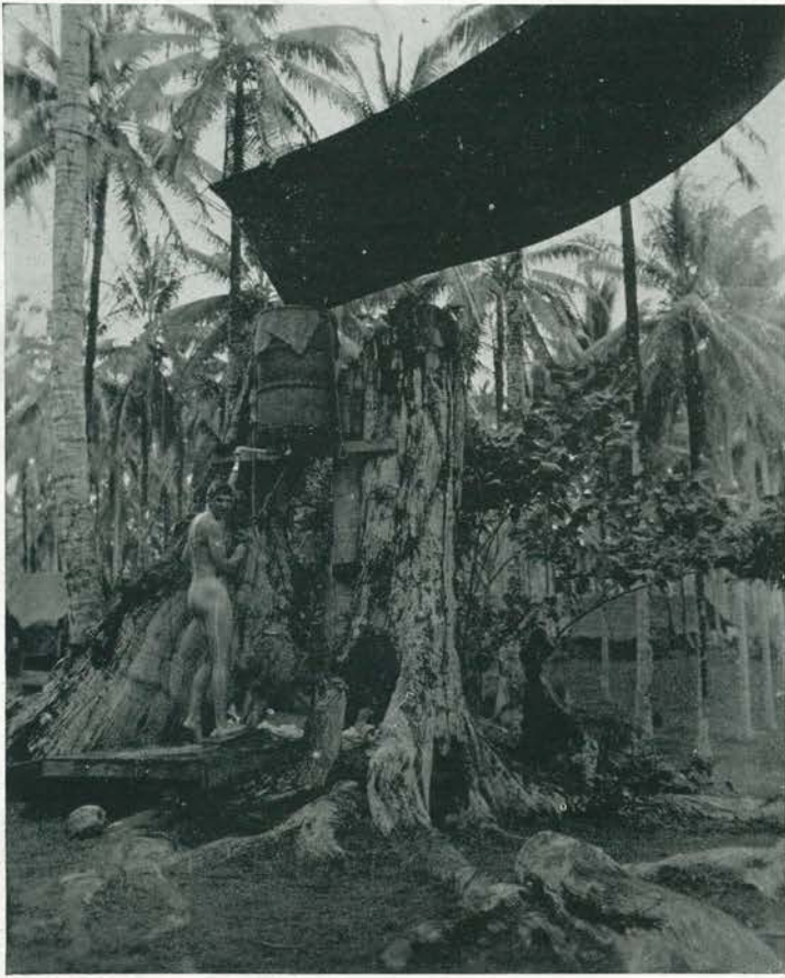
HOMEMADE SHOWER. Daily rains caused many individual showers to be erected. These consisted of tarps stretched between the trees and drums for the storage of water. Lt.(jg) "Bill" Hart makes use of shower set in hollow tree trunk.
