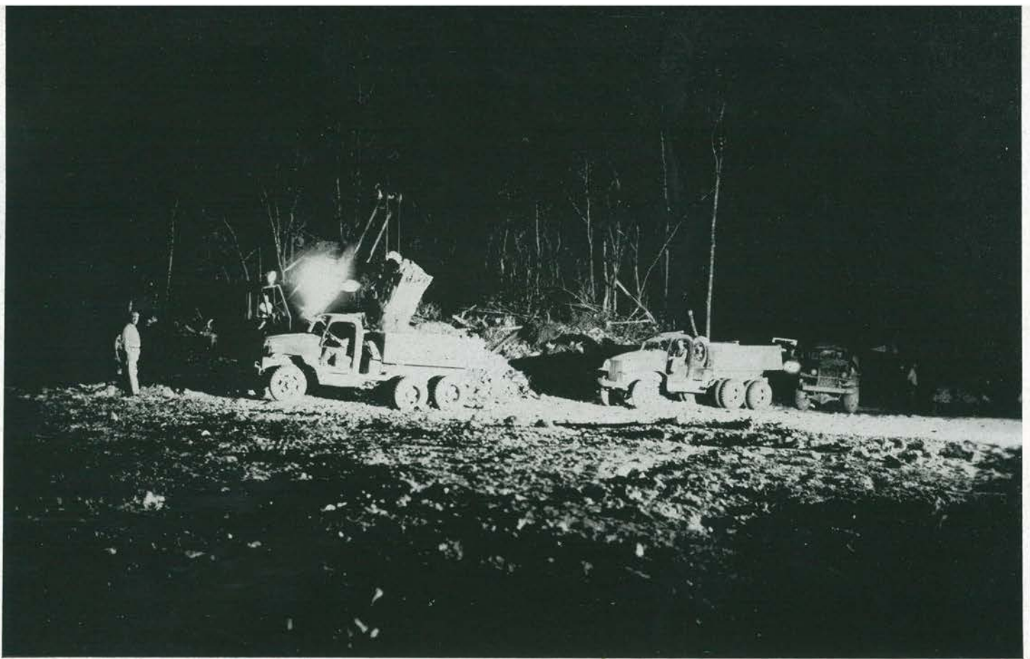
DAY AND NIGHT. The equipment didn't shut down until it broke down unless Jap bombers came over. This was a quiet night with everything running smoothly as the stripping operation progressed. There were four spreads like this clearing at the edge of the
