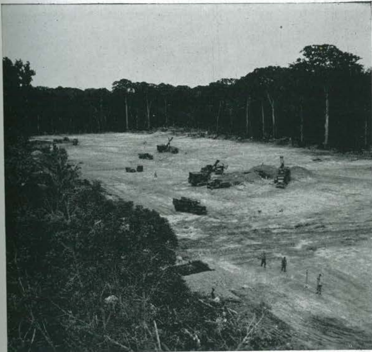
STRIPPING DOWN. This area is almost cleaned up. Soon the shovels can be moved to a borrow pit and the pan spread can come on through to perform its phase of the work. Excavations were former 90-mm. gun pits.
