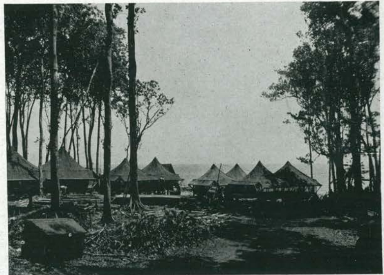
PILOTS CAMP is well under construction. Carpenters (center) are completing tent decks. Replete with screening and framework, these tents provided cool, comfortable living quarters for combat-weary P-38 pilots at Stirling. A mess hall and shower rounded out camp.
