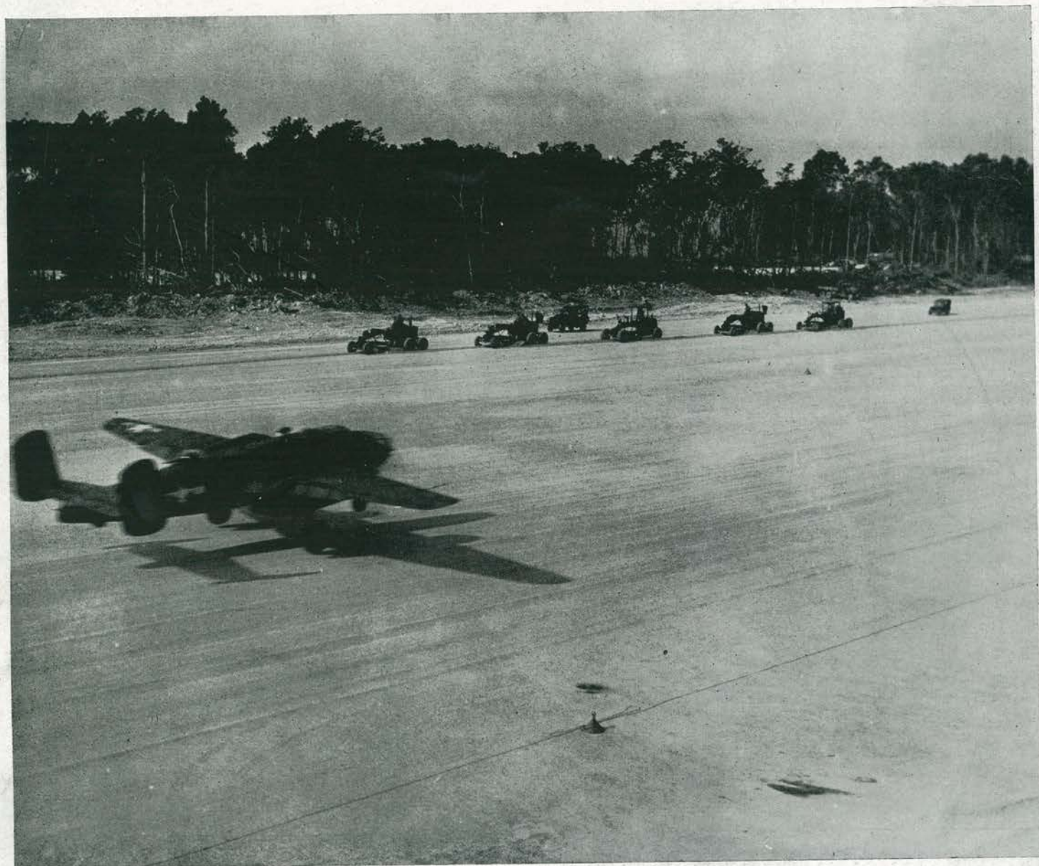
RAIDERS AND GRADERS. A B-25 takes off as part of a strike against last remaining Japs in the Solomons without interfering with a grading spread. It was usually necessary to clear runway when a mission was taking off or returning. It was this constant handicap that made it necessary
