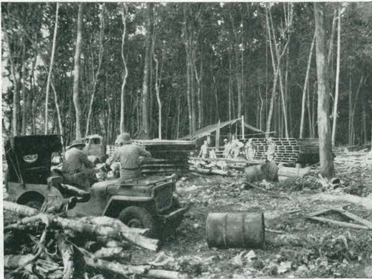
FIRST CARPENTER SHOP, set up in rough clearing, consisted of tarps to cover saws. Half sections of tent decking were assembled here and trucked to jobs where other carpenter crews put them together. This assembly line system speeded operations immeasurably.
