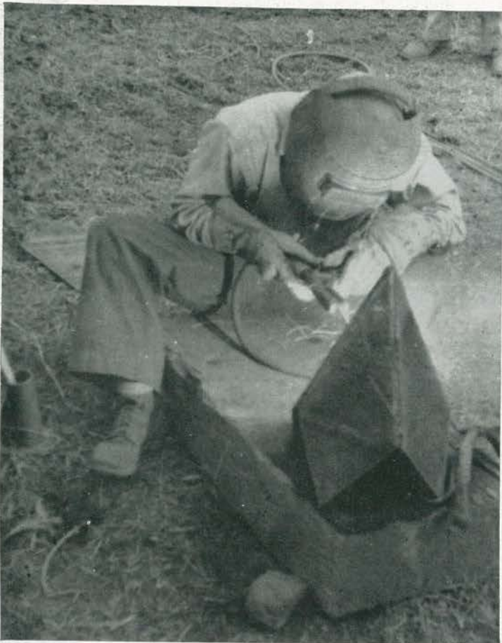
SHOEMAKER. Frequent solid-rock ledges in river beds presented formidable obstacles to pile-driver. Only after pointed shoes of steel plates were fashioned together and attached to the leading end could piles be driven home. Tom Clements is welding.
