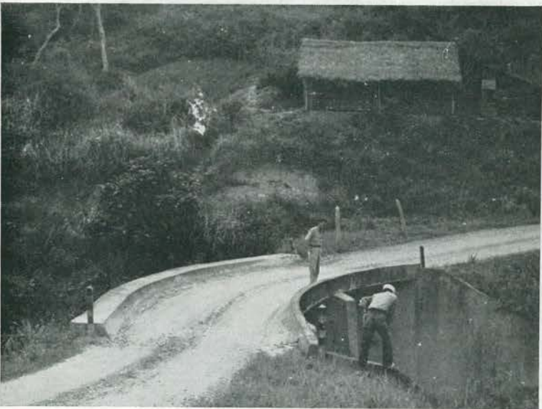
INSIDE CURVE. In sharp contrast to modern road and bridge construction methods of Seabees were the primitive, hand-made efforts of the native French. Lack of equipment and proper materials, coupled with different ideas, resulted in this curved curiosity.
