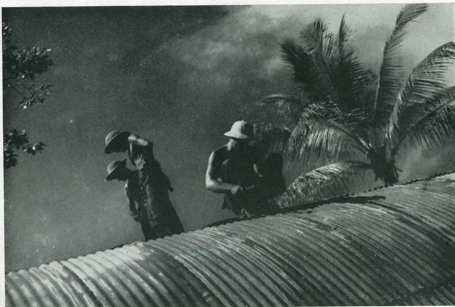
TOPPING IT OFF. Richard Bogdanski and Charley Danford consult on the finished product while Clarence Nielson nails last section of quonset roof in place. While working in the open, sun helmets were a necessary item of apparel. Tender, young palm at right (one of a few growing any dis-
