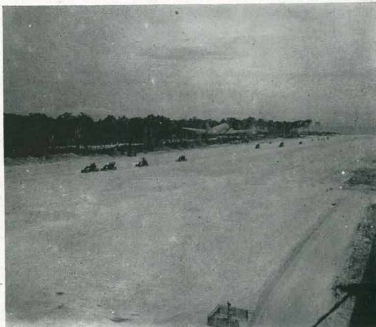
CROWDED OPERATIONS. A huge SCAT transport, loaded with top priority passengers and freight, prepares to take off as re-blading of runway continues at furious pace. Weather station's theodolite, used for making wind observations, is inside picket fence enclosure.
