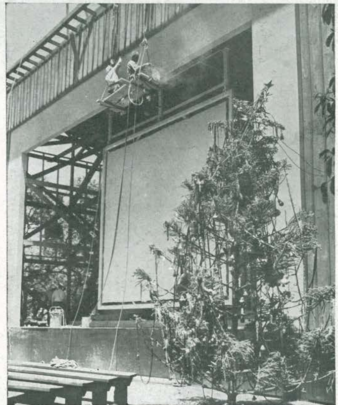
SPRAY BOYS. Albert Mundy and Sheldon McCaleb get in the last licks on the otherwise completed screen and stage from swinging scaffold. One of several community Christmas trees is already decorated and wired for lighting in anticipation of pageant.
