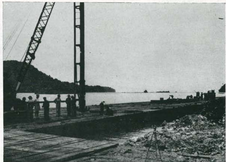
PILE-DRIVER rig is poised to sink one of many piles used for dolphins and clusters. Piles were sharpened and steel-tipped to secure them in coral bottom. Net tender and barge (right) are laying submarine net across harbor entrance.
