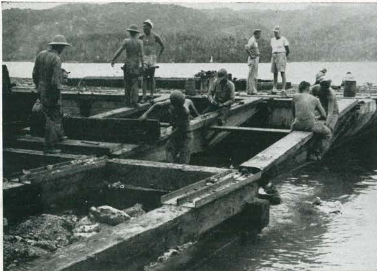
THE DETAIL. Heavy ramps from pier to shore are put into place. Timbers for the ramps were made of heavy native lumber cut to order by battalion sawmill. Four ramps of this type connected the pontoon pier to the land. Such work had to be right.
