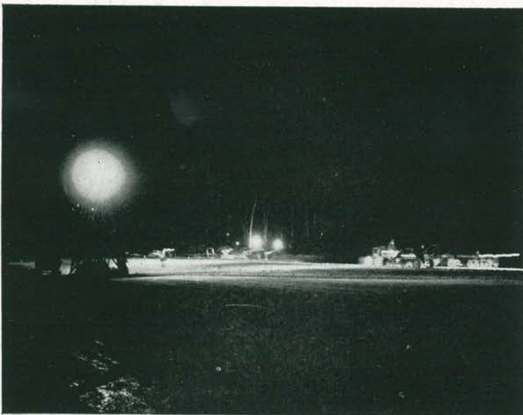
YOU ROUGH IT OUT, then finish it off! It's all in the day's work. The fine-grading equipment follows right along behind the heavy units. Those men at the light towers aren't mere spectators. Alert goes on, lights go off!
