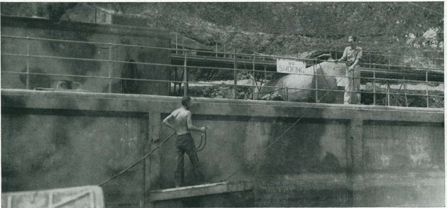
SPRAYING IT ON. Sheldon McCaleb (with spray gun) stands on small raft while painting sides of gasoline barge. Albert Mundy gives him a tow from the rail. These craft had crews of 15 with a CPO in charge. Lacking motive power of their own, they were towed to destination by sea-
