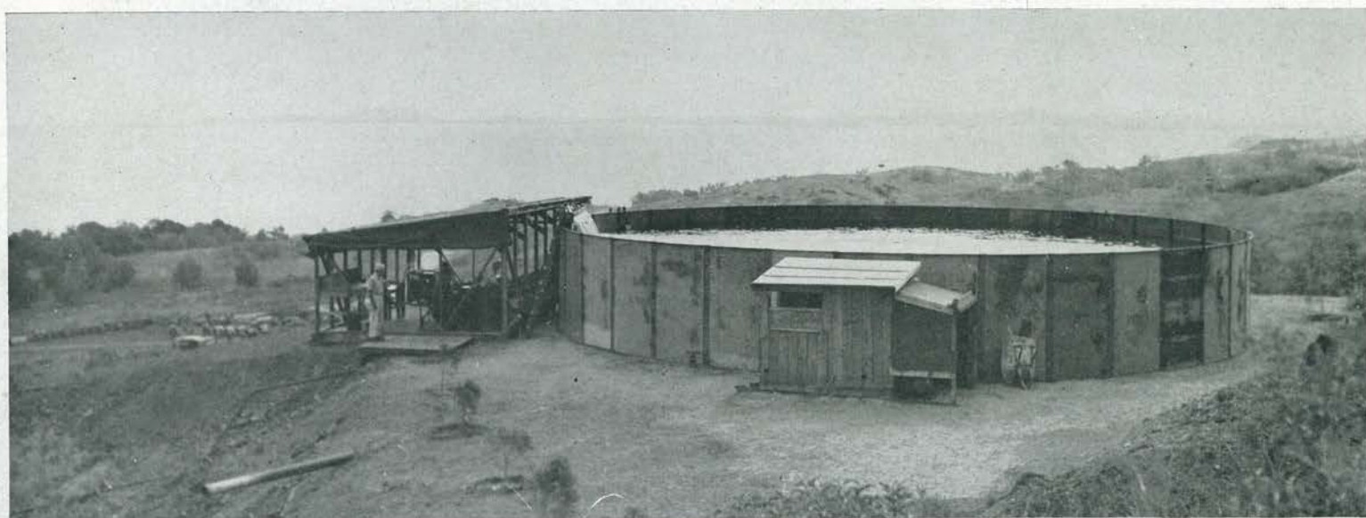
SOME CONTAINER! One section of a 10,000-barrel, bolted steel tank served as the water storage point for entire camp. Planned by Carpenter Tom Bailey and rushed to completion by Christmas Day, the filtration unit
