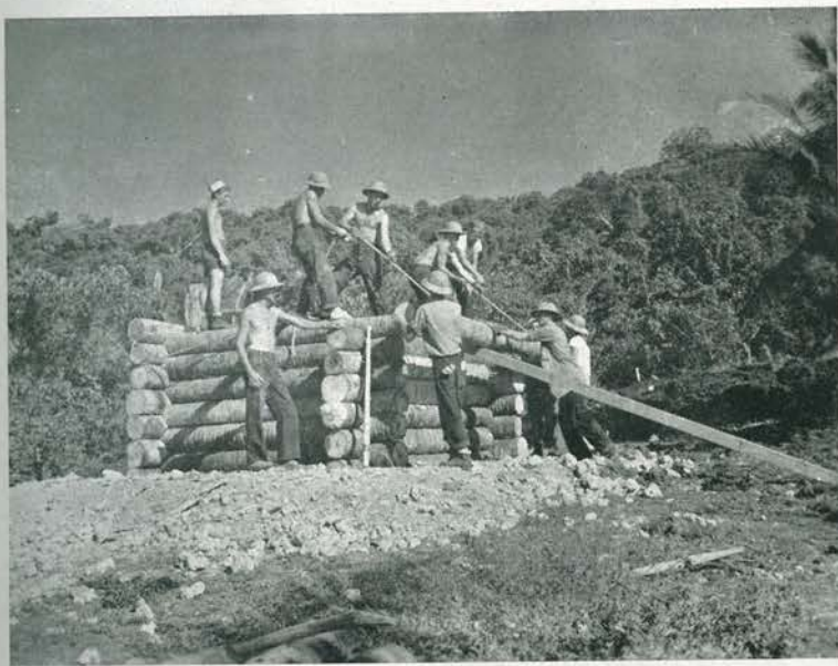
LOG ROLLING. Chief Vic Cedarstaff supervises construction of one of the many blockhouses built around the island for ammunition and dynamite storage. Heavy coconut logs were plentiful, of course, but their pulpy texture made them heavy and difficult to saw.
