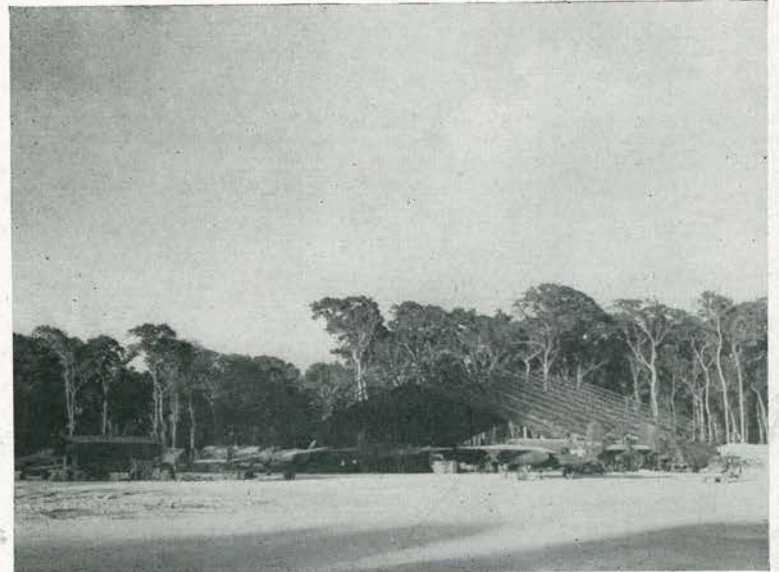
SICK CALL. Wounded aircraft are crowding completed hangar for "treatment." Structure had been erected on three other islands and 87th riggers were able to use only 11 of 13 main trusses. This plane "hospital" was constructed for the 25th Fighter Squadron.
