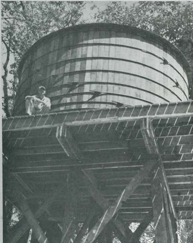
WATER TOWER. Towering virtually as high as the tallest surrounding jungle monarch, this imposing water tower supplies the pressure for the entire Camp Ostran water system. Perched high on the supporting platform, Lieut. William C. Reilly looks his project over.
