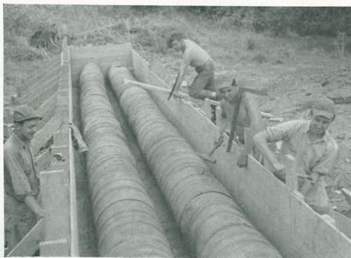
DRUMMERS. Oil drums (with ends out) were spliced together in long double rows and set on concrete foundations for culverts. Carpenters, like Ray Pursley's crew, then built forms around drums for other three sides. Others shown: Nelson, Stuchlik and Straz.
