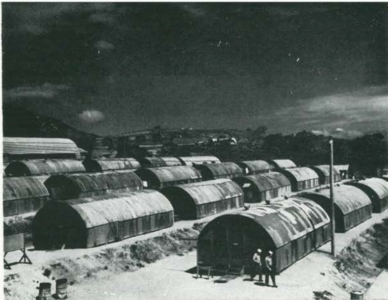
SEABEE HIVES. It was only a matter of days until almost everyone was comfortably settled under metal roofs. Located on a sharp slope, the rows were first terraced to keep the huts on an even keel. Officers Country is in background.
