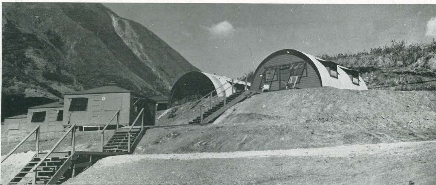
TOP OF THE HEAP. Comdr. Easterly and Lt. Comdr. Flynn occupied the three-room quonsets shown on upper terrace. The breath-taking view from this highest level surpassed all others in the area. Equipped with run-
