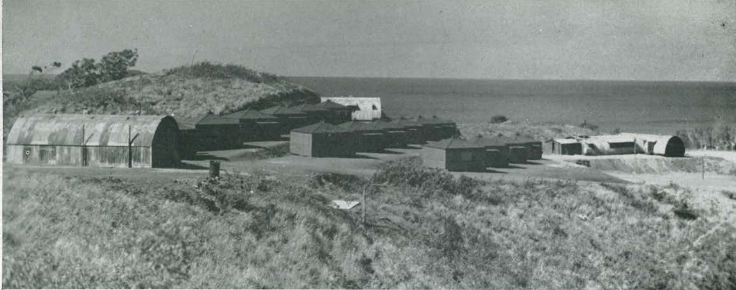
THE HILL. Igloo-like Dallas huts, small quonsets and a choice location established Officers Country at Monte D'Or as a snug, comfortable community. Erected long after the crew camp was completed, it was never-
