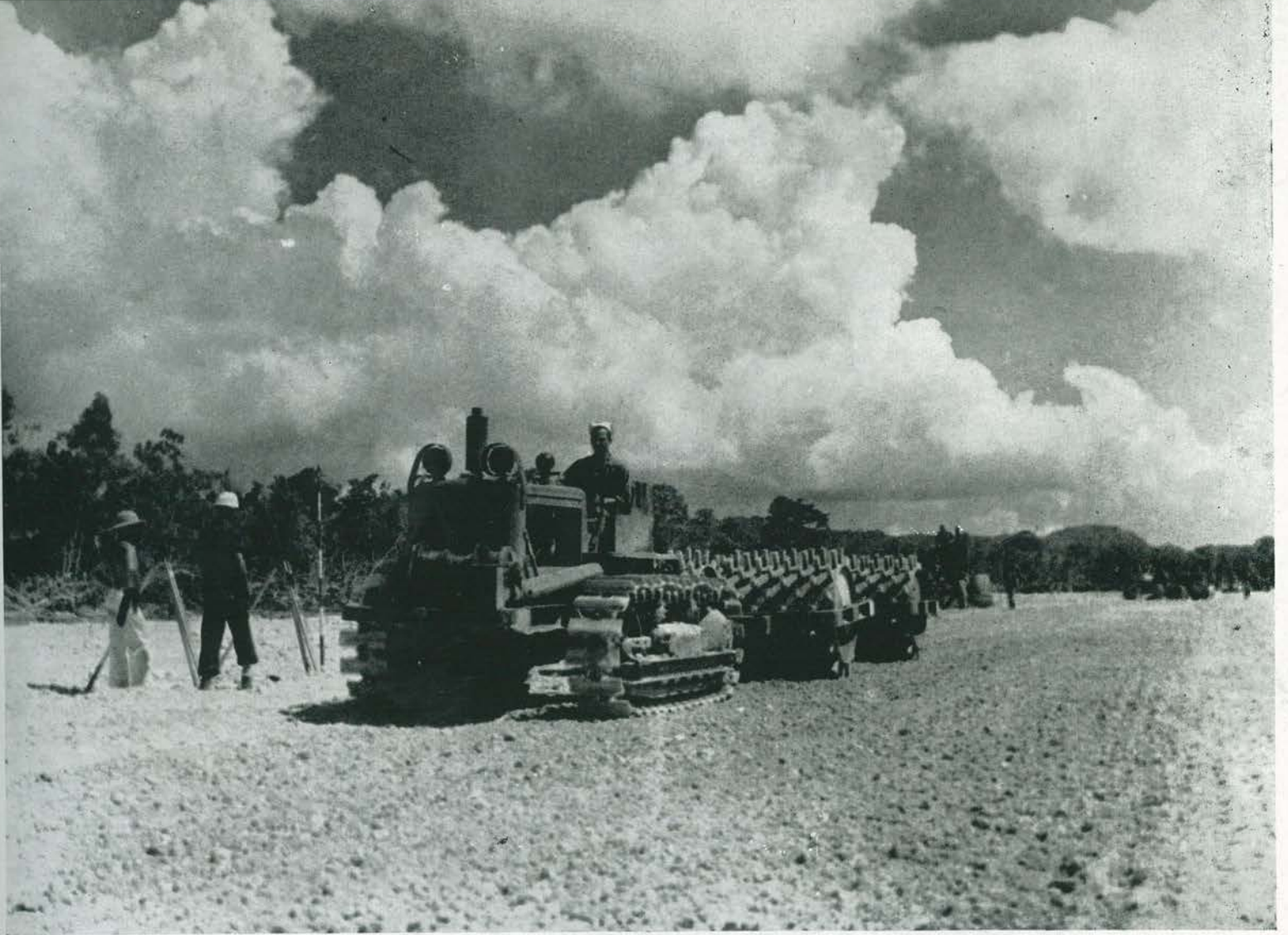
WALKING OUT. All fills were considered properly compacted when the sheepfoot roller "walked out." The sheepfoot also proved itself invaluable with its ability to spread large chunks of soft coral into smaller ones, thereby speeding up the operations immeasurably. Here, R. F. Johns is operating the sheepfoot rig. Surveyors Tom Campagna and Byron Chronic (with transit and levels) are setting blue tops. Grade Foreman Jim Bailey, (staff in hand, right) is supervising operations. Grader operator is C. J. Rominger.
