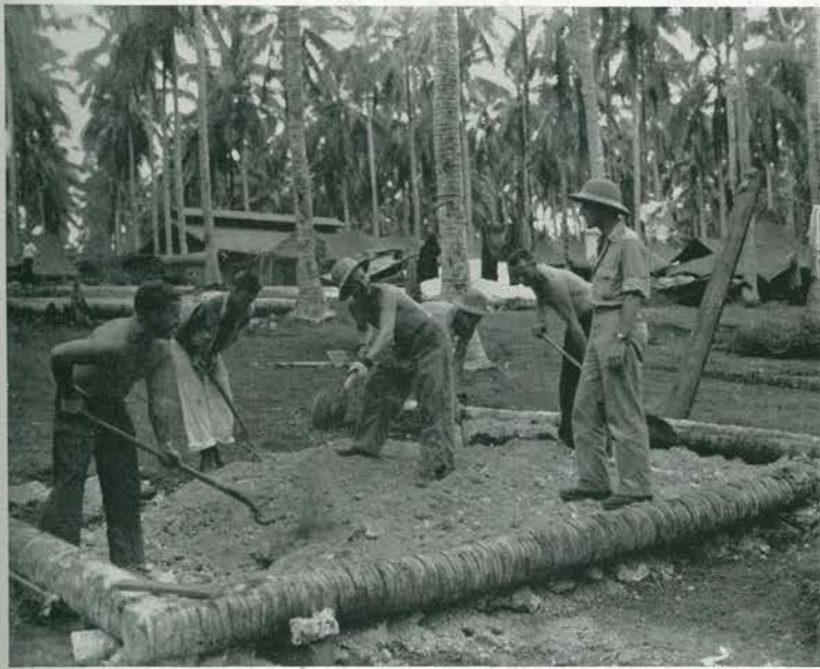
SHOVEL OPERATORS. To leave camp perfectly clean, "shovel operators" level off tent decks constructed of logs and coral. Left to right: Charlie Suojanen, Carl Knudsen, Lee Oakley, Robert Bowman, Alexander Cudney and Chaplain Ernest Marble.
