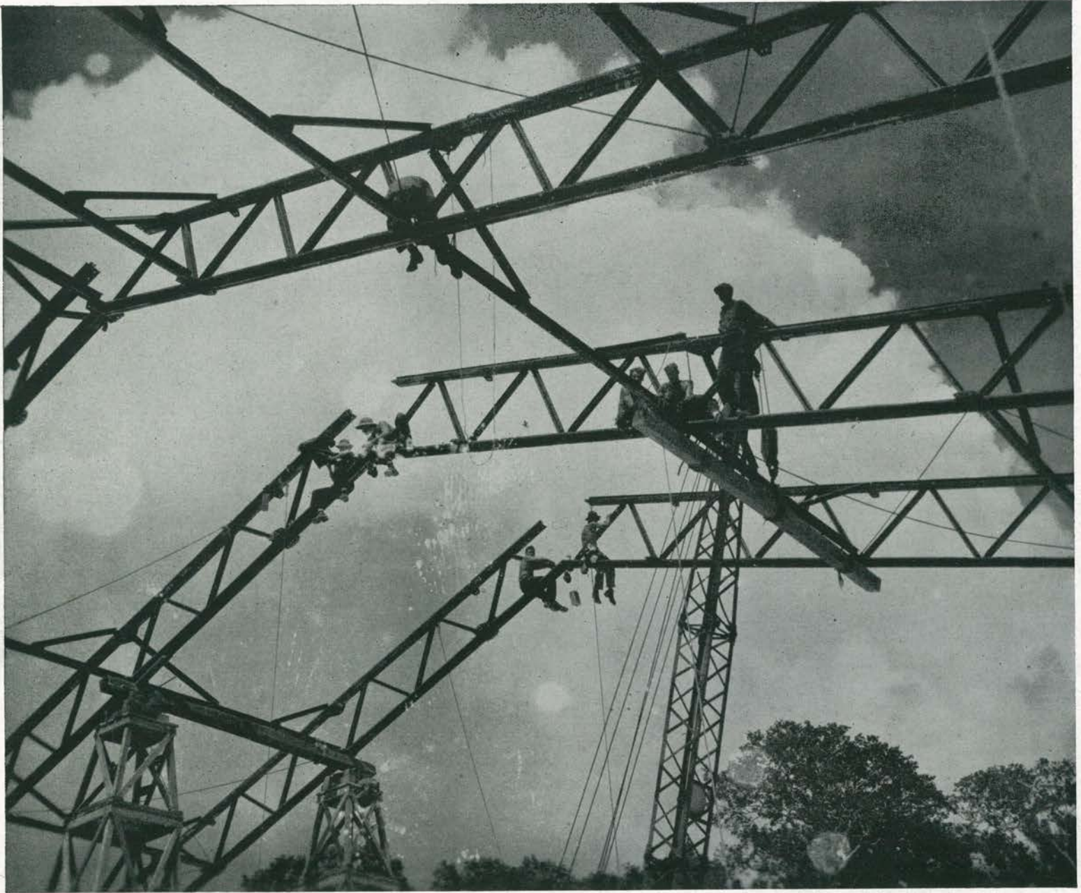
Eli Pifer took care of the delicate crane work. Chief Hugh MacDonald's carpenter crew provided the essential scaffolding and bracing. Structure was 120 feet wide, 160 feet long and 43 feet in height.
