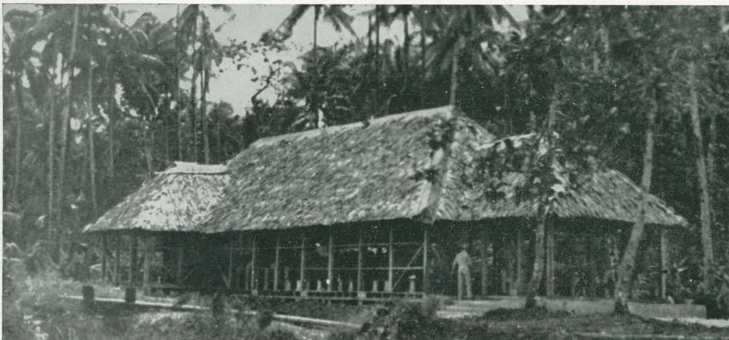
REPARATION. With peace eventually restored in the Treasuries, New Zealanders and Americans—as reparation for destroying the native church in exterminating the enemy—began building another church for their island friends. New edifice was erected on a beach in vicinity of former church site. Structure featured ornate windows
