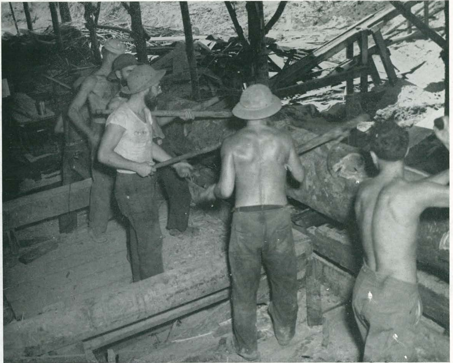
SWEATING IT OUT. Shirtless, bearded sawmill hands prepare a large native log for sawing into finished lumber for the innumerable top-priority jobs all over Mono and Stirling. Projects, it seemed to these men, could never be supplied with enough lumber to meet the ever-increasing
