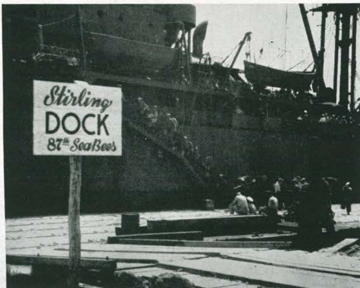
AND STILL THEY COME. Three CPOs sweat it out (seated on piling, right foreground) as endless lines continue up accommodation ladder. While the 87th builders are still given credit for Stirling Dock, gone forever is the famed sign, "What's Up, Dock?"
