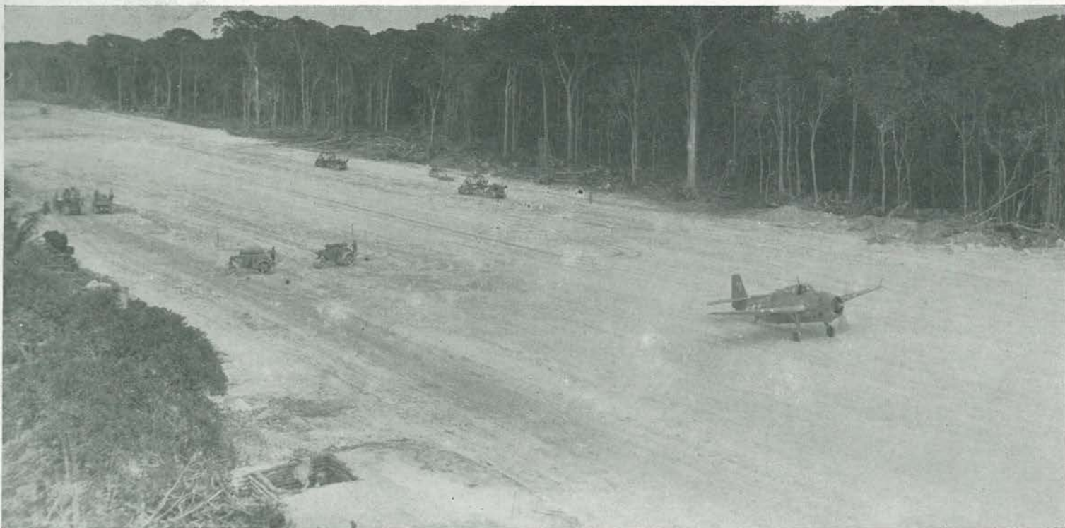
COMBINED OPERATIONS. Roller operators, forced off section of the Strip they were working on, watch as CASU 8 torpedo bomber takes off. Pans, working side sections, roll on undisturbed. Landings presented a somewhat greater hazard as the noise of diesels often prevented operators
