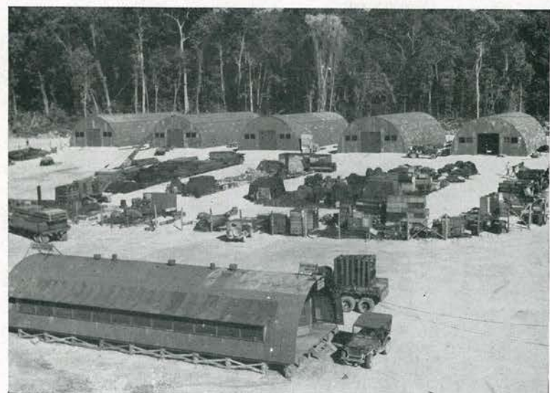
SUPPLY DEPOT , built in dock area, consisted of five 40x100 quonset warehouses and a compound surrounded by a barbed-wire fence. Office of Port Director was the 20x48 quonset (foreground). Area was once a Seabee baseball diamond
