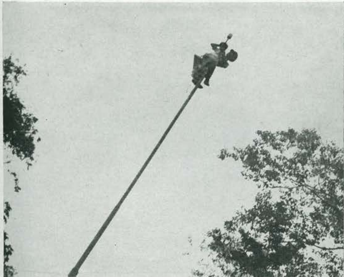
THE DARING YOUNG MAN. Chief Ted Marienthal inspects flagpole he and crew erected in front of the mess hall. Having followed this work as a civilian, Marienthal was equally at ease aloft or on the ground. "Nothing to it, Mates!"
