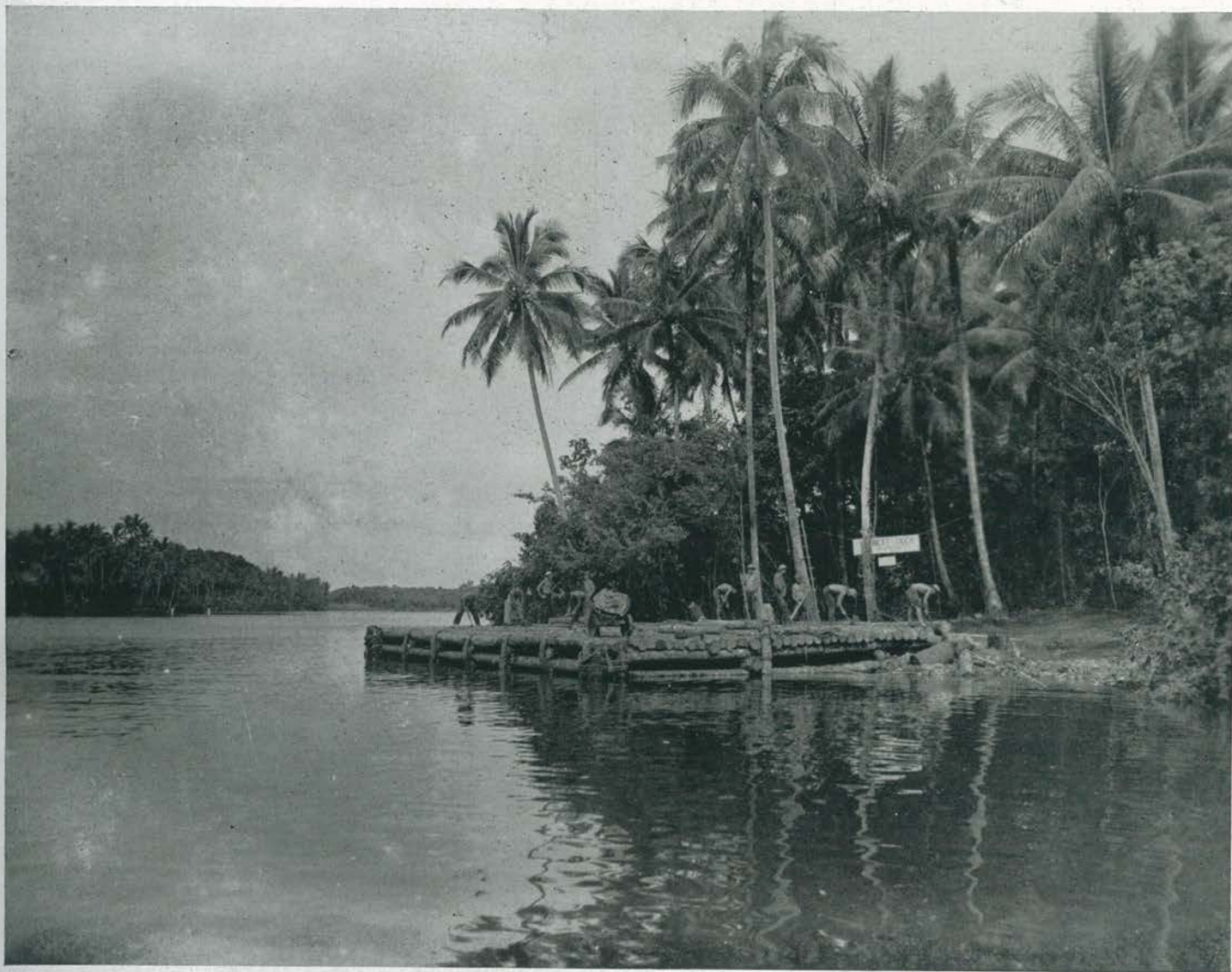
PT BASE. Torpedo dock for the cocky little night raiders was built by Chief Bill Inness and his Company A carpenter crew. Working long days with only hand-axes, this group completed the first Stirling project assigned the 87th in jig-time. Made of lashed coconut logs, the above crude struc-
