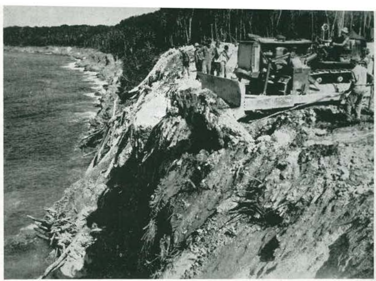
EASTY DOES IT, BOYS. The big rock is tottering, but Clyde Pemberton and his D-8 are precariously close to the crumbling edge of a 70-foot cliff. Lieut. L. D. Spaw, Jr., with his little stick, is delivering the necessary push.
