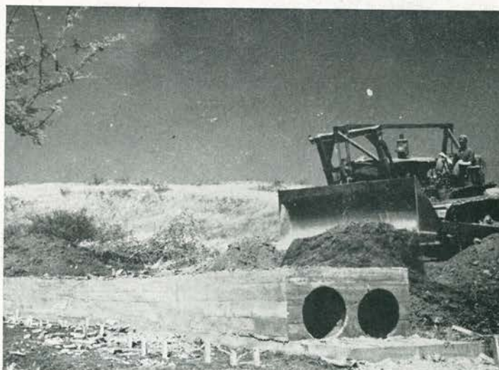
OVER THE TOP! Once the concrete had sufficiently hardened, wooden forms were stripped off and the indispensable bulldozers bladed tons of earth over the drains to bring spot to road level. Grady Thompson (at controls) shows how it's done.
