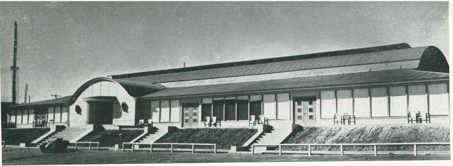
NRS OFFICERS CLUB. A plywood entrance, screened terrace, a few ship's lanterns—and presto!!!—the once lowly quonset acquires the regal lines of a modern night club. Designed and supervised by Lt. Comdr. Flynn, it
