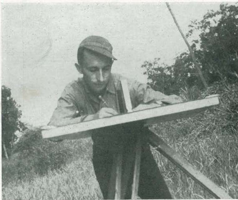
TOPOGRAPHER. Jean Worley of Lincoln, Nebraska, pores over his plane table to plot the topography of one of the multiple bridge sites and culverts, which were built along 13-mile stretch. Worley sports typical cap worn by most Seabees overseas.
