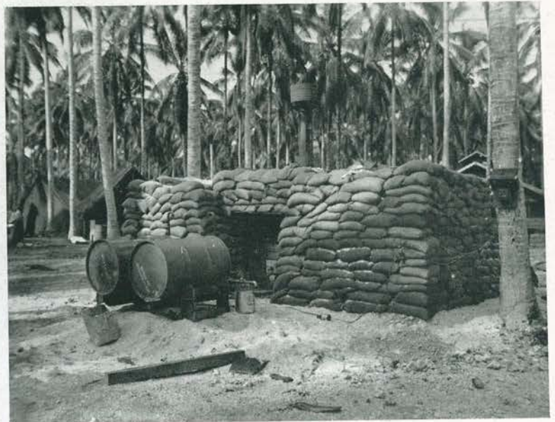
OUTDOOR OVEN. The finished oven is well insulated with sandbags to maintain the high temperature necessary in good baking. Despite its unusual appearance, the oven successfully provided the always hungry 87th with all-essential bread and cake.
