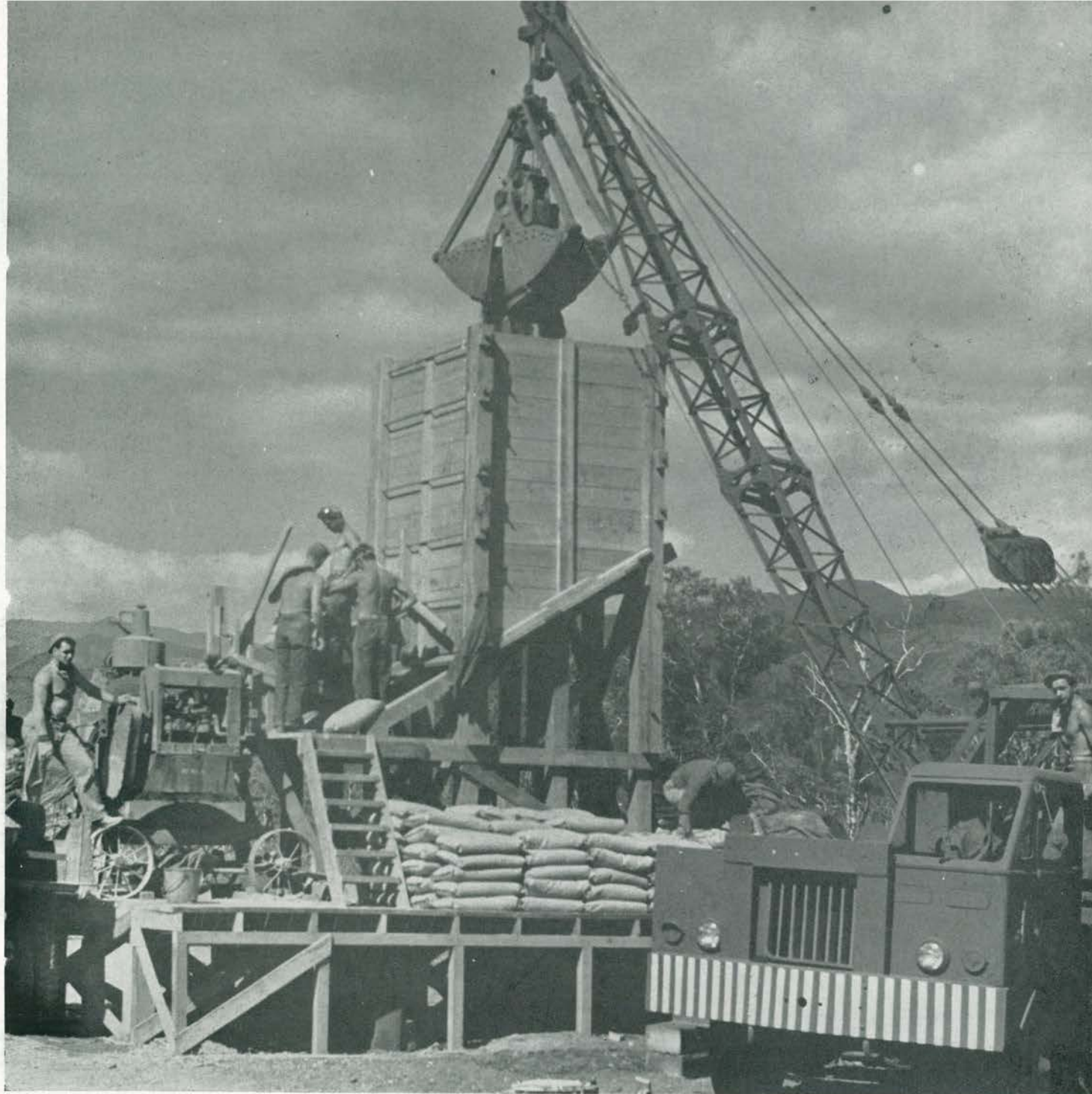
MACHINE AGE. In order to speed the distribution of mixed concrete, a mixing plant was centrally erected in the primary construction area. A clamshell rig was set up next to it. With this convenient arrangement, the aggregate was scraped directly into large, wooden hopper from
