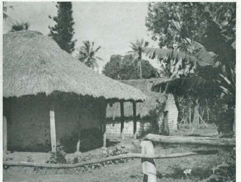
HOME, SWEET HOME. Besides providing an adequate shelter against the rain, straw-thatched roofs of native huts were a haven for rats, snakes and insects. Walls were mixture of clay and earth, but kept the temperature inside quite comfortable.
