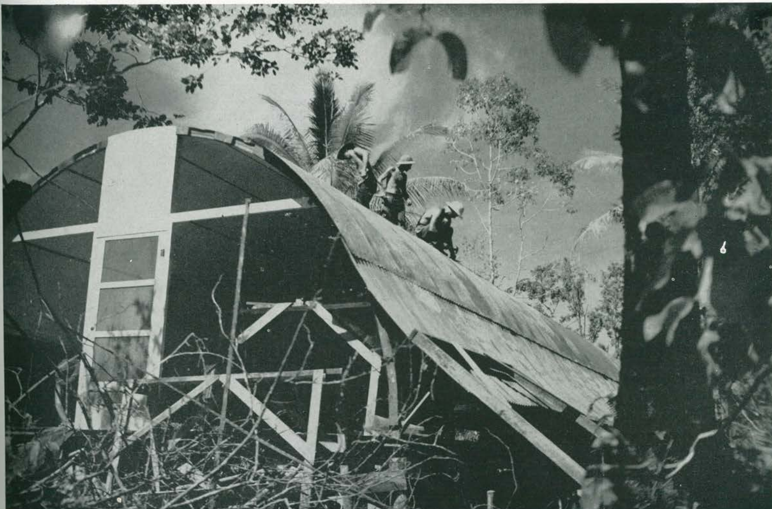
JUNGLE HOSPITAL. The first quonset hut erected on GOODTIME nears completion as a few carpenters work aloft while others finish inside trim. A group of these huts—eventually manned by medical officers and corpsmen—served as an emergency hospital for all air strip personnel. Airfield
