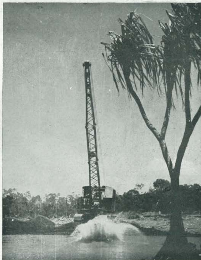
SPLASH. Final gravel-topping for completed stretches of new road was scooped out of handy stream bottoms with the dragline. Splash resulting from this operation was fodder for visiting picture book cameraman. Semi-tropical tree adds class to shot.
