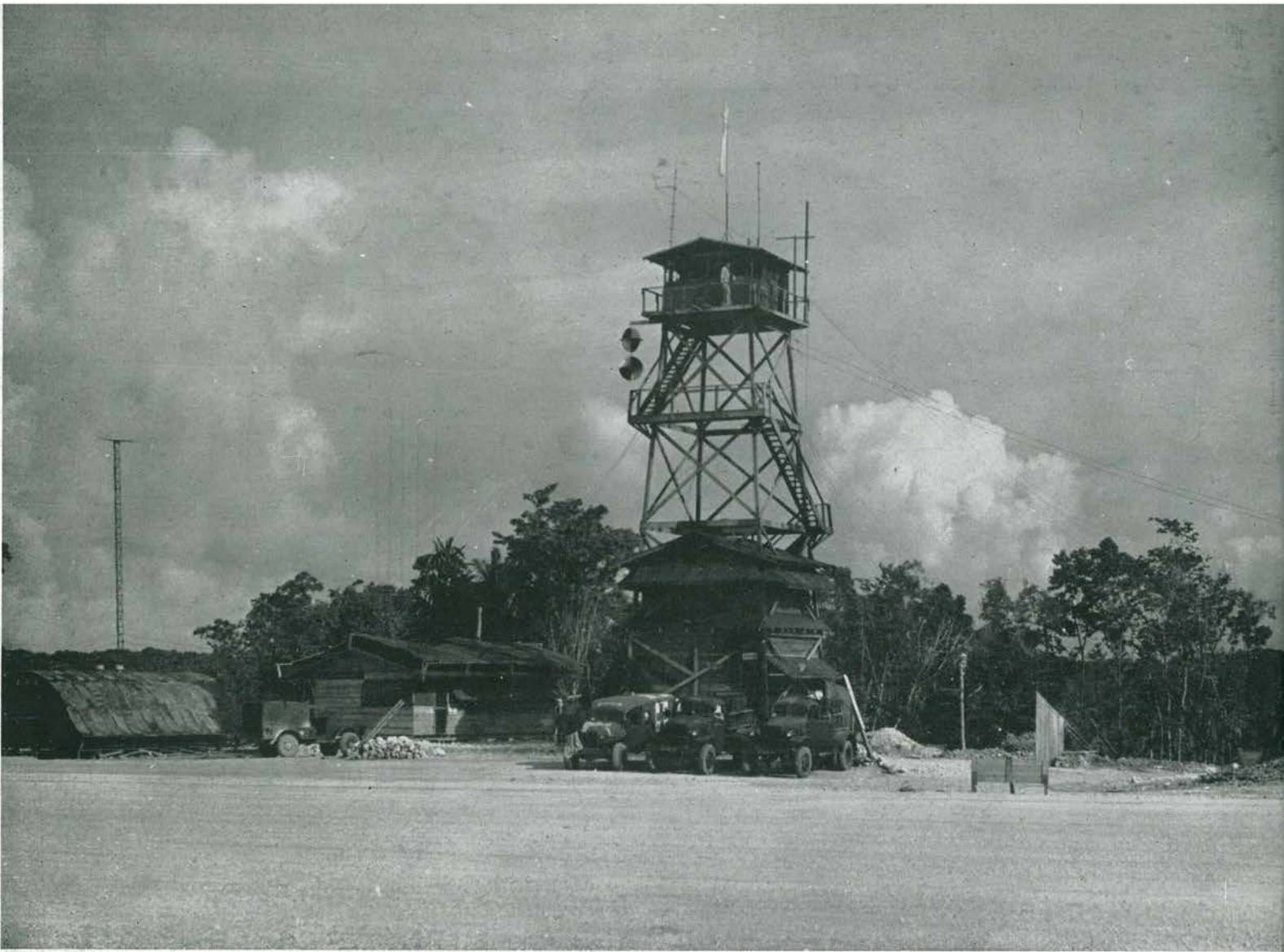
CENTER OF OPERATIONS. Not only did the Earthmovers build a strip on Stirling, but they constructed aviation facilities to go with it like this 60-foot control tower and the communications and weather huts shown here. Equipped with sizeable bolts and timbers,
