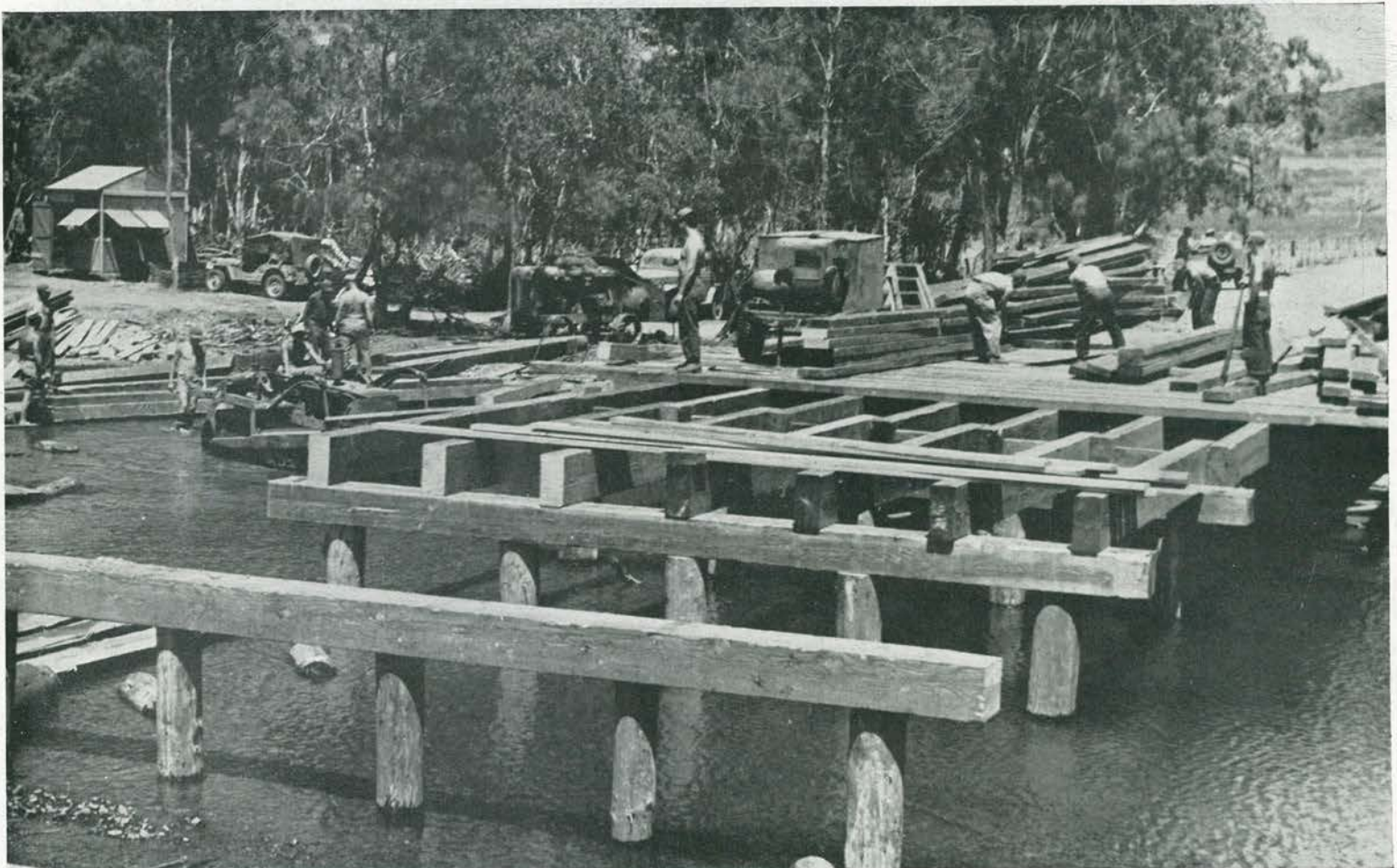
SKELETON CROSSING. Largest bridge of the project was the one across Frenchman's Creek in the long valley between Poya and Point Nepui. Utilizing a total of 55 piles, this sturdy bridge was 110 feet in length and 22 feet in width. Heavy 16x16 stringers (tying in the piles) were, in turn,
