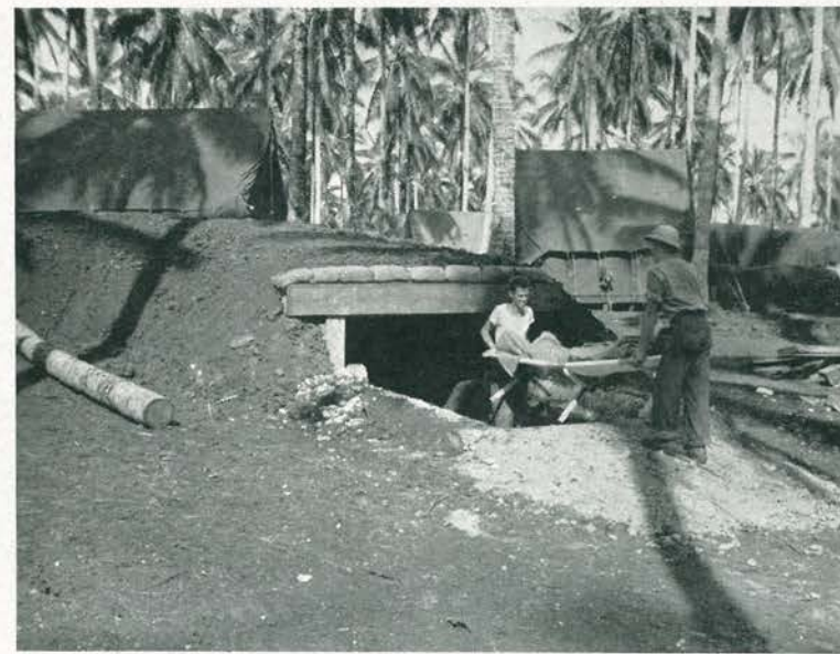
ALL CLEAR. Pharmacist Mates Fred Colby and Gaylord Hold remove a "patient," Archie ("Red") Reynolds, from roomy Sick Bay dugout after a simulated air alert. This sturdy shelter, built to accommodate 16 beds, was reinforced by heavy timbers and sandbags.
