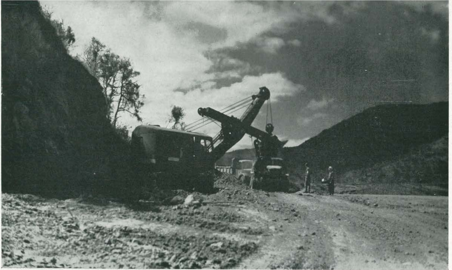
FACE LIFTING. The big Northwest shovel was kept busy tearing out huge chunks of the mountainside, which bordered the road project. Transporting the above monster and other heavy equipment the 133 miles between Monte D'Or and the Bourail location presented a major traffic problem.
