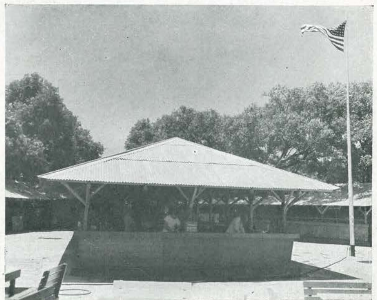
ALL SET to open next day (Thanksgiving), exterior of TRADE WINDS fountain was finished with stained plywood and a fireproof asbestos roof. Once opened, its 175-foot bar was never without several hundred parched servicemen.
