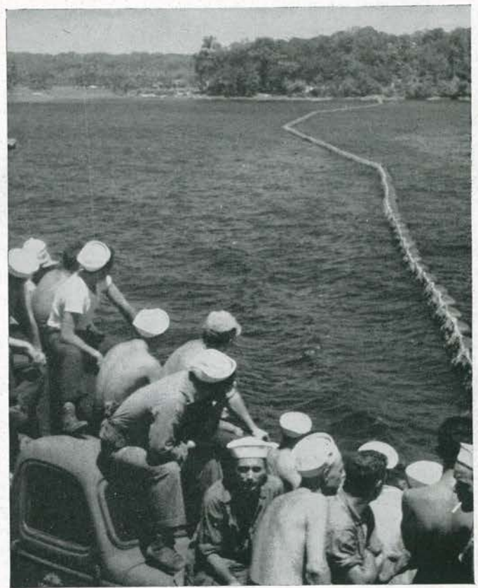
SUB NET, stretched from Stirling across to Mono, protected harbor and PT Base from enemy raiders. Seaplane tenders and PBYS, as well as sizeable warcraft, also found sanctuary inside its protective rim. Skillful navigation was required upon passing net opening.
