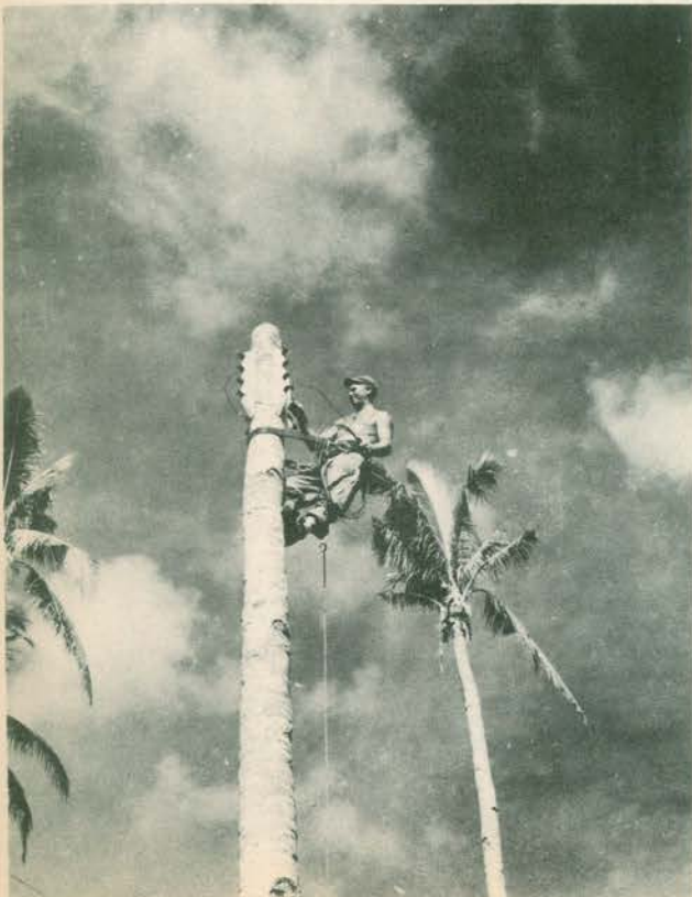
Stringing a Line
