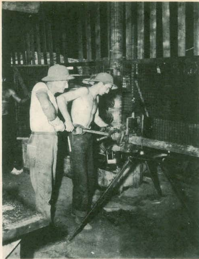
Threading Pipe
