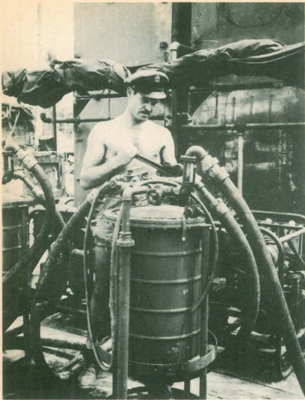
Assembling Water Purification Unit
