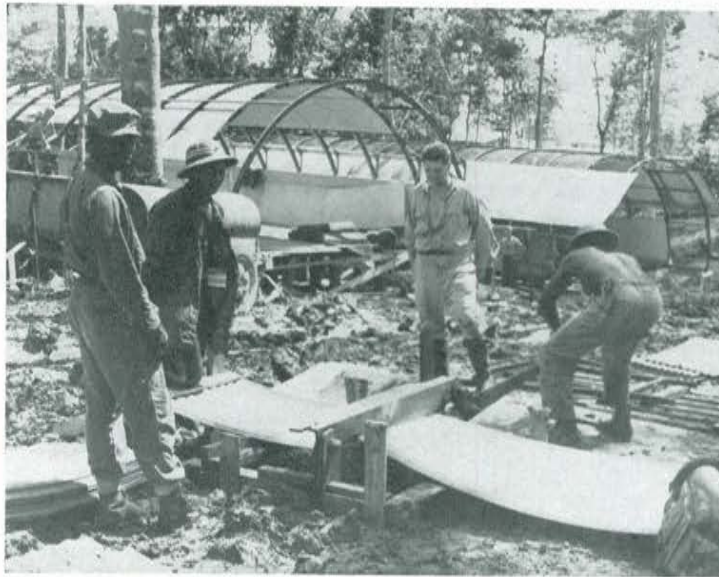
QUONSET HUT CONSTRUCTION
