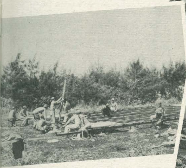
Construction begins on Saipan
