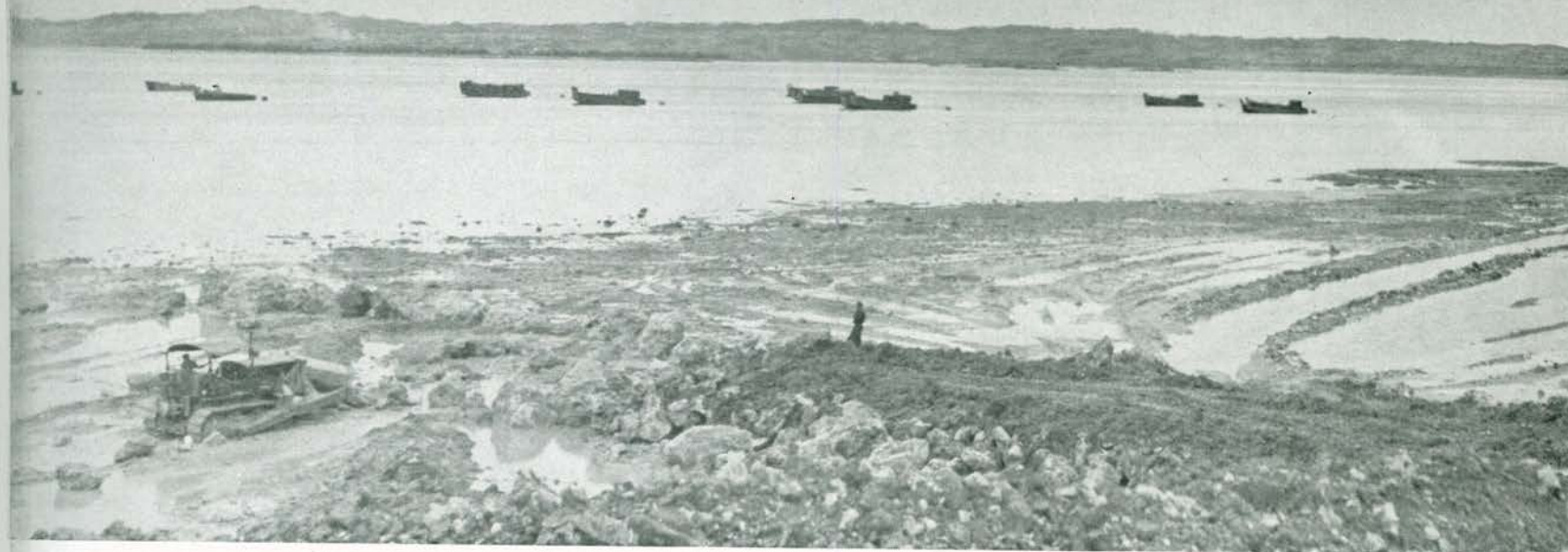
Fill material gradually formed an approach for the Section Base pier.
