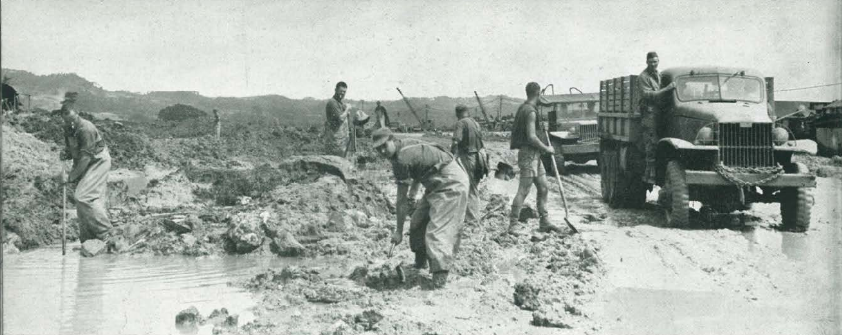
Three shifts shovelled to drain water and fill holes on the supply road to the front lines.
