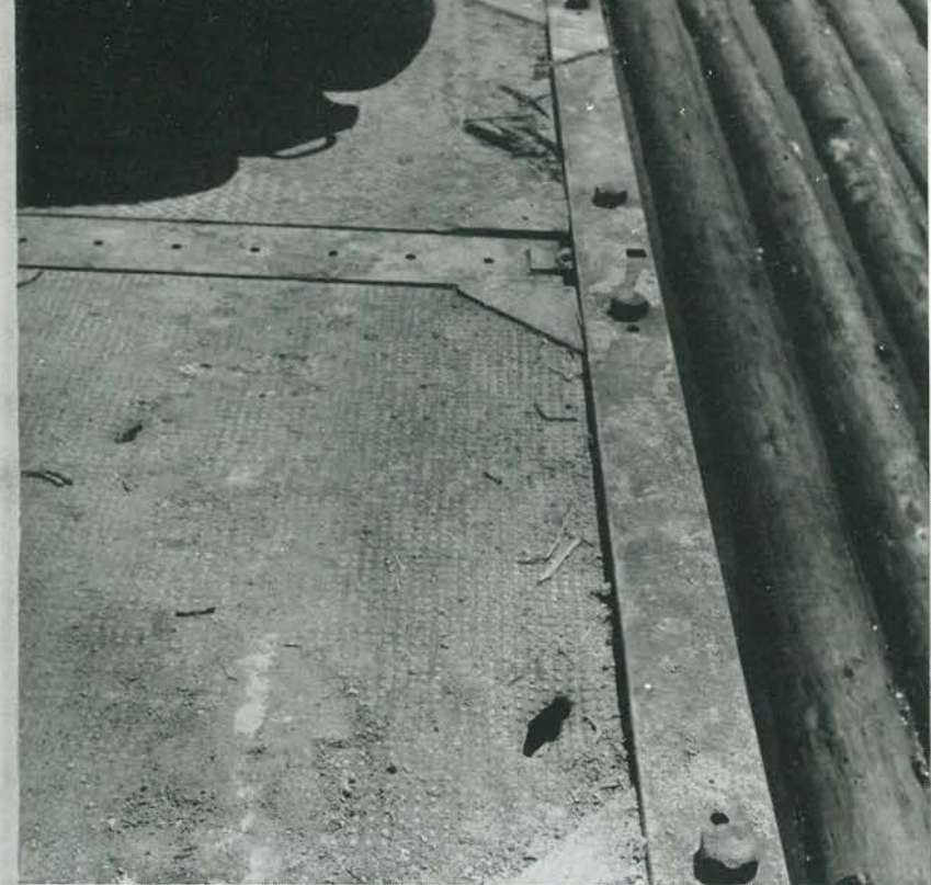
Shrapnel from a Jap bomb punctured pontoon cells on May 17
