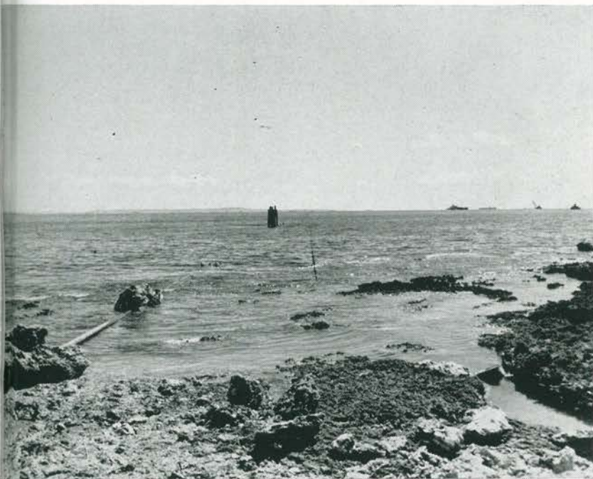
Dolphins were driven for sea-loading tanks
