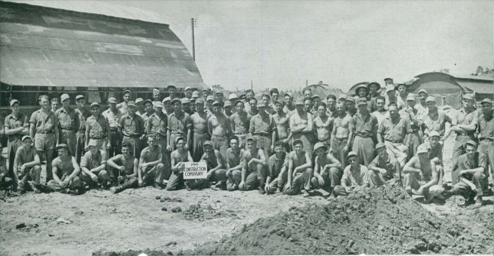
Top: Too few men could be spared from high-priority jobs for camp construction; the crews did a big job
