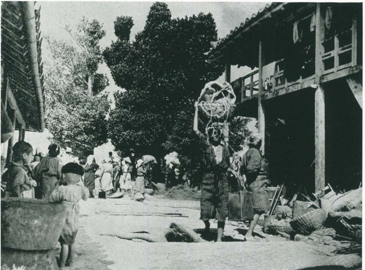
Top: Trees and walls protected the village homes from typhoon winds
