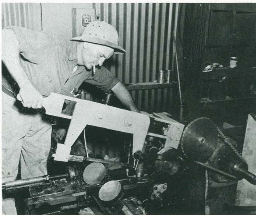
Above: Ingenious Swoboda also improvised a power hack-saw for some hard cutting.
