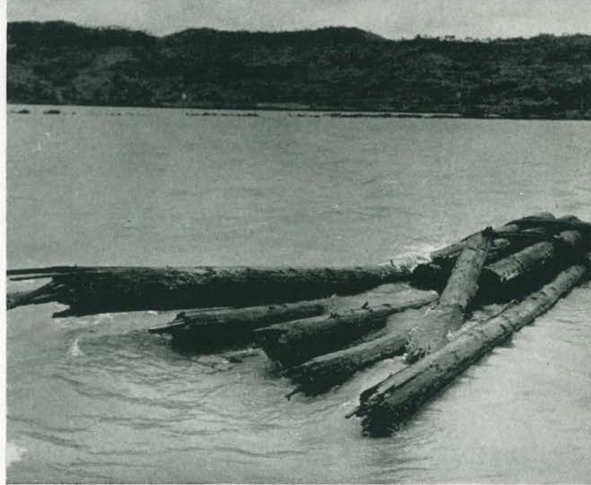
When an LST rammed the pier, it sheared off a dolphin
