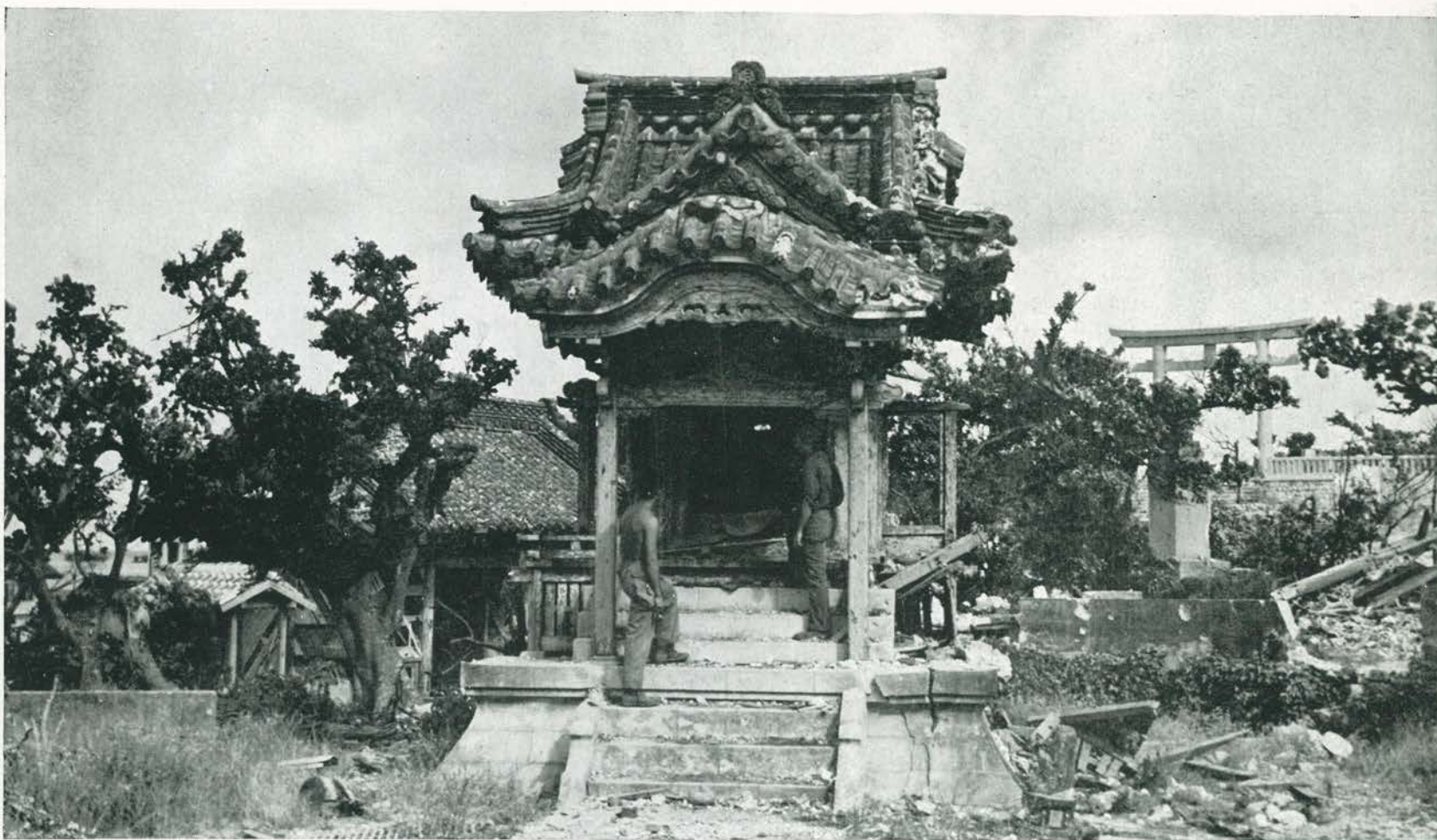
Top: Sandbags had not been much protection
