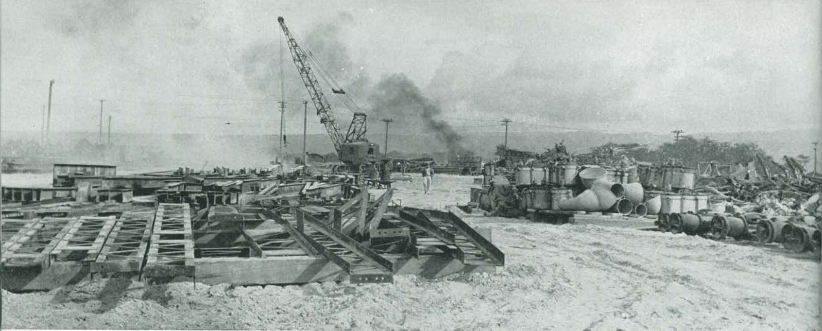
The damaged steel pieces had been stored in a muddled heap
