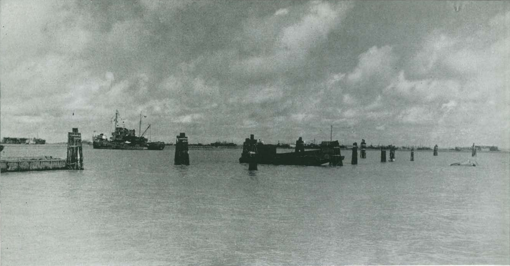
The Baten Ko pier was knocked out by the pounding. Later a part of it was reconstructed
