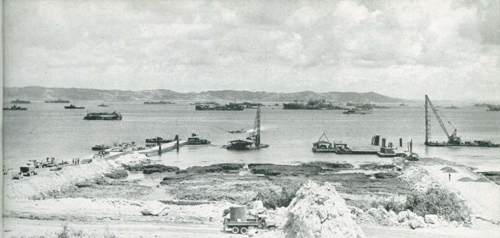
The approaches neared completion
