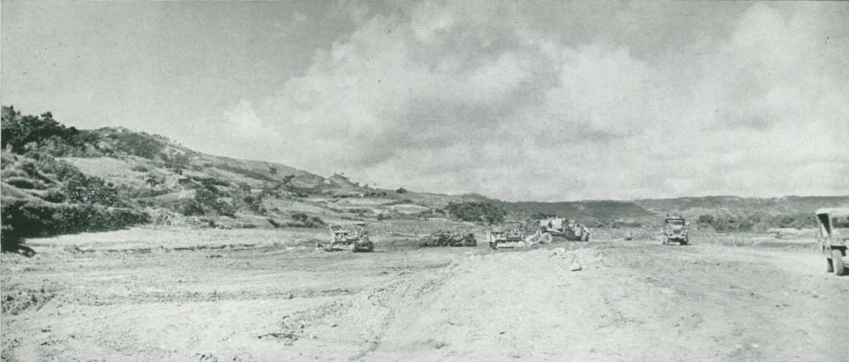
Heavy equipment widened the old Jap road along the south shore of Buckner Bay
