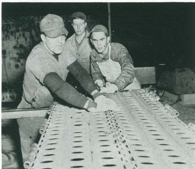
Above: Stephenson, Kelley and Ellis inserted hinge rods Below: Over 500 mat sections were completed
