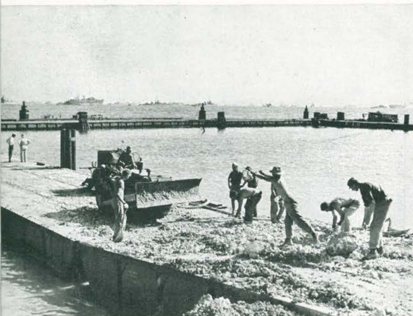
One tough problem was the fill where the coral rock, the pontoon and the sea water met
