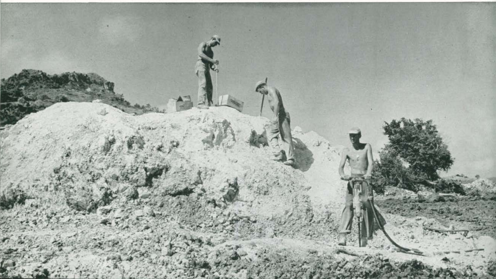
Macht, Horbach and Footer drilled holes for blasting away rock in the road right-of-way
