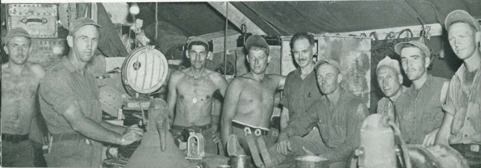
Below: Our electricians put in lines for needed power and light
