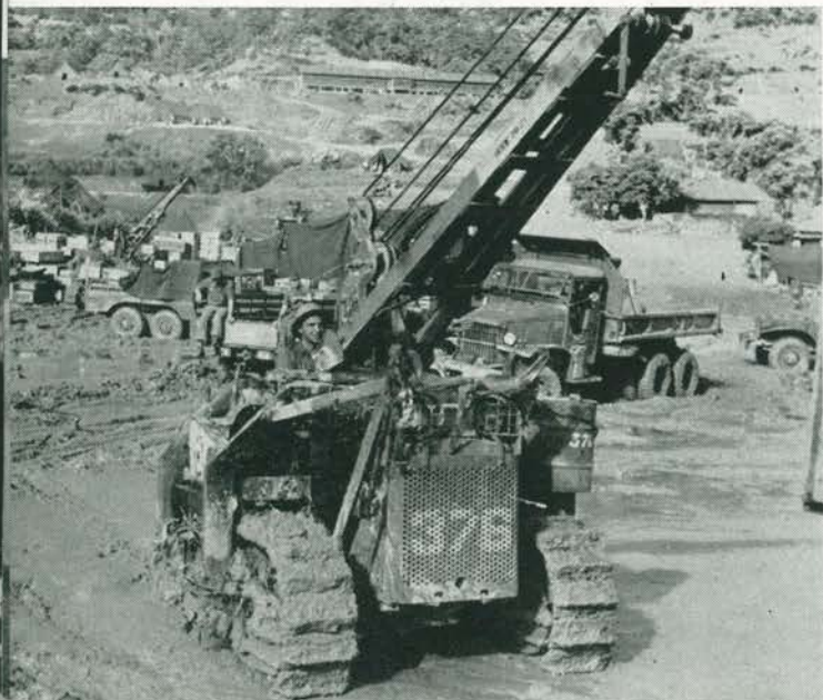
Cats and cranes handle heavy loads in the compounds and pulled trucks out of the mud.
