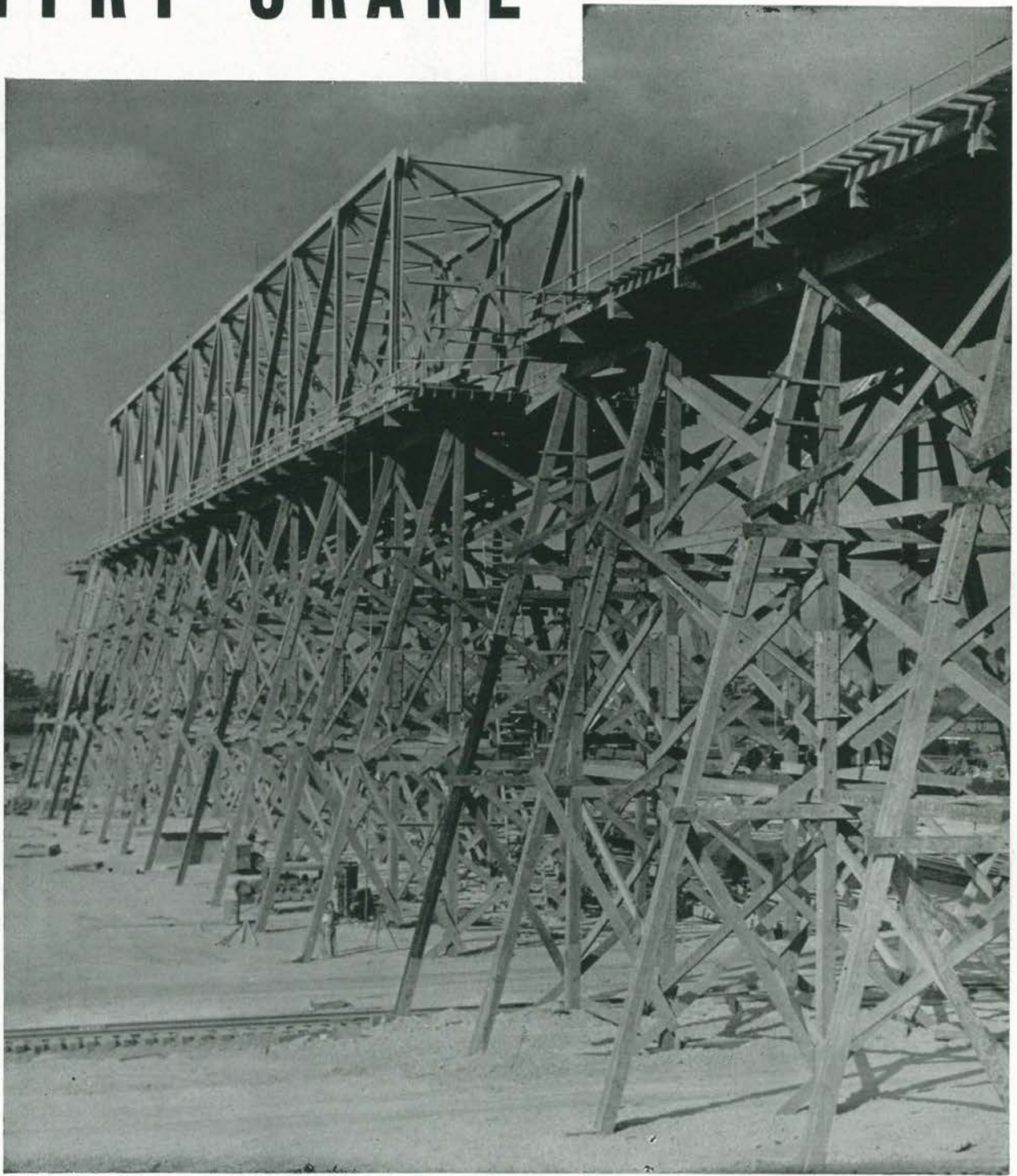
The gantry crane loomed high on the Pearl Harbor skyline
