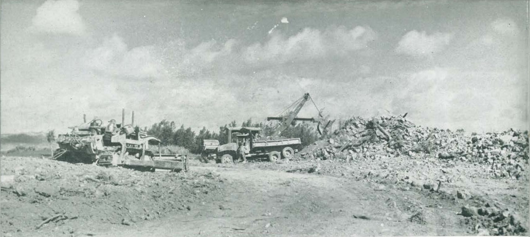
Rubble from ruined villages furnished fill for the pier approaches
