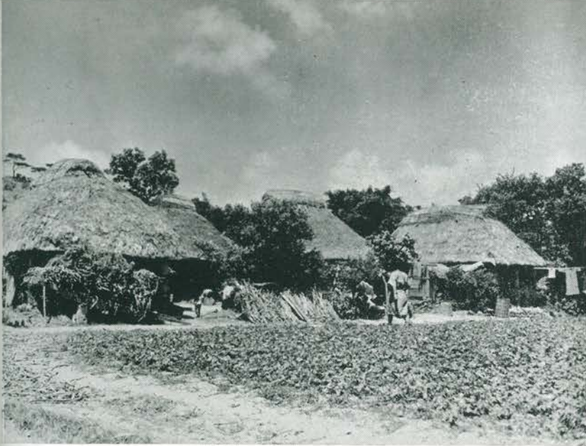
Very few homesteads escaped damage during the fighting
