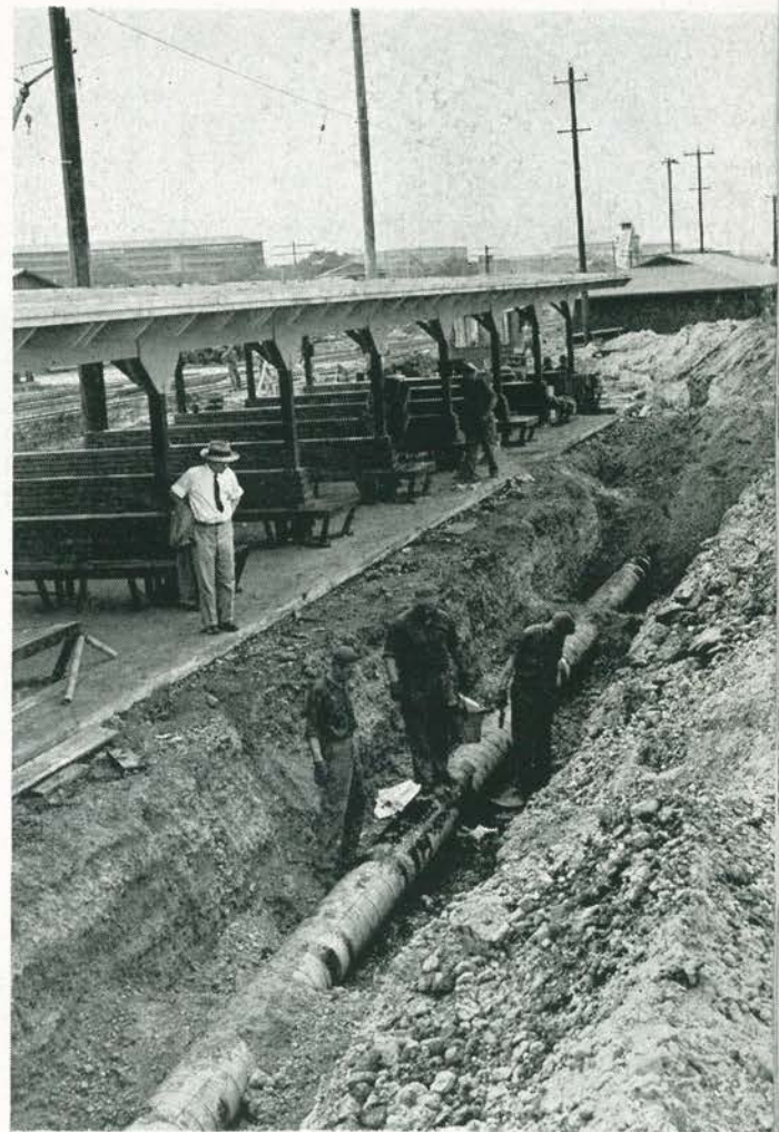
A BERTHING FOR FUEL BARGES was developed near Halawa stream. Old moorings were removed; nineteen dolphins were driven; a timber catwalk was built; pipe lines were laid; a machine shop, office, galley, and living quarters were erected. Soon Navy Yard oilers were using the berthing to supply the ships.
