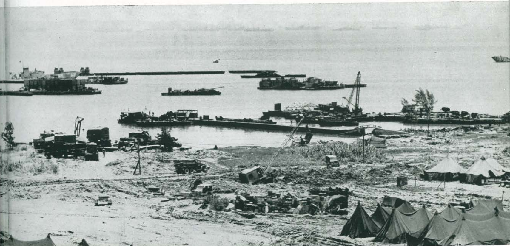
The docks of the pontoon assembly yard were surrounded by boats and barges
