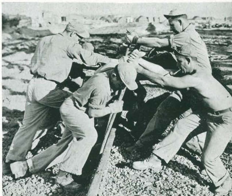
Below: "Elbow-grease" aligned the iron-rail runways Bottom: The runways were solid for 60-ton loads
