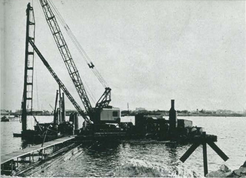
A BARGE SLIP was built at Iroquois Point to handle airplane-loaded barges. Aircraft were stored on a large field in this area. The slip helped to speed the transfer of the planes from ships to the field and from the field to the carriers.
