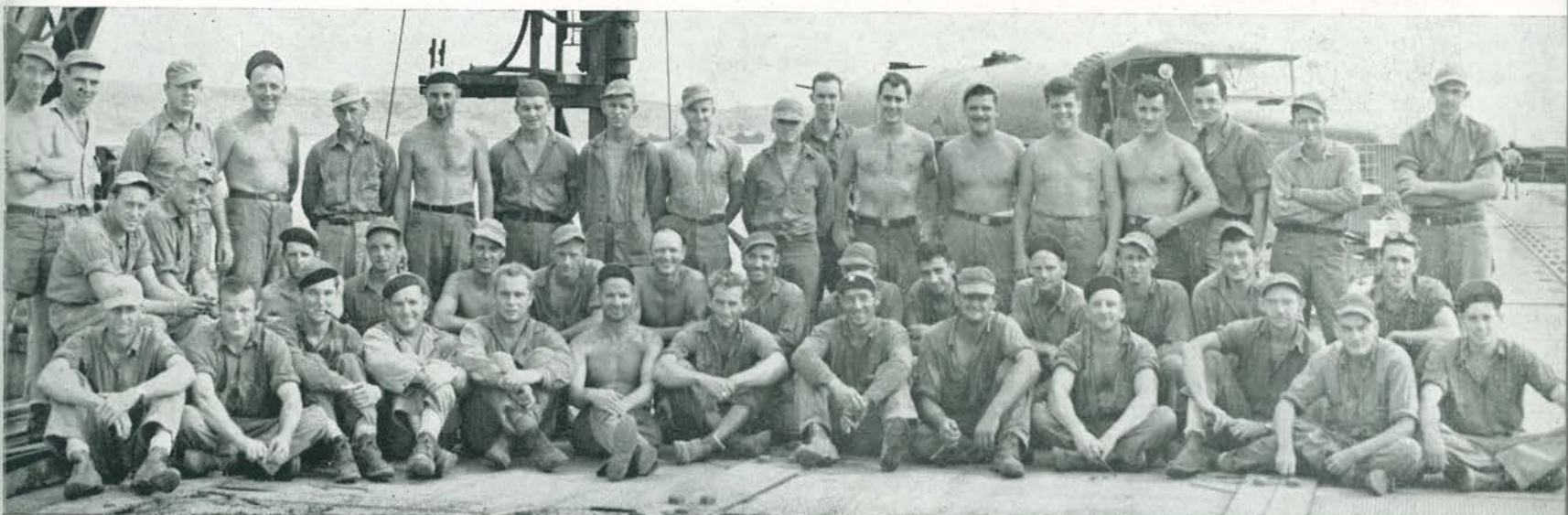
Part of the crew that built and maintained the Baten Ko pier
