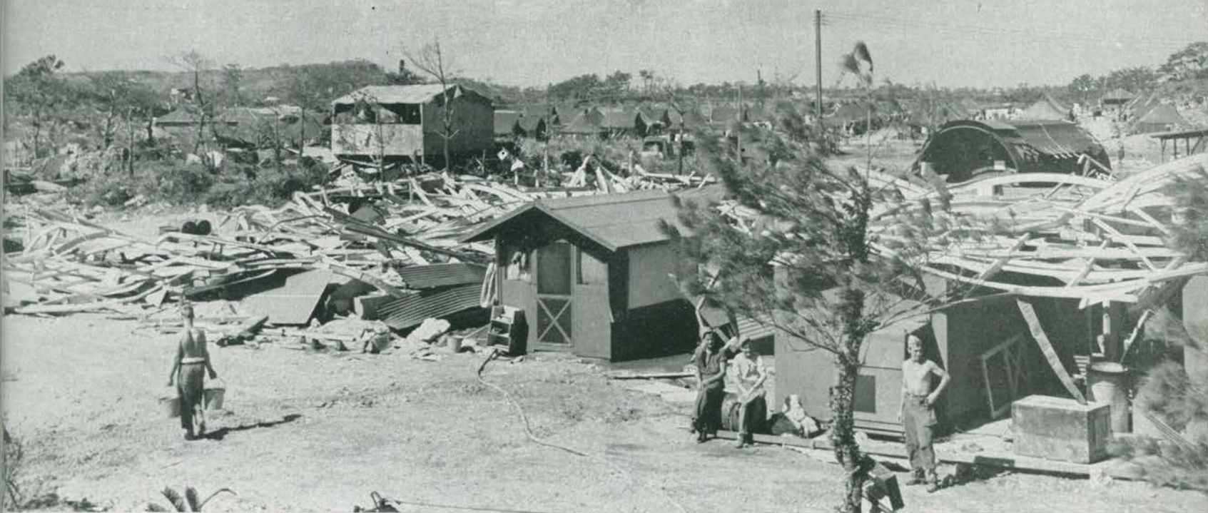
The pieces of the galley and mess hall—two large quonset huts—were peeled off like a head of lettuce; then the huts collapsed
