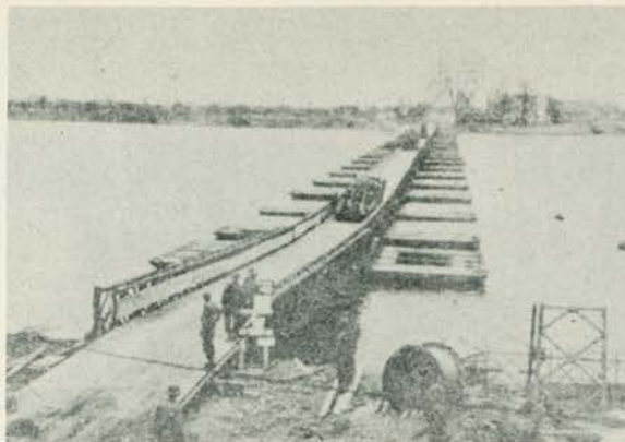
Bridge at Oppenheim
