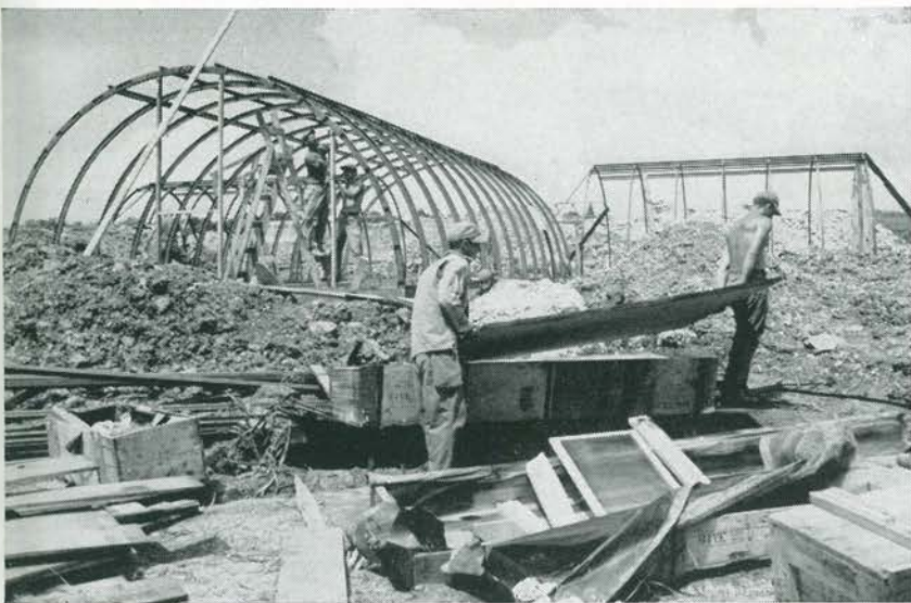
The unusual three-way quonset building was constructed by the 145th at Yontan airfield on Route No. 6. It was a joint communications building.
