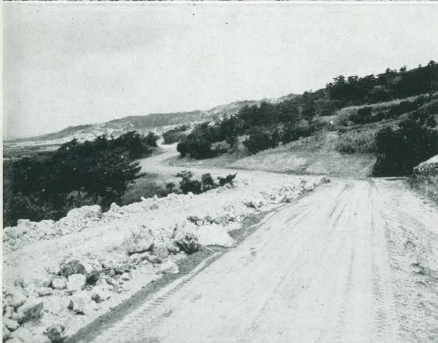
Shown here are six views of the Route No. 13 job which involved grading from Kuba Saki south along the Pacific coast side of Okinawa to Yonabaru airfield. Much of the road was relocated, and that portion from Route 32 junction south was coral-surfaced by the 145th.
