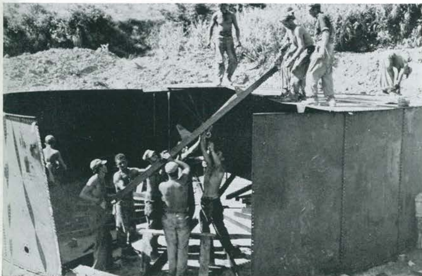
Here are three views of men of the 145th constructing a huge aviation gas tank farm near Yonabaru airfield. The twelve one-thousand barrel steel tanks were located about a mile north of the field and west of Route 13. Besides construction of the tanks, the job included the laying of two miles of four and six inch pipeline. The job was under supervision of Lt. Bentz, Lt. (jg) Redd, and Lt. (jg) Hewett.
