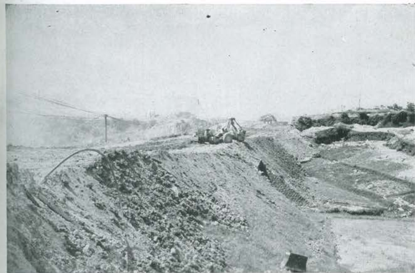
A broad, gleaming, coral-topped highway was the result of 145th labors on Route No. 1 south of Machinato toward Naha on the west side of Okinawa. Upper photo shows the finished product. The two lower photos are progress shots.
