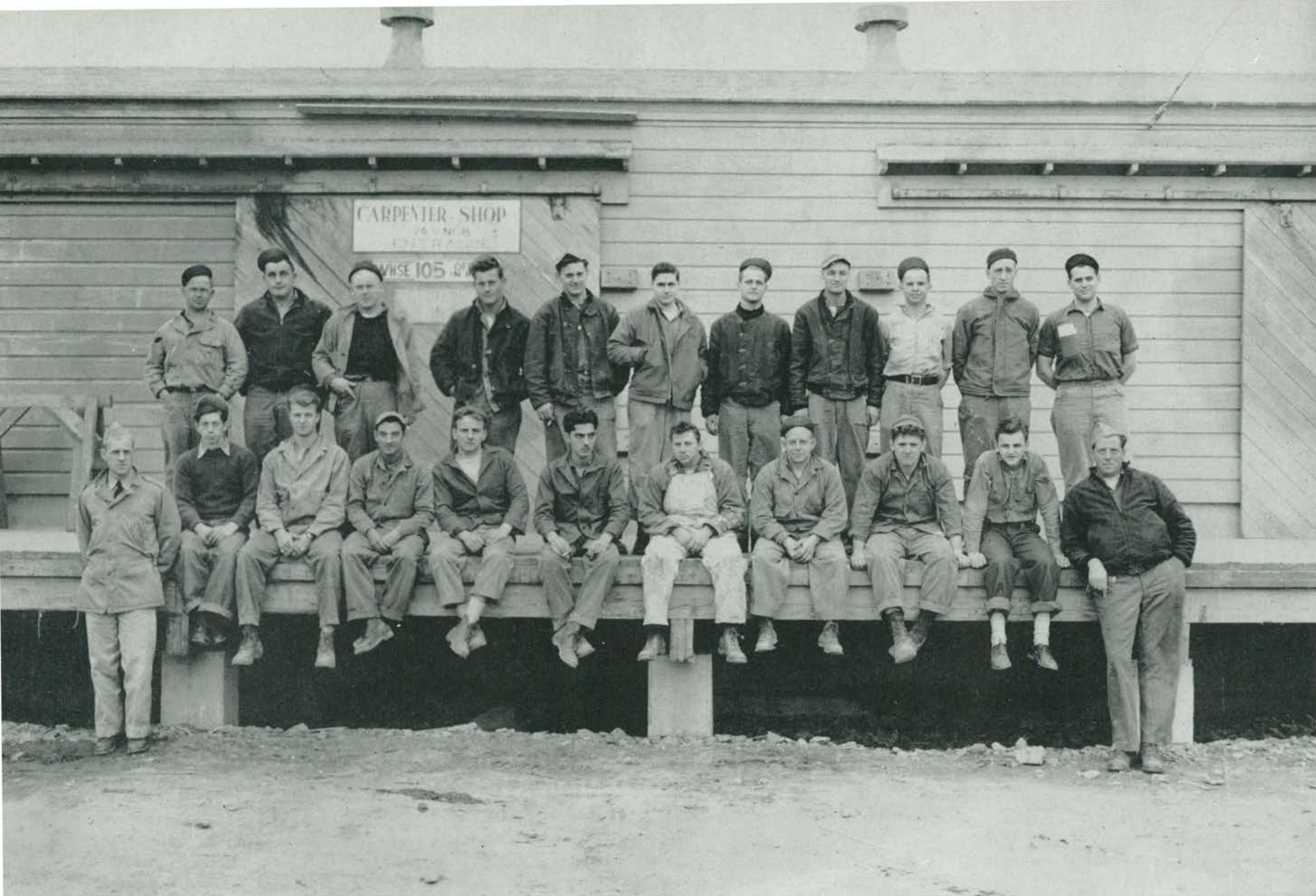
CARPENTER SHOP AND PAINT SHOP CREWS
