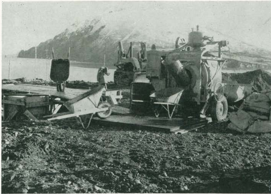
Pouring Foundation for East Tower
