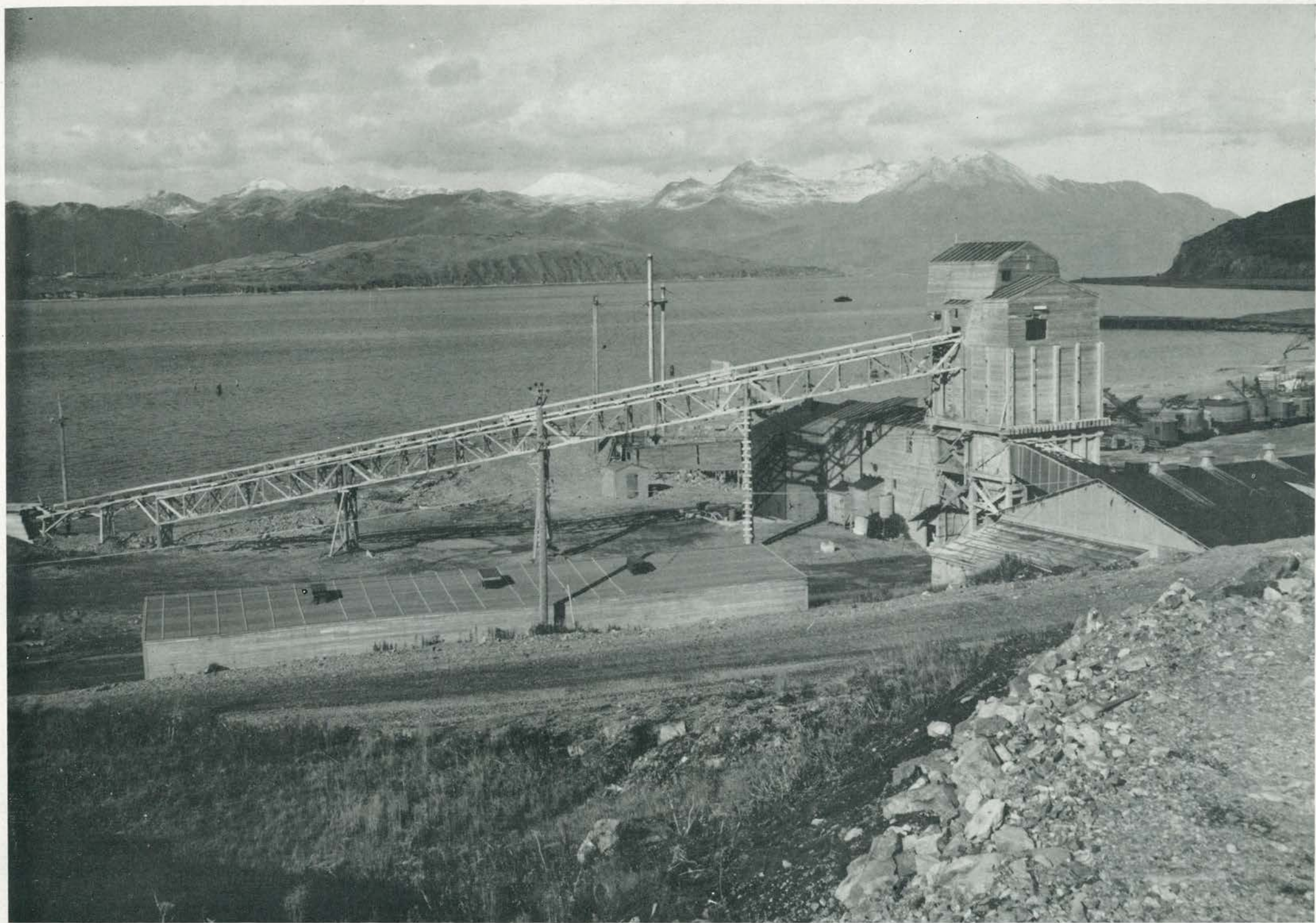
AGGREGATE PLANT WITH HOG ISLAND IN BACKGROUND
