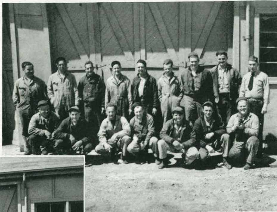
Road Maintenance of CB Shops Crew
