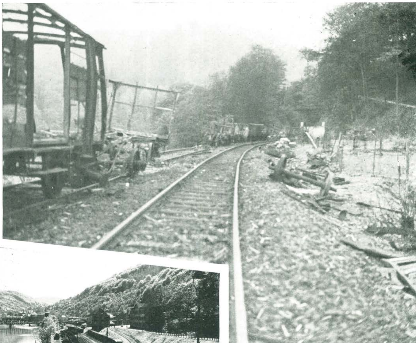
The remains of German munitions train which caught fire in tunnel are dragged out onto sidings to allow the passage to be cleared and repaired. Below German laborers lay rail on one of the very many rail bridges which had to be rebuilt to insure the carrying of material for the section reconstruction and rehabilitation of the area.
