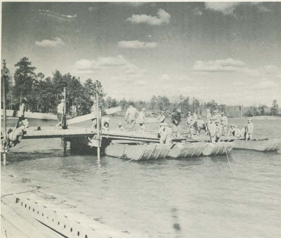
Ponton bridge construction at Birchen Lake
