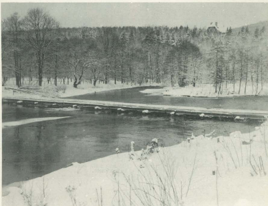
Snow-covered floating treadway bridge in the Ardennes.
