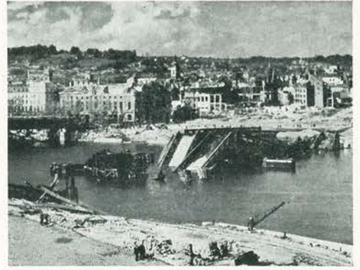
Bombed-out bridge, Rouen, France.
