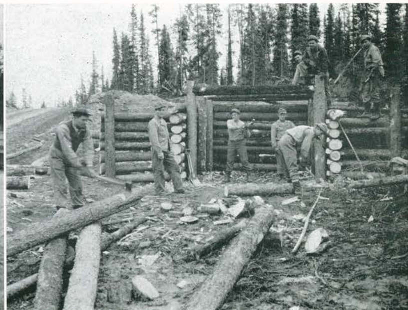
F Company builds a gravel bunker for road surfacing, mile 26.3.
