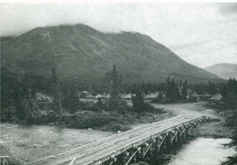
Takhini river bridge was built by Company D during the time they were isolated in this peaceful valley. Later Company F occupied the same camp.
