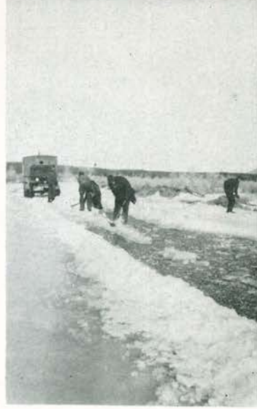
Chipping off a high center in the ice crossing at the Donjek.
