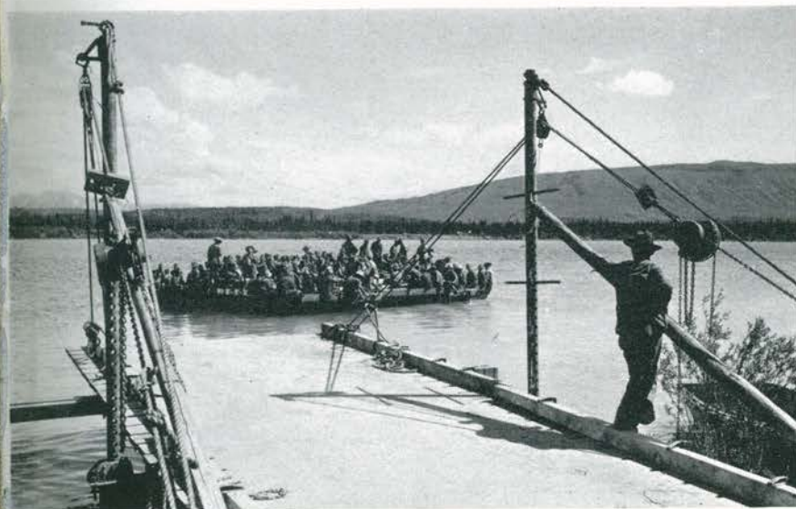
340th Engineer troops rest for a change and let out-board motors on the ponton ferry do the work of crossing the Tagish river.
