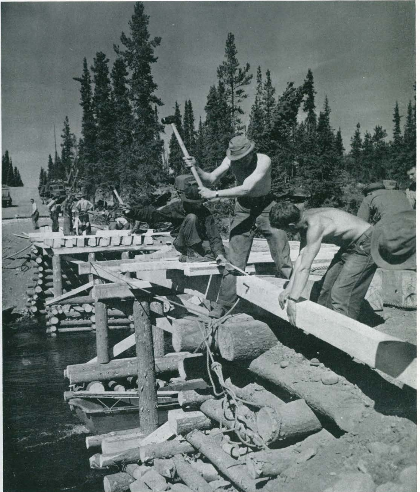
Multiple action nicely "frozen" is represented in this fine shot of the Morley River bridge under construction. Two newly completed sections of road will be joined by the bridge.
