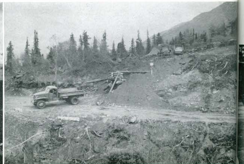
A gravel chute built into the sides of a deep valley. In this vicinity ground was swampy, full of boulders, and cut by deep gullies.
