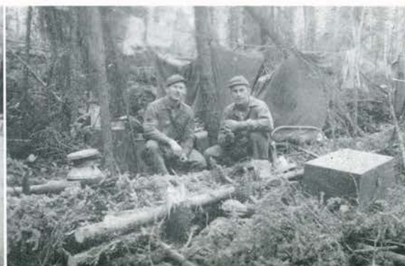
Late in June, 1943, C Company joined B Company just above Beaver Creek to work on the road.
