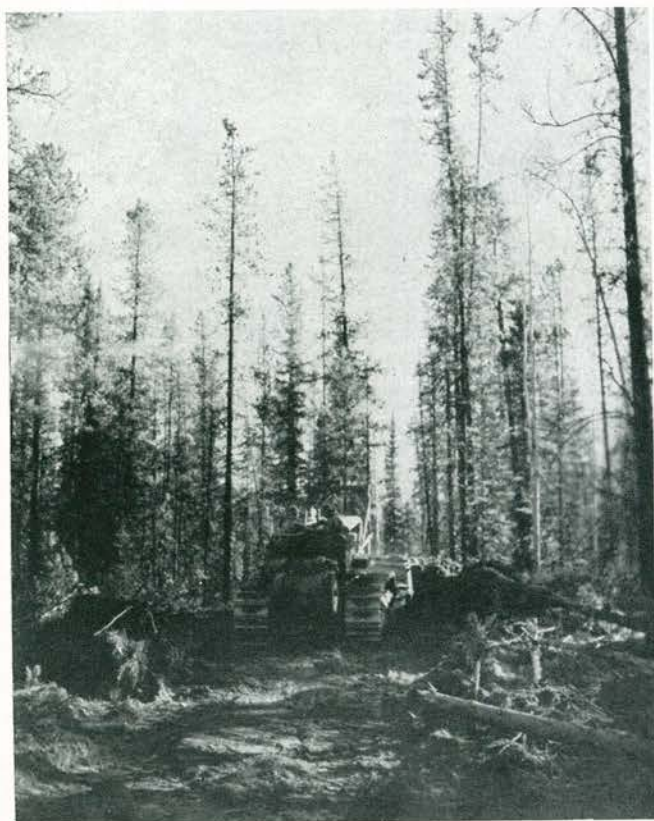
As the "cats" go, so goes the road. The leading D-8, E Company, plows through the forest.
