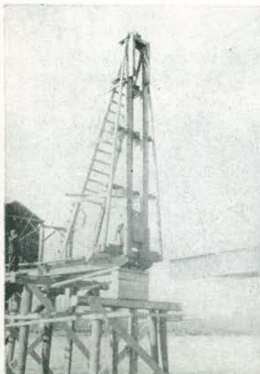
Pile driver hoisting a steel beam in the reconstruction of the Tanana bridge.
