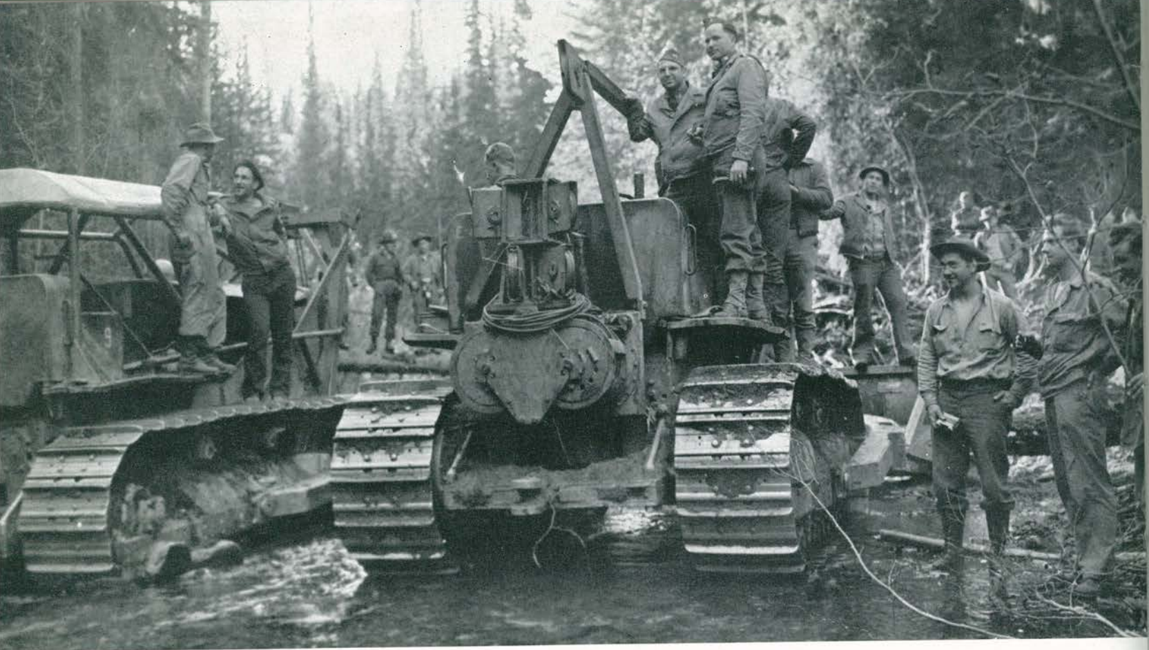
A big moment, long awaited, was the meeting of the "cats." The 340th, working south, and the 35th Engineer Regiment, coming north, met at Contact Creek, mile 219, on September 24, 1942.
