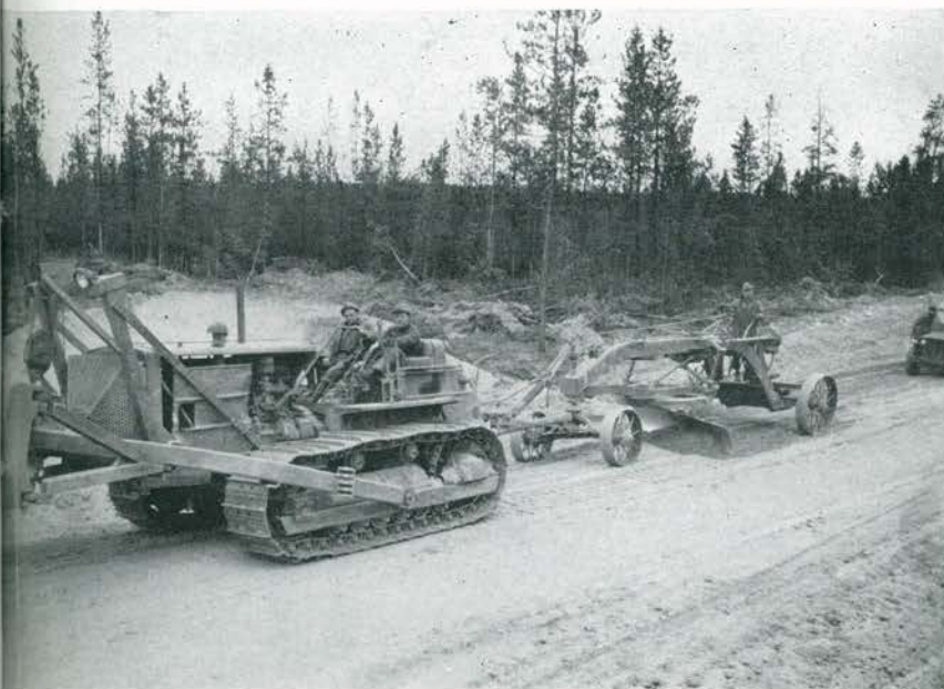
Grading the road at mile 157 are A Company men.
