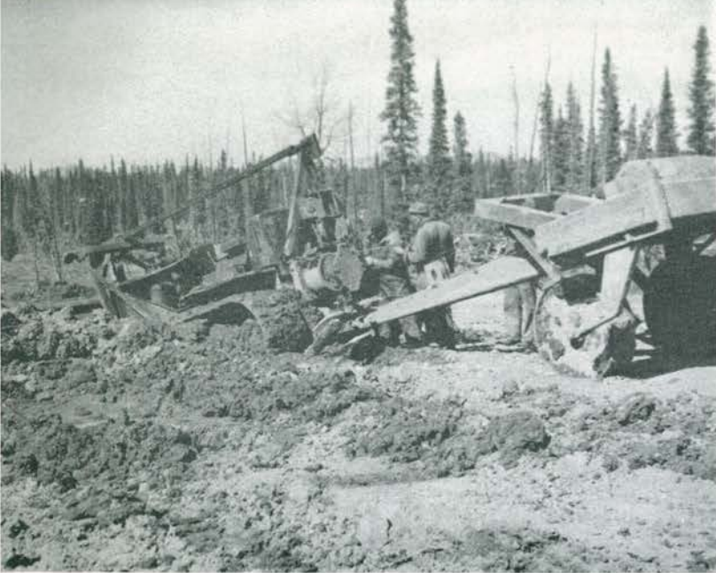
A Company F cat takes a nose-dive in the soft ground at mile 4.
