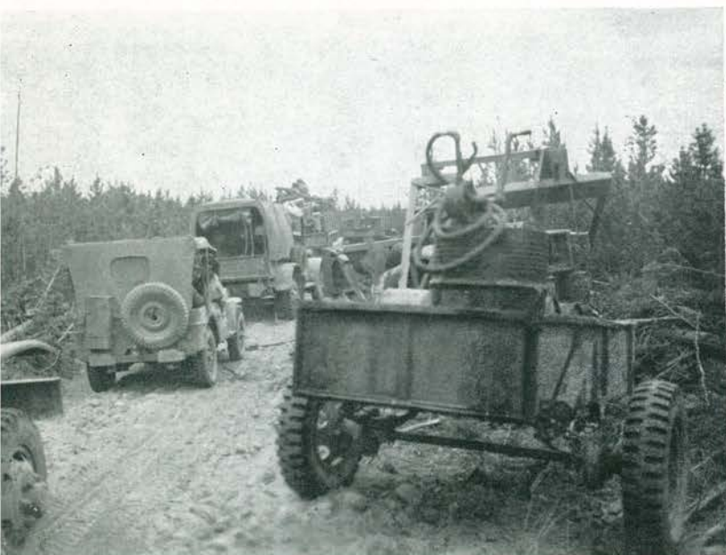
Moving day, with a typical convoy of men, trucks and equipment. The 340th goes on to another stretch of road building.
