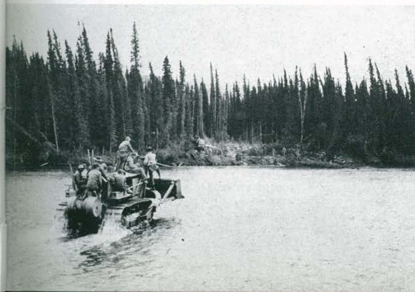
A little matter of lacking a bridge is no handicap to a D-8 cat. One fords the Rancheria river at mile 120.
