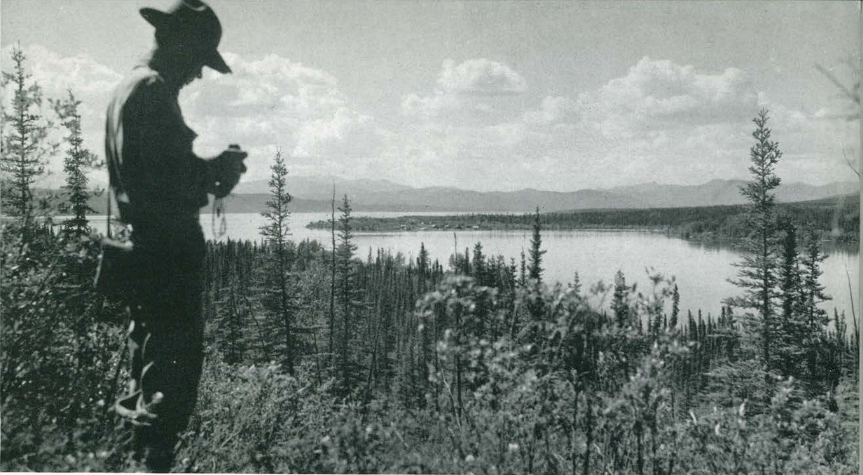
Nisutlin Bay—beginning of the 340th Engineers' 220-mile section of Alcan Highway construction. Mile 0.0. The village of Teslin appears in the background, across the bay.
