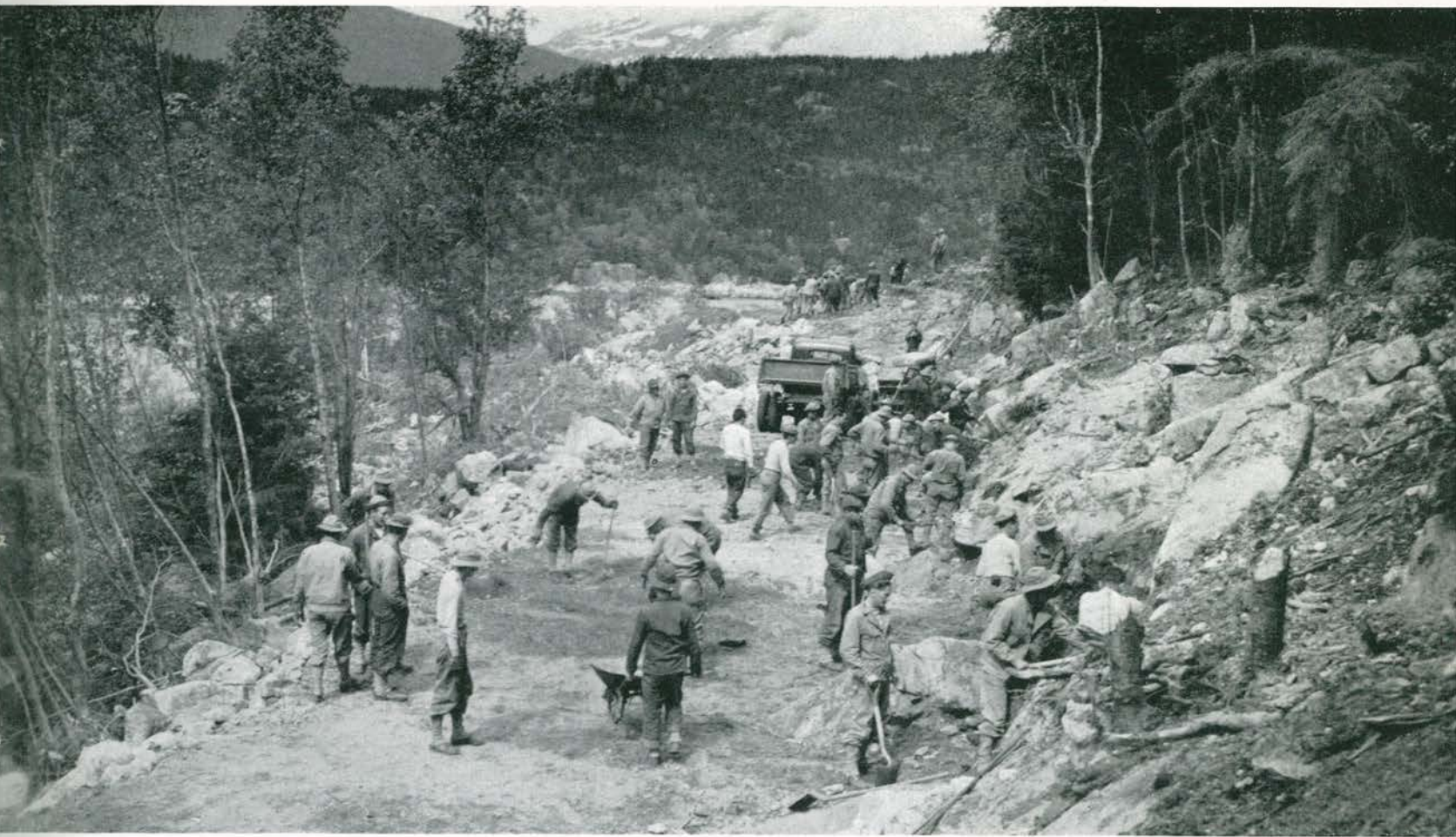
First Road Job—Skagway-Dyea—May, 1942.
