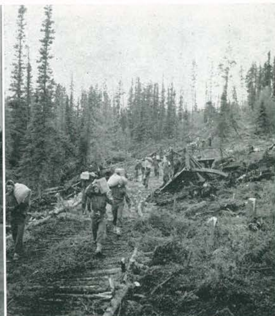
When trucks bog down and D-8's are practically buried in treacherous swampland, manpower comes to the rescue. Rations being "portaged" over a piece of corduroy trail.
