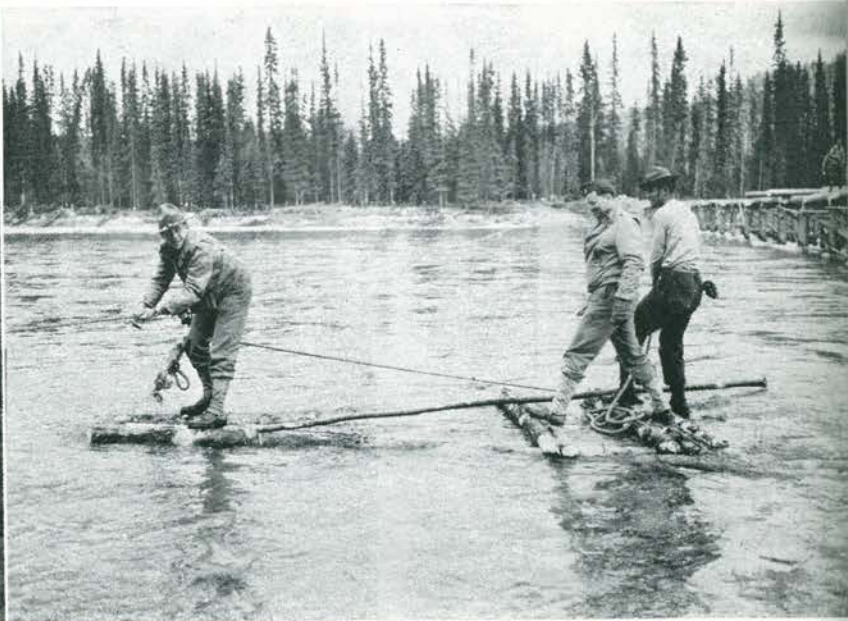
Another method of moving. Lts. Hilgendorf and Maxwell cross the Hyland river, mile 211, on a trail ferry powered only by the swift current.
