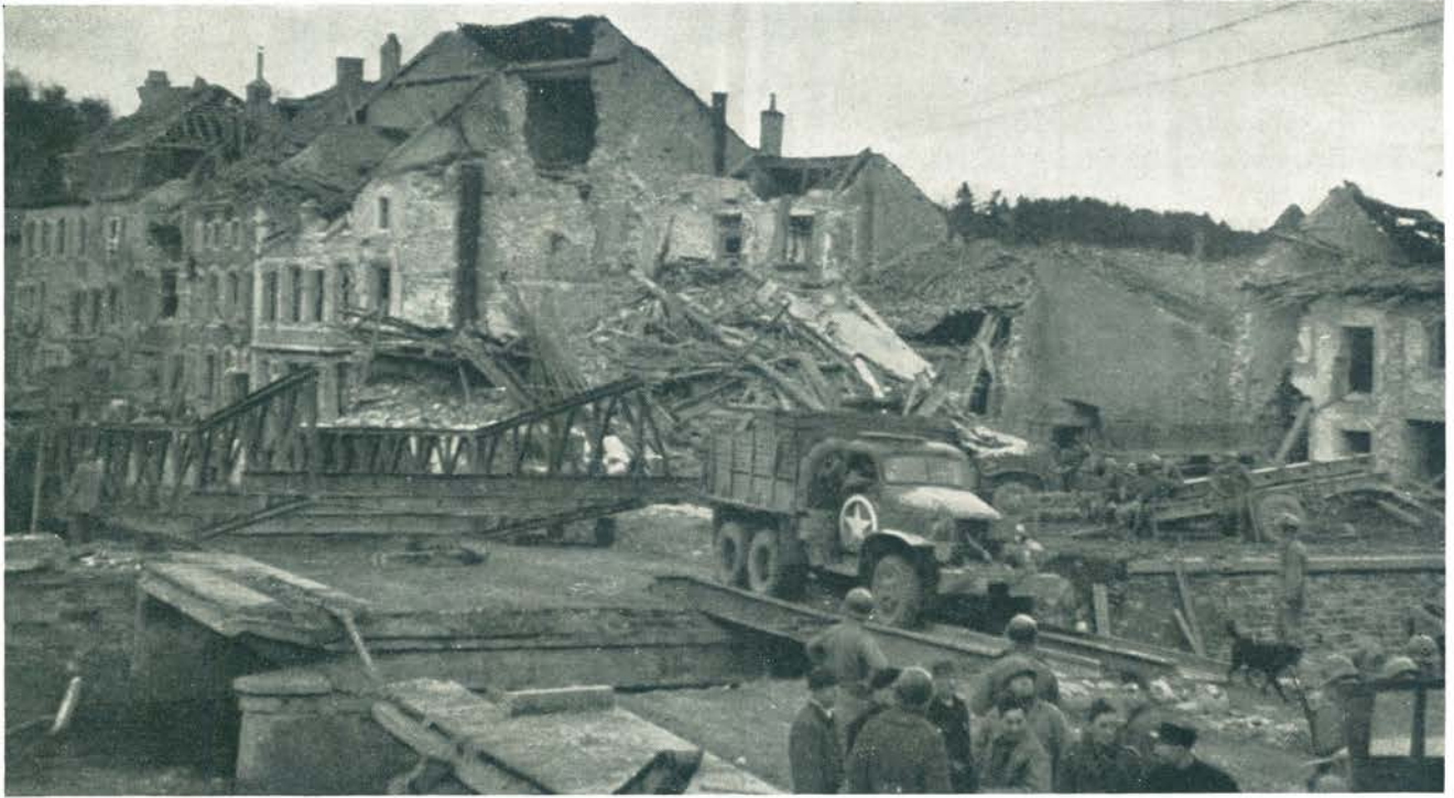
Blamont fell, and the road to the Alsace Plain was clear. France, November 20, 1944
