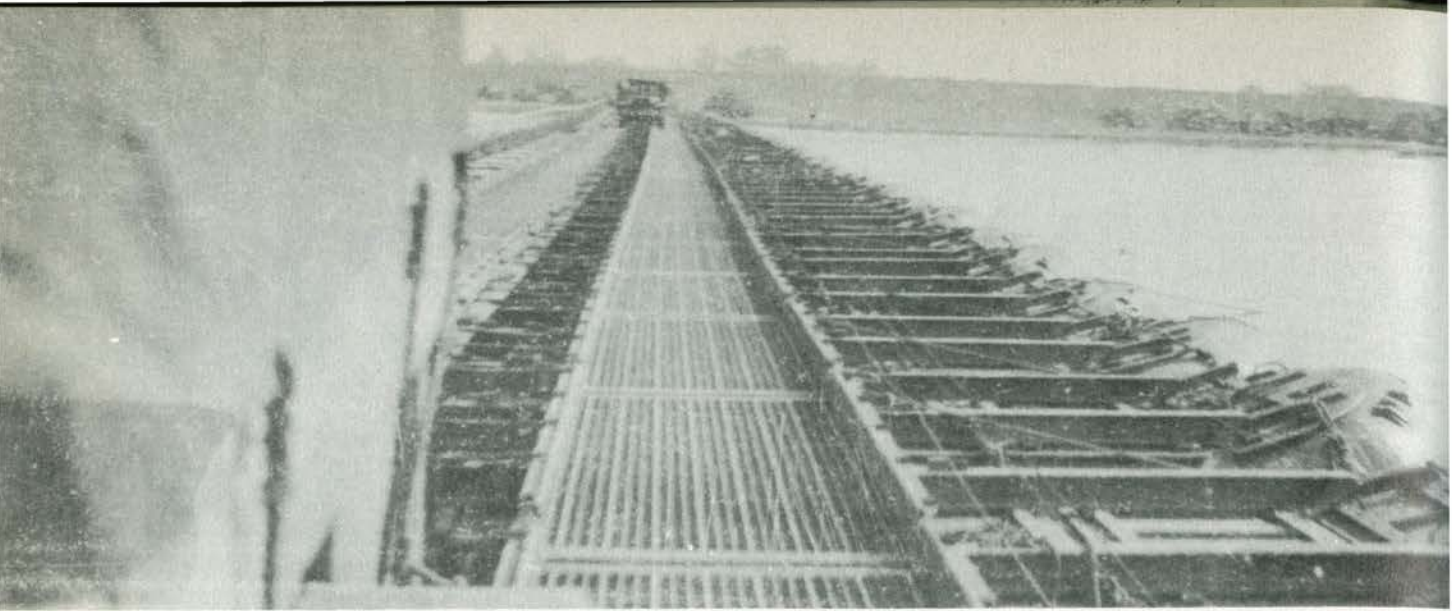
The Elbe Bridge
