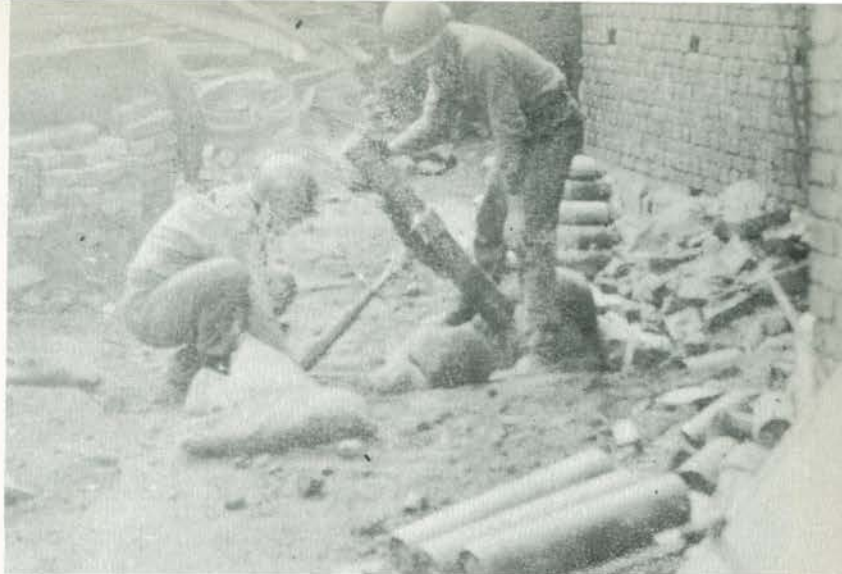
Laying 'em in
