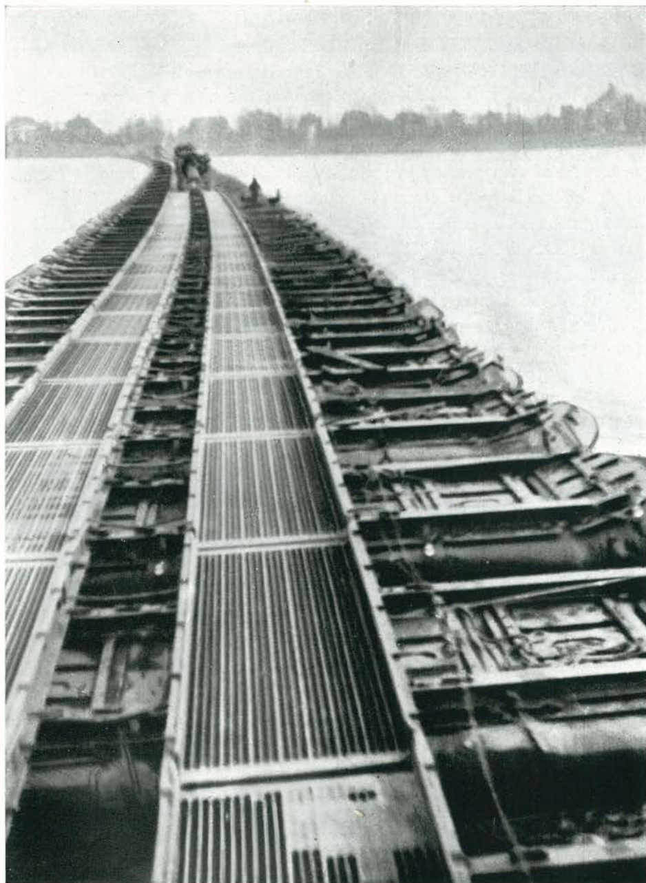
RHINE BRIDGE World's longest tactical span at Mainz.
