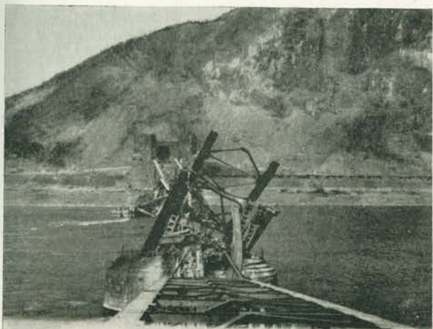
AND LATER — This is the same bridge after incessant shelling caused it to topple into the Rhine.
