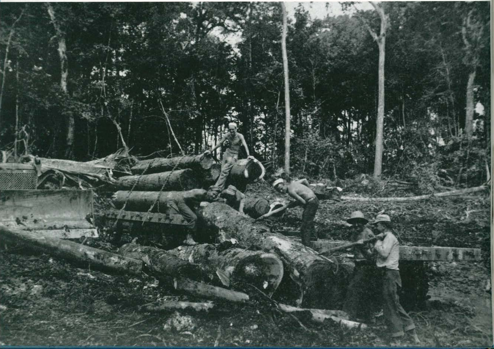
TAXIWAYS HAD TO BE FINISHED WITHOUT DELAY. HARDWOODS TEAKWOOD, MAHOGANY, AND EBONY TREES LEFT DEEP ROOTS EMBEDDED INTO THE CORAL. . . . SEABEES APPLIED THE BULLDOZER, LOGGING CREW, AND DYNAMITE AND SOON HAD THE JOB ON THE WAY
