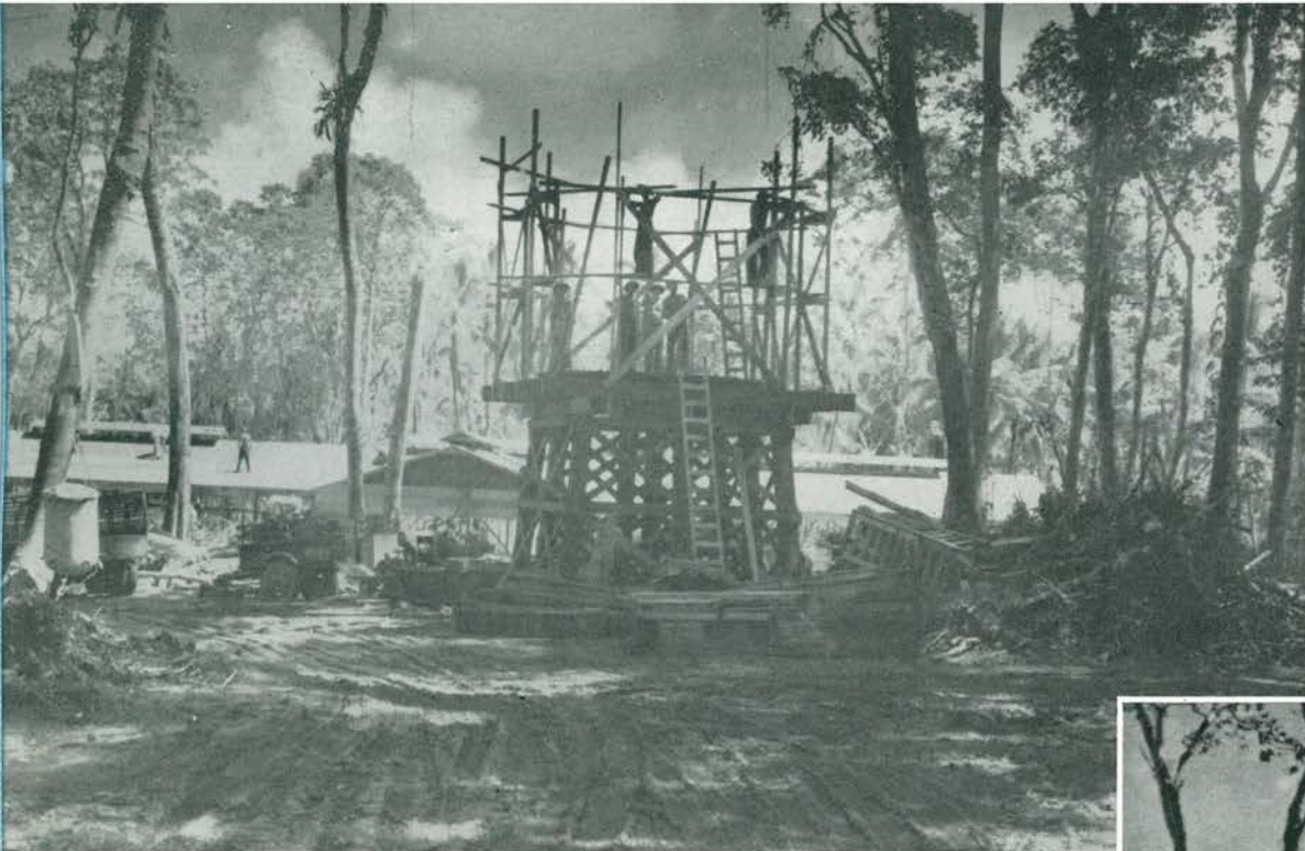
CONSTRUCTION OF WOODEN WATER TANK
