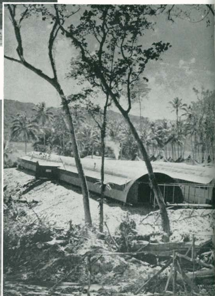
WE CONSTRUCTED FLEET
