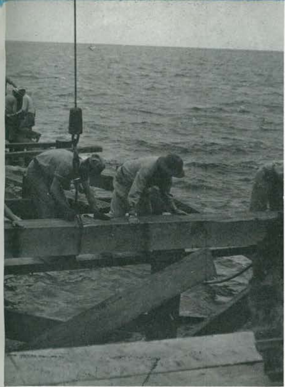
CRANE IS USED TO HOIST BEAM.
