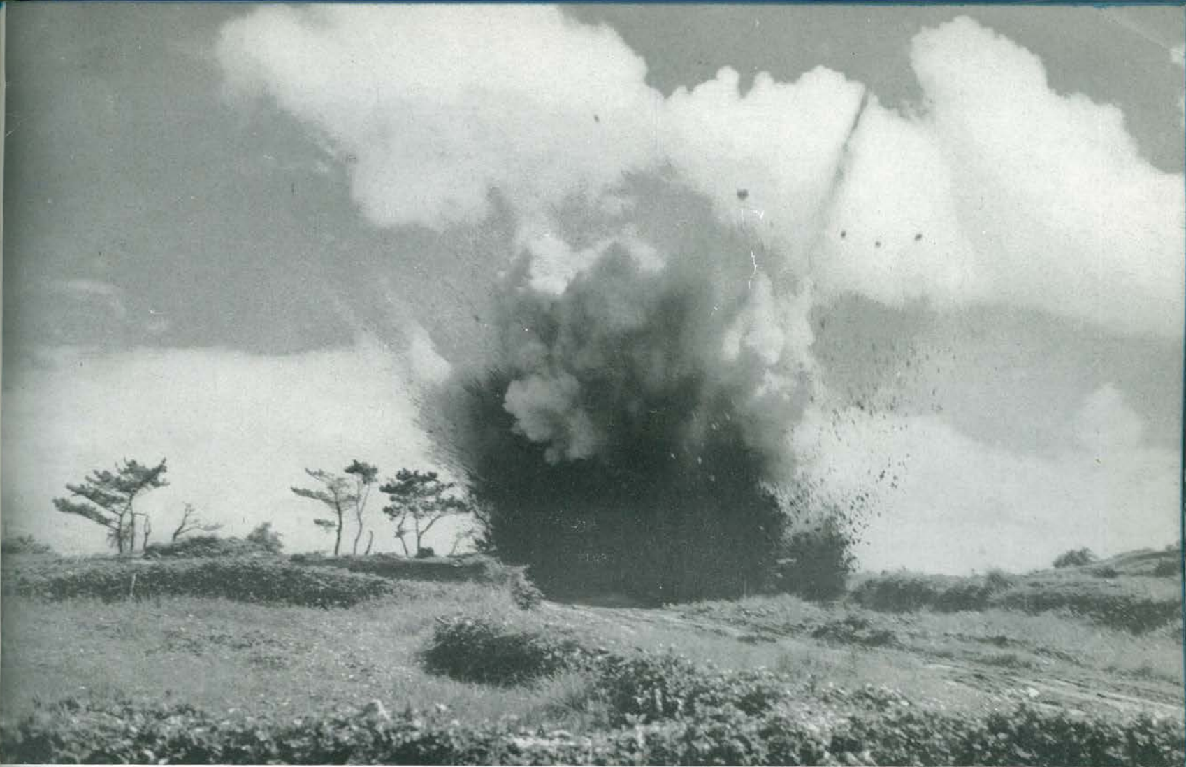
TONS OF DYNAMITE ARE USED IN BUILDING AN AIRFIELD. THE DYNAMITE CREW CONSISTS OF ALERT, TOUGH AND SPECIAL TRAINED MEN.
