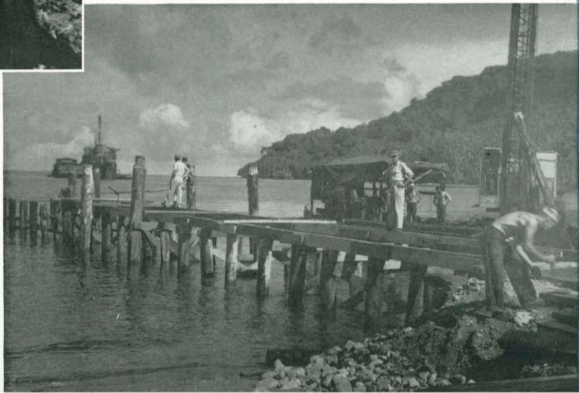
PIER CONSTRUCTION, MONO ISLAND
