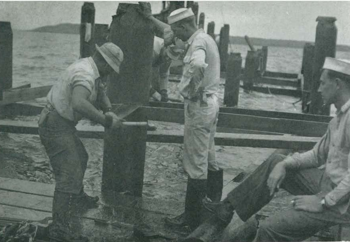
PILES RECEIVE FINISHING TOUCHES
