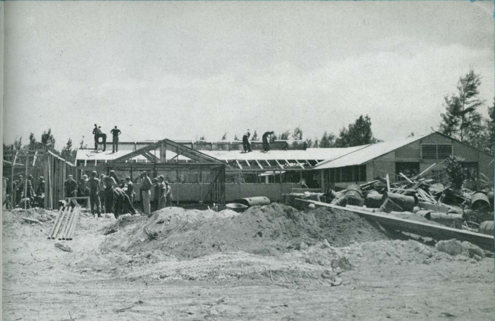
CONSTRUCTION AND MORE CONSTRUCTION. THE DITCHER WAS EMPLOYED BUT WITH LITTLE SUCCESS, BECAUSE THE SOIL WAS OF A SANDY NATURE.
