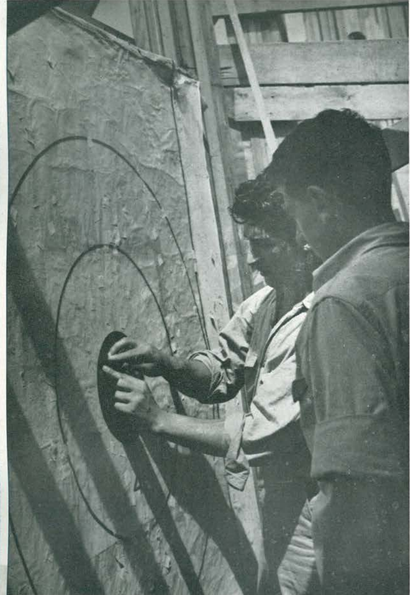
SEABEES REPAIR TARGET AT THE 82ND. RIFLE RANGE.
