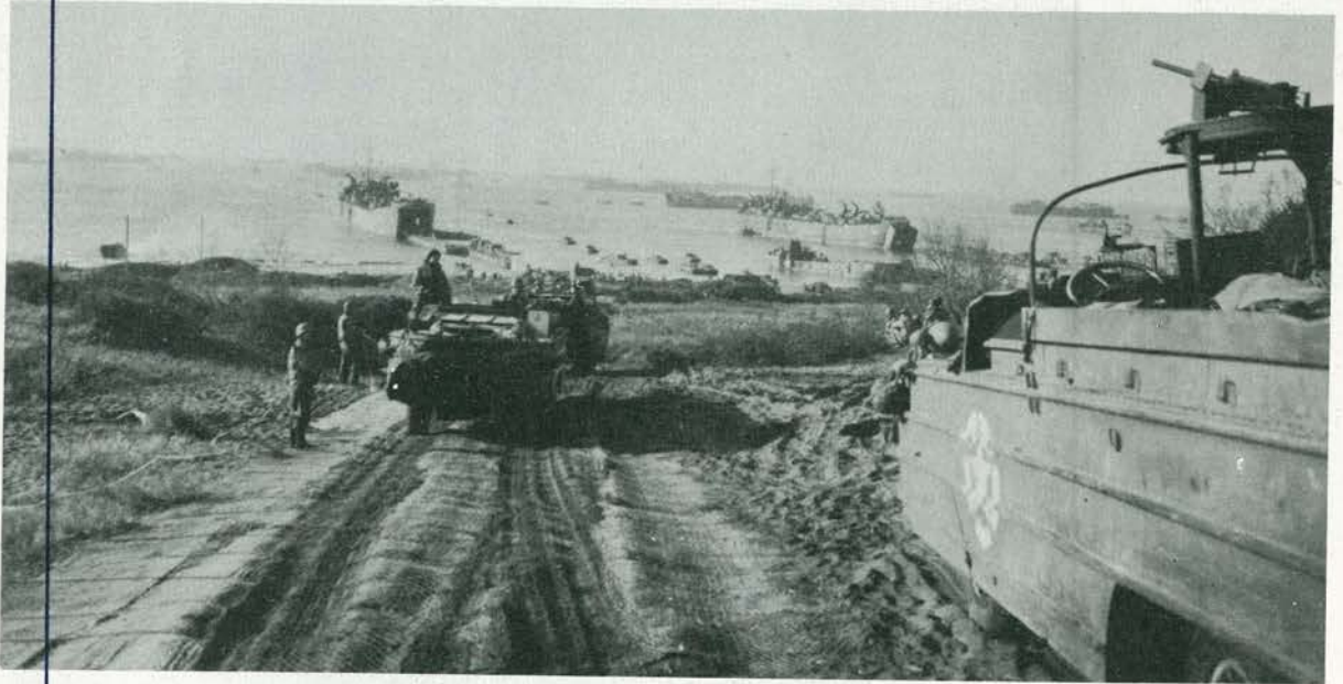
MEN AND EQUIPMENT COMING ASHORE AT ANZIO
