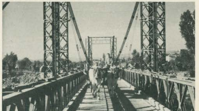
Near Florence: Experimental Suspension Bailey
