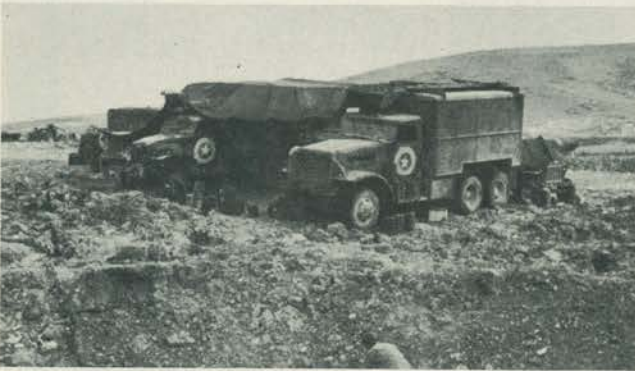
Staging Area No. 1, Bizerte: A Shell Hole
