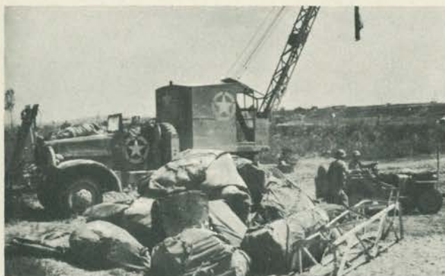
San Benedetto: First Step in Bridge Building
