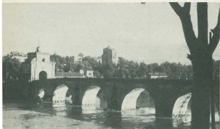
Pons Milvius: Rebuilt B. C. 109
