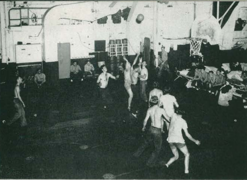
Hangar Deck Hoop Harange.
