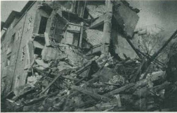
Typical of bomb damage in Cologne
