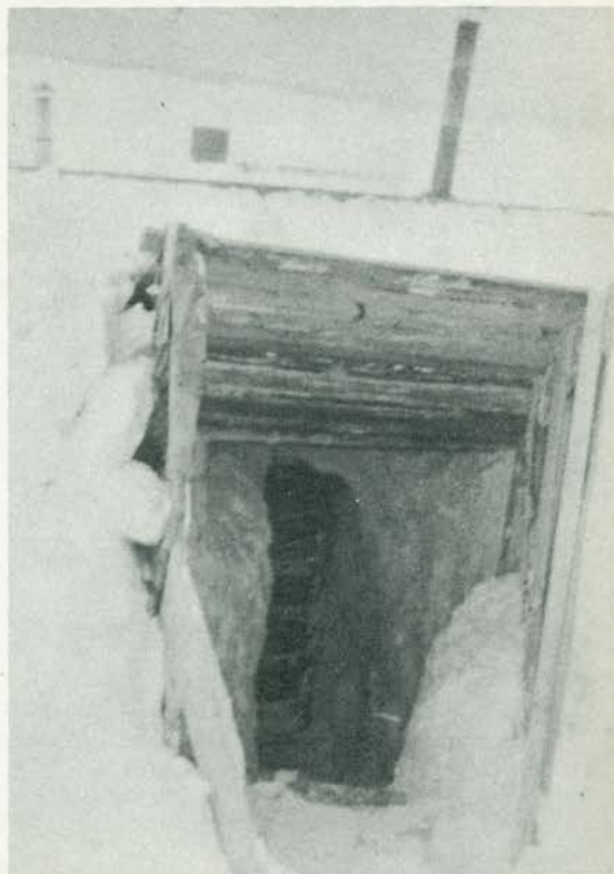
Adak. Storm entrance to living quarters
