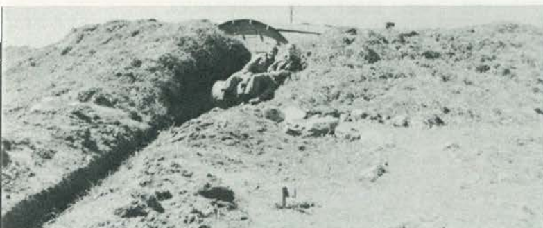
1st Sec. Quonset hut. Dug down five feet, and four feet of spoil. S/Sgt. Timmons, Cpl. Doose
