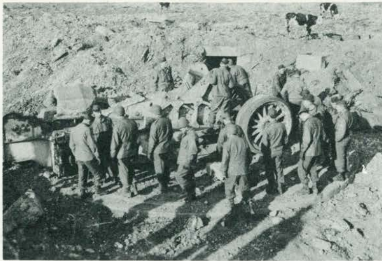
German constructed defenses about two miles back from the coast near Dieppe. Four of these guns were dug in below the surface and tunnels joined them. Guns were spaced 75 to 100 yards. Each gun was blown up at the breech by retreating Germans.
