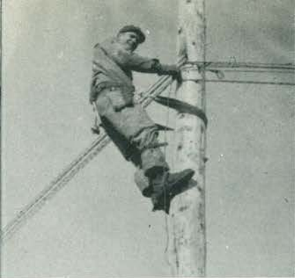
Pfc. Ramer "stringing" wire on Adak
