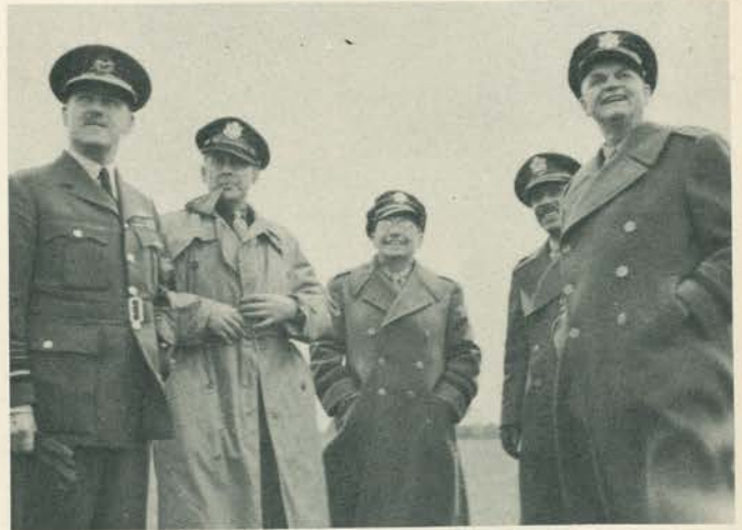
The High Command was happy over preparation progress. Sir Stafford Leigh-Mallory, Col. Wm. Whitacre, Lt. Gen. Louis Brereton, Brig. Gen. Beach, Maj. Gen. Paul Williams
