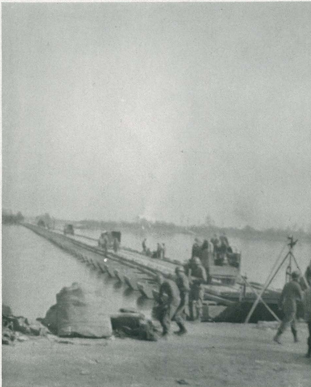
A completed pontoon bridge in operation. The vehicles maintain distance to prevent undue strain on any one section of the bridge.
