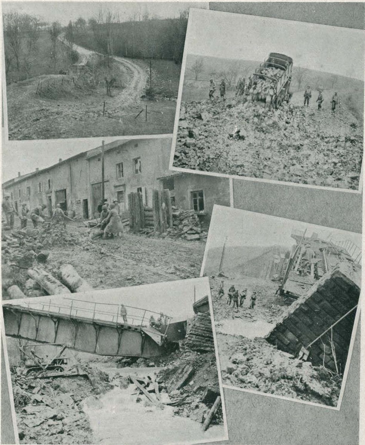
Twisted bridges and hasty enemy road blocks occupy the engineer's time.
