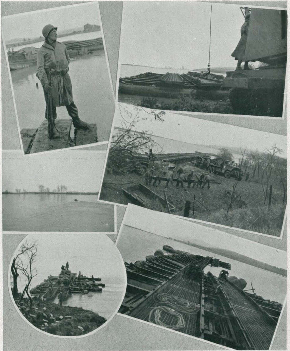
Water is an obstacle easily overcome by the modernized pontoon bridge.
