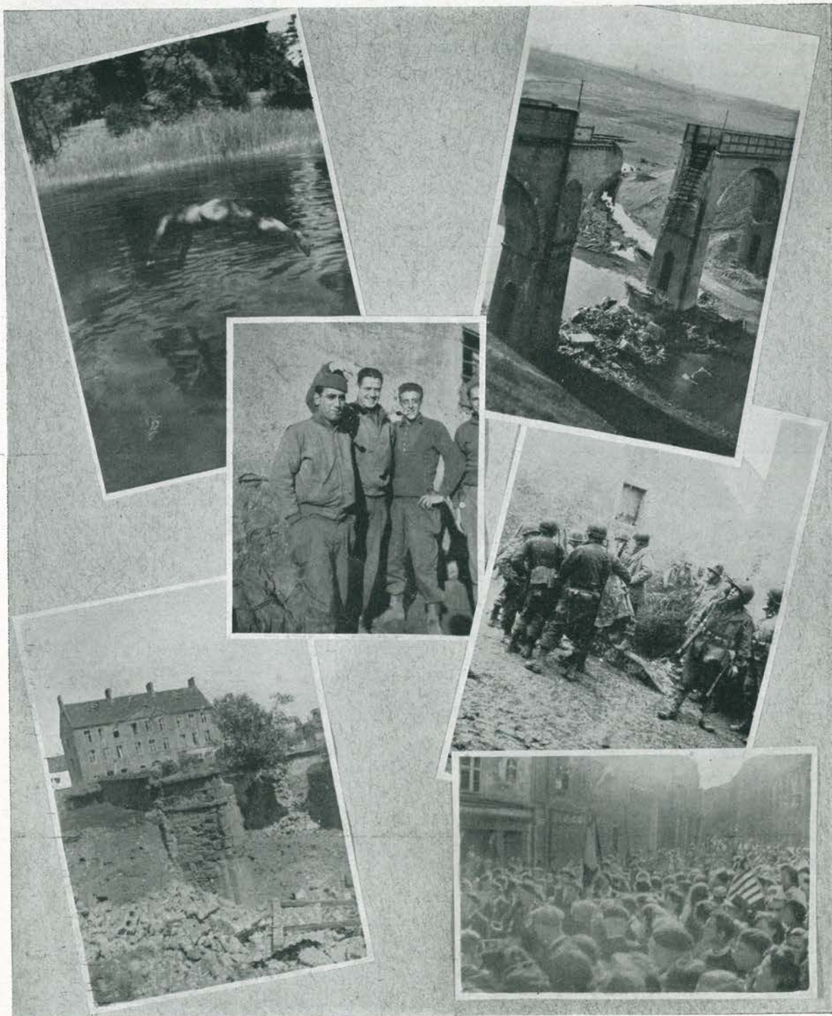
Blown bridges are encountered at Abouè in our advance toward Metz.
