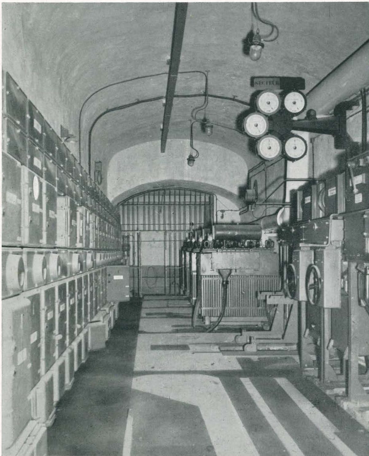
A power plant in the Maginot Line. Systems like this kept living conditions in the fortifications pleasant, with air conditioning, electric kitchens and moving pictures.
