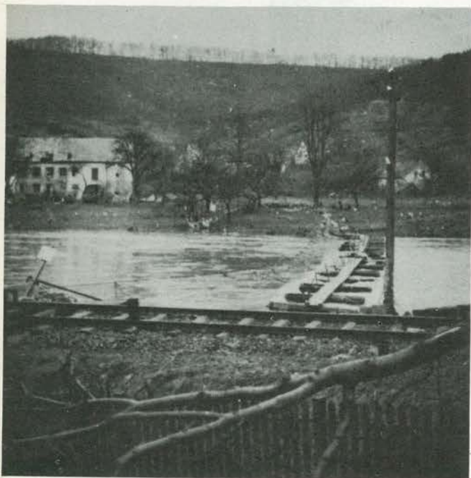
Sauer River Footbridge
