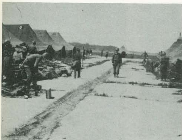
Supply on street
