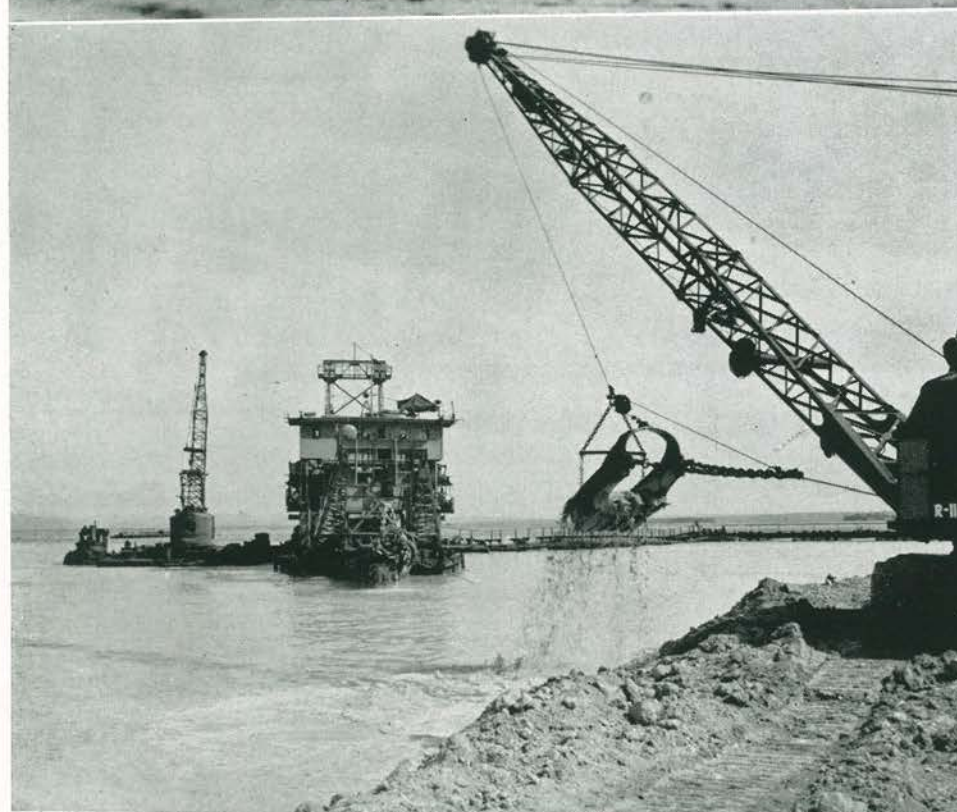
SUCTION DREDGE IN OPERATION
