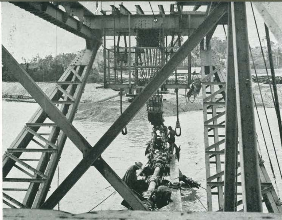
DREDGE SUCTION AND CUTTER HEAD
