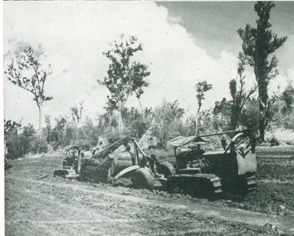
D-8 WITH SCRAPER GRADING COMPOSITE
