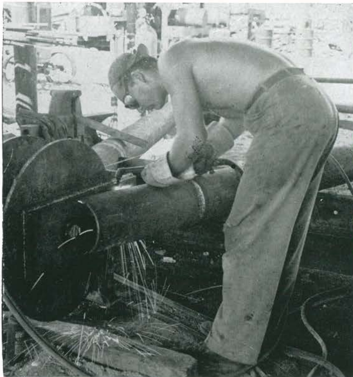
WELDER WORKING ON BARGE FRAME
