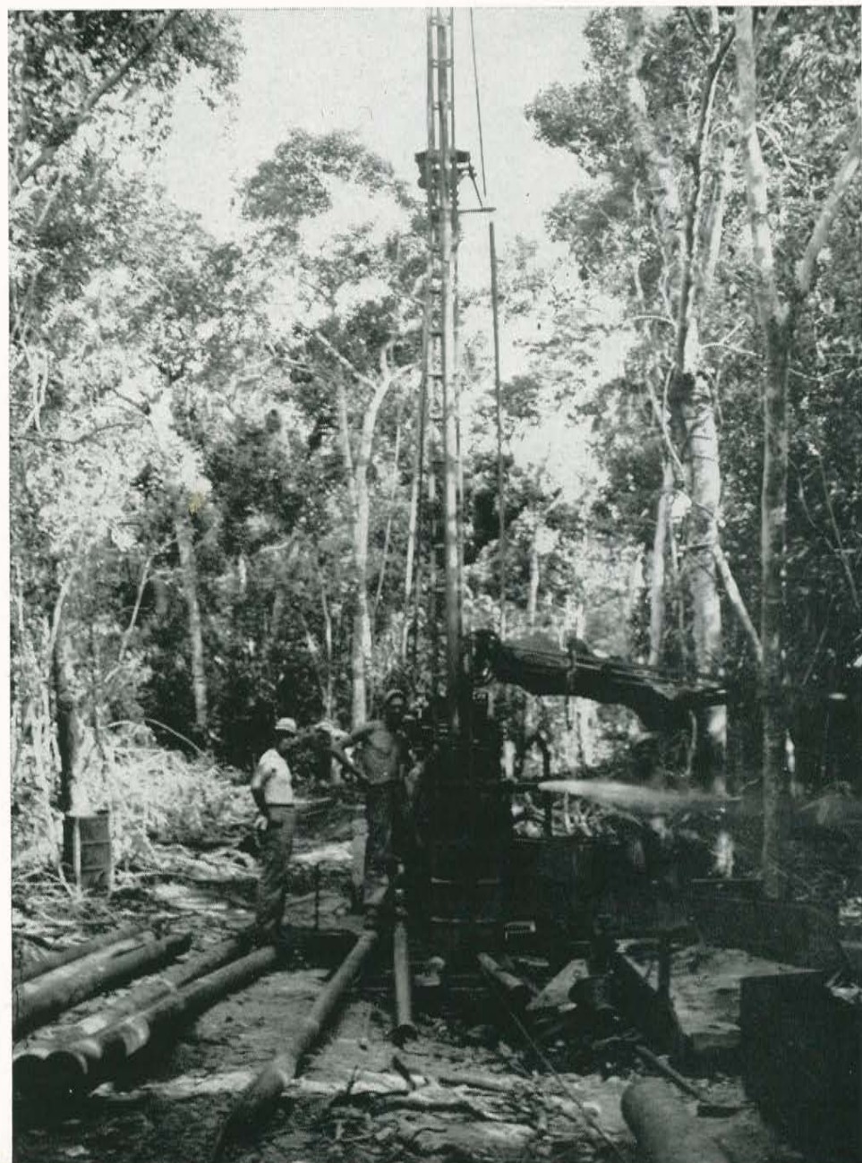
DRILLING A WATER WELL
