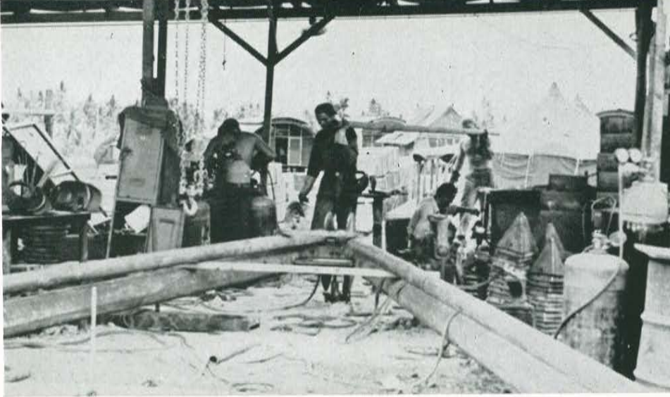
WELDING SHOP FABRICATING BARGE 'A' FRAME
