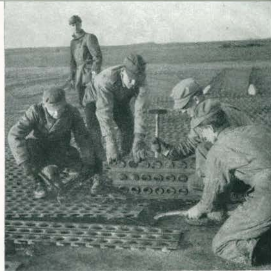
Laying pierced plank for the review at Honington.
