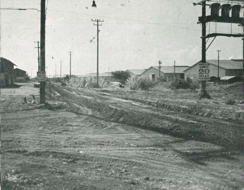
Paving laid by 90th men in the CHA 1-3 Naval Housing areas added a pleasing modern village appearance. Here reside hundreds of civilian workers employed at the nearby Pearl Harbor Navy Yard. In addition to the paving, the 90th Seabees did the highway culvert job shown in
