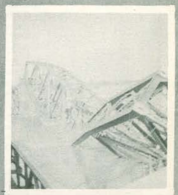
DEMOLISHED BRIDGE ACROSS RHINE RIVER—MAINZ, GERMANY
