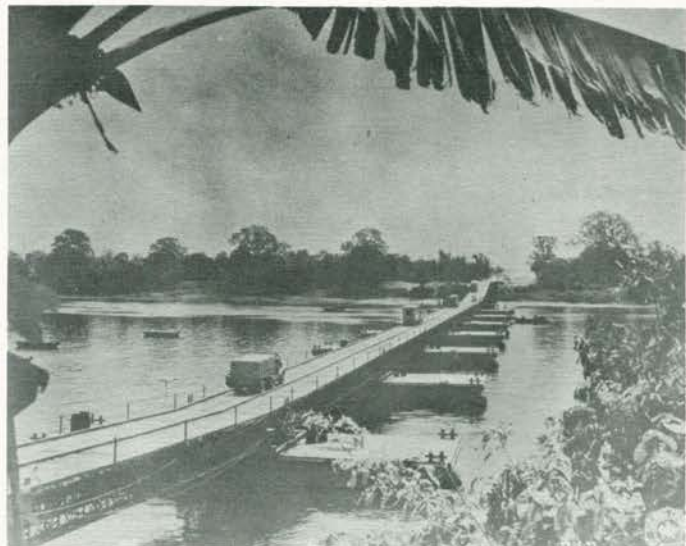
Vehicles of China-bound convoy No. 114 drive over the 110-ton barge bridge across the Irrawaddy River at Myitkyina, Burma
