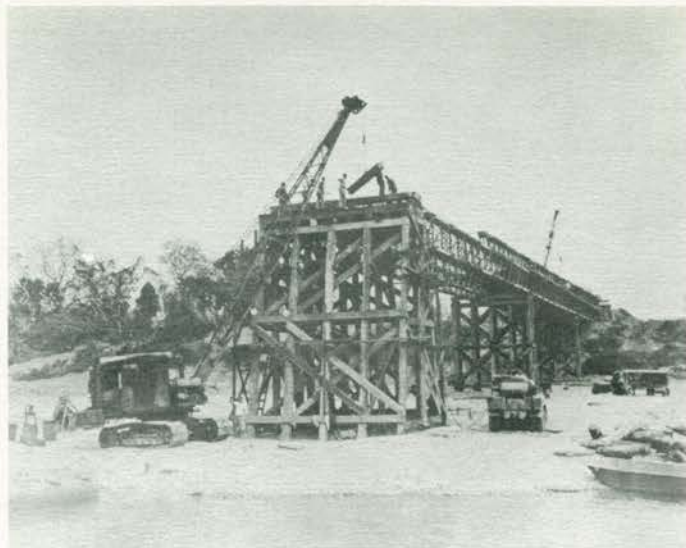
Lorain crane lowering cap on trestle bent of H-20 floating bridge over which Ledo Road will cross Irrawaddy River, Burma.
