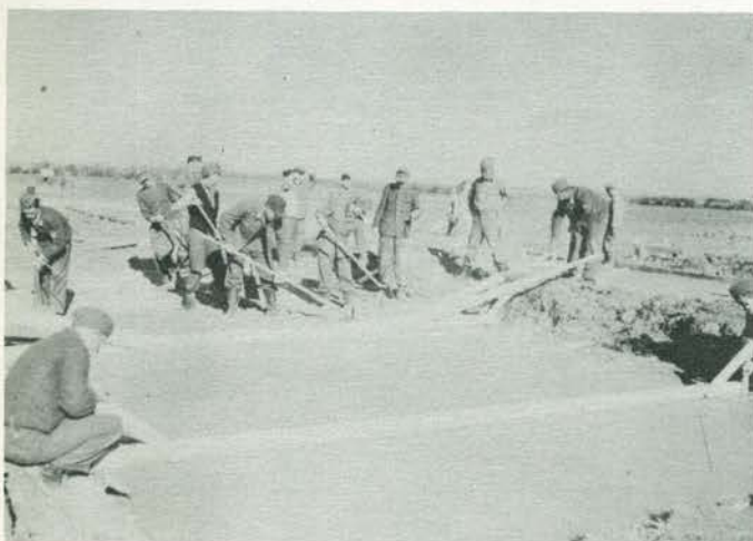
Laying concrete floors — POW workers
