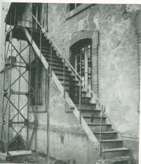
Fire escape construction — Le Mans
