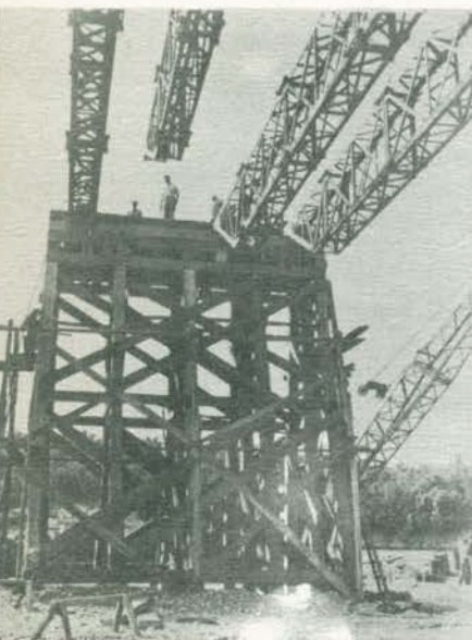
Launching nose of 4th H-20 section almost in place on cap of 3rd trestle bent of Ledo Road bridge across the river.
