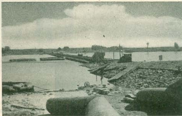
"By noon of April the 14th, NINTH Army Engineers had completed this treadway bridge."
